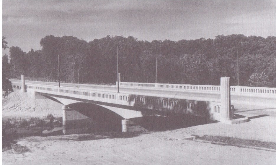
Figure 3.10: Delaware's version of Bomber Plant Bridge, erected 1951
