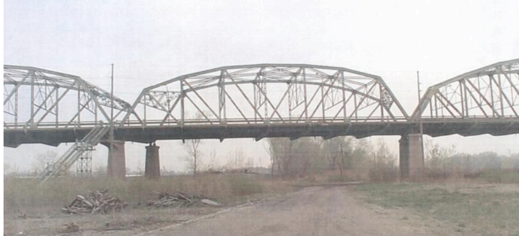
Figure 7.2: Parker through truss, erected 1935, available through Indiana's Historic Bridge Marketing Program
