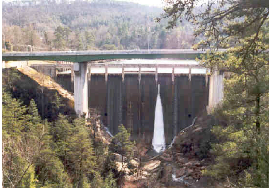
Figure 4.6: Tallulah Falls Bridge after deck replacement
