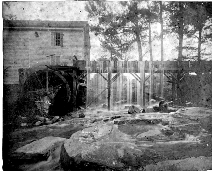
Figure 6.3: Grist Mill at Big Sandy Creek
