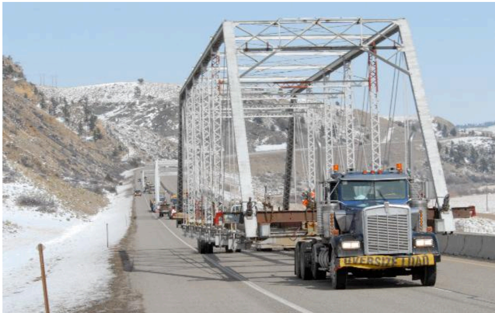
Figure 1.9: Craig Bridge during its relocation to Ten Mile Creek at the State Nursery in 2006
