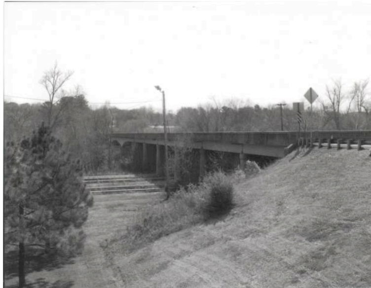
Figure 5.5: Bomber Plant Bridge
