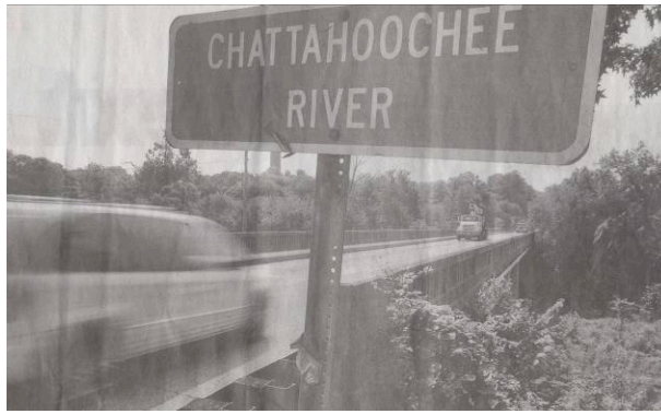
Figure 5.4: Bomber Plant Bridge meets controversy in 2007
