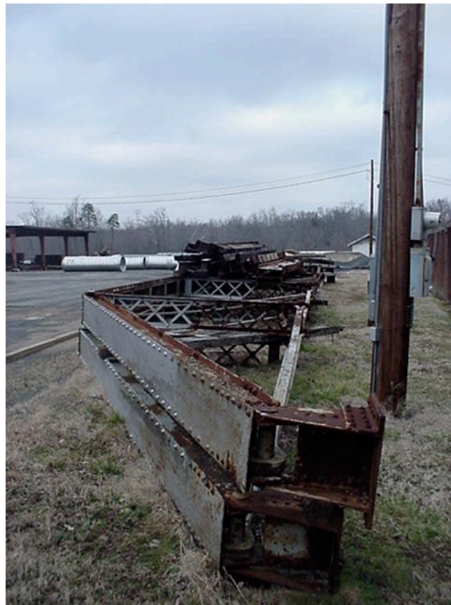
Figure 1.8: National Register-eligible 'pony truss' bridge, shown ready for relocation, currently listed as "recipient identified" by the NCDOT
