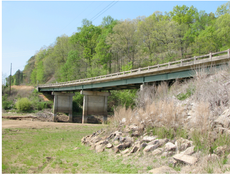
Figure 3.7: Lula Bridge over the Chattahoochee River
