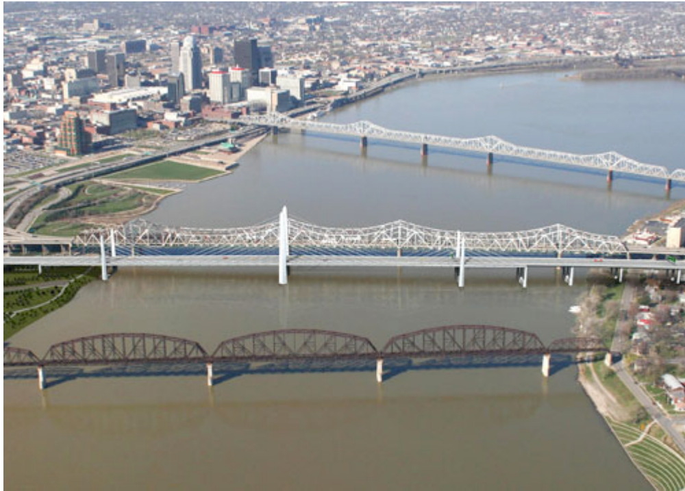
Figure 7.3: Three of the Ohio River bridges in the Kentucky-Indiana Project
