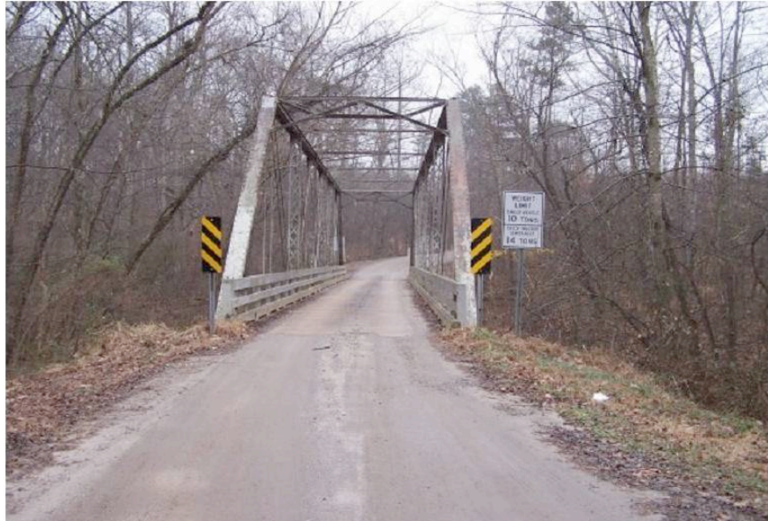
Figure 1.7: National Register-eligible 'Pratt through-truss' bridge (built 1910) currently listed as "under contract" by the NCDOT
