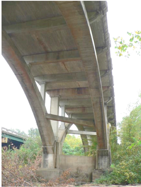
Figure 3.9: Substructure of the bridge carrying US Highway 78 (Westbound) above the Apalachee River
