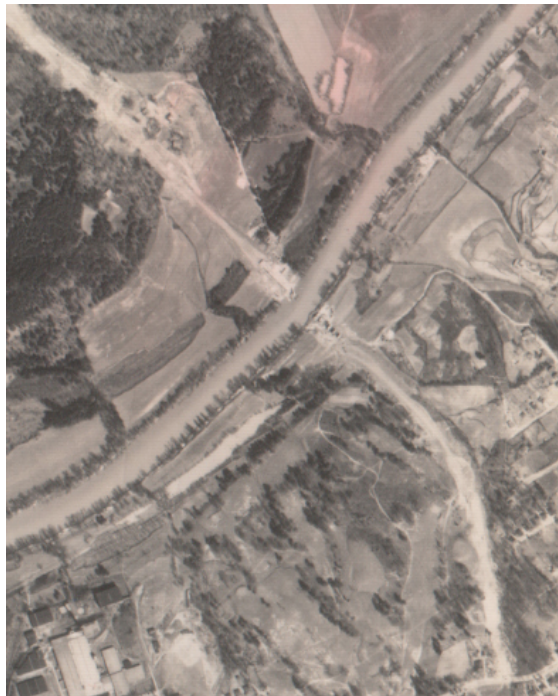
Figure 5.1: Aerial view of the construction process of Bomber Plant Bridge
