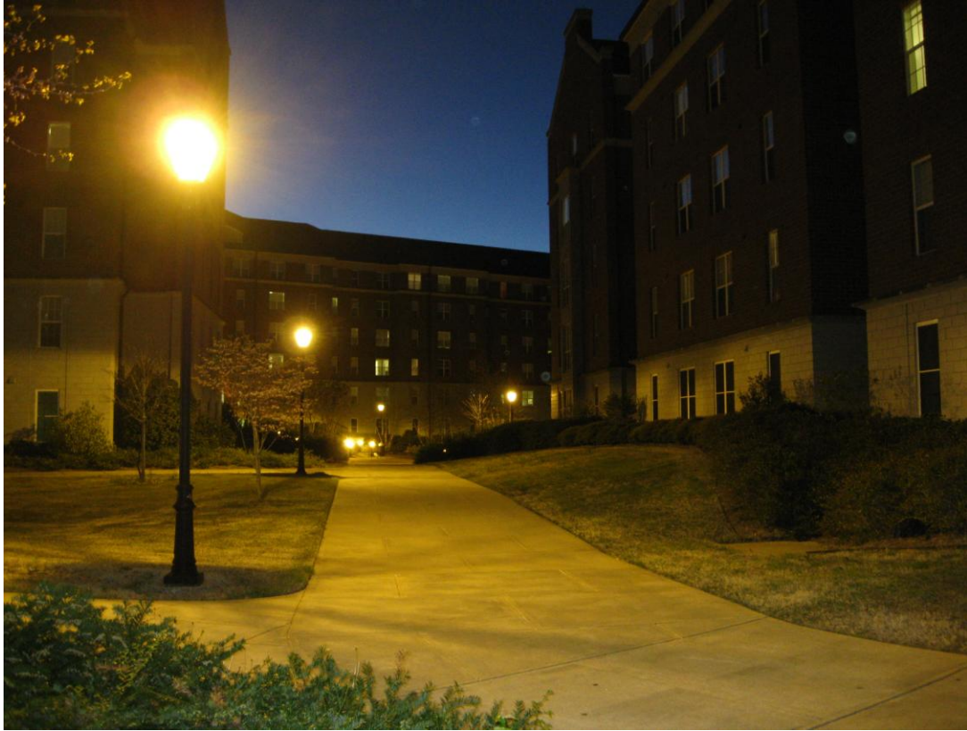
Figure 5.19 Before view of existing lighting for area II
