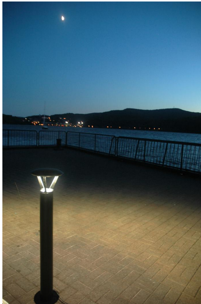
Figure 5.12 Selected full-cutoff bollard light
