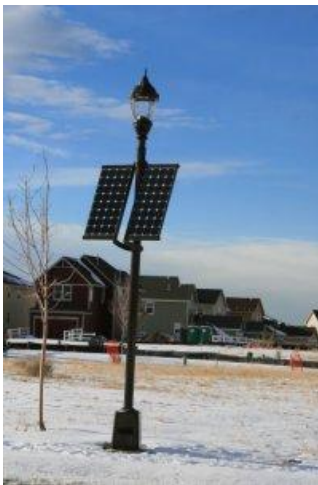
Figure 3.7 (Image to the left) Self-contained solar power system
