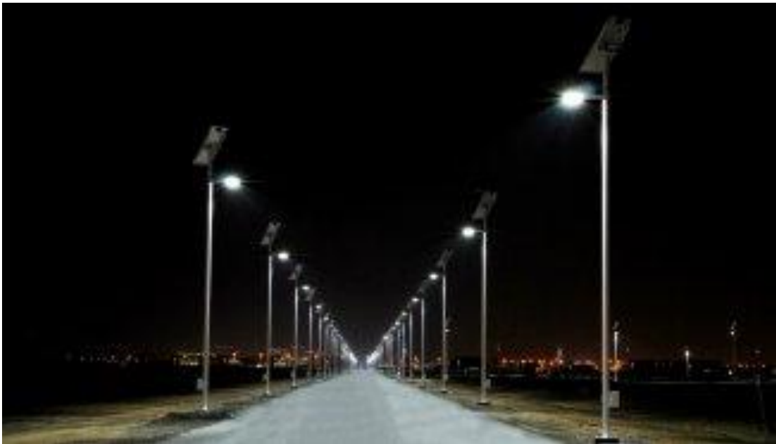
Figure 3.11 Solar roadway lights
