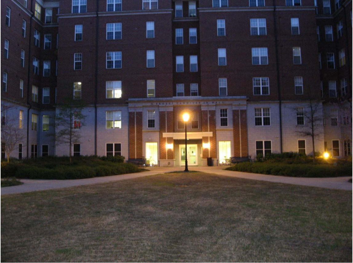
Figure 5.14 First before view of existing lighting for area I
