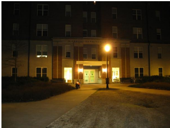
Figure 5.8 (Image on the right) Light installed in front of Vandiver Hall
