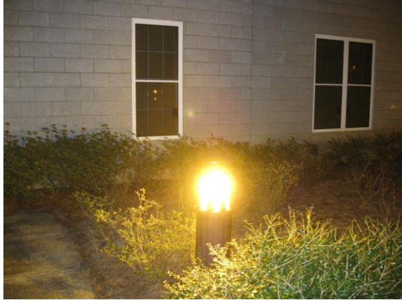
Figure 5.7 (Image on the left) Light trespass from existing bollard light
