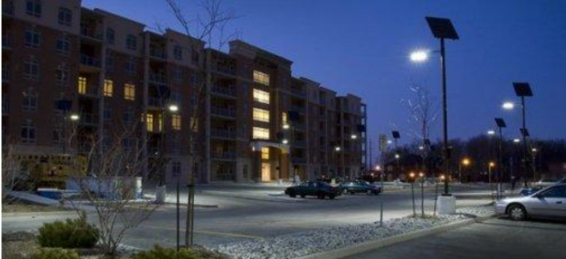
Figure 3.12 Solar parking lot lights
