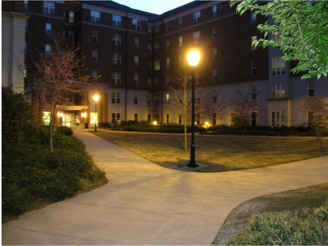
Figure 5.16 Second before view of existing lighting for area I
