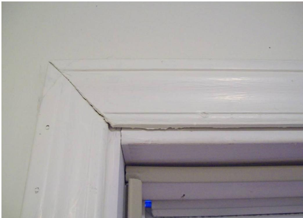
**Figure 73:** 105 Sammy's Road, Deteriorating Door Frame & Broken Seal, Clearview, Alleghany County, VA (Leonard, 2014)
