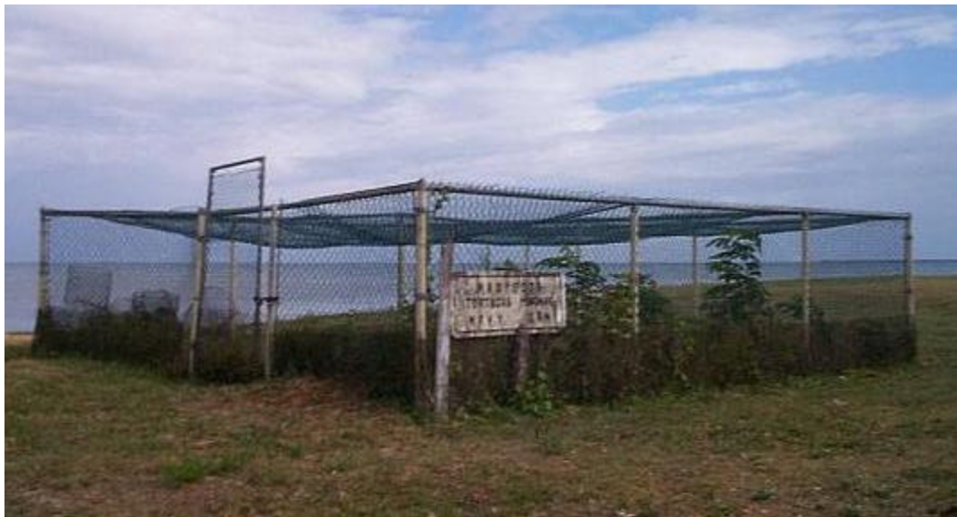
Figure 1.1: Enclosure to protect turtle eggs and baby turtles. This enclosure, built by the Navy, is on a beach in the NASD.
