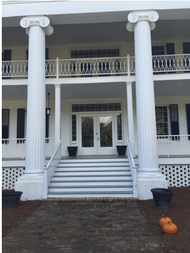
Figure 4 Greenwood Plantation door and surround; taken October 2015
