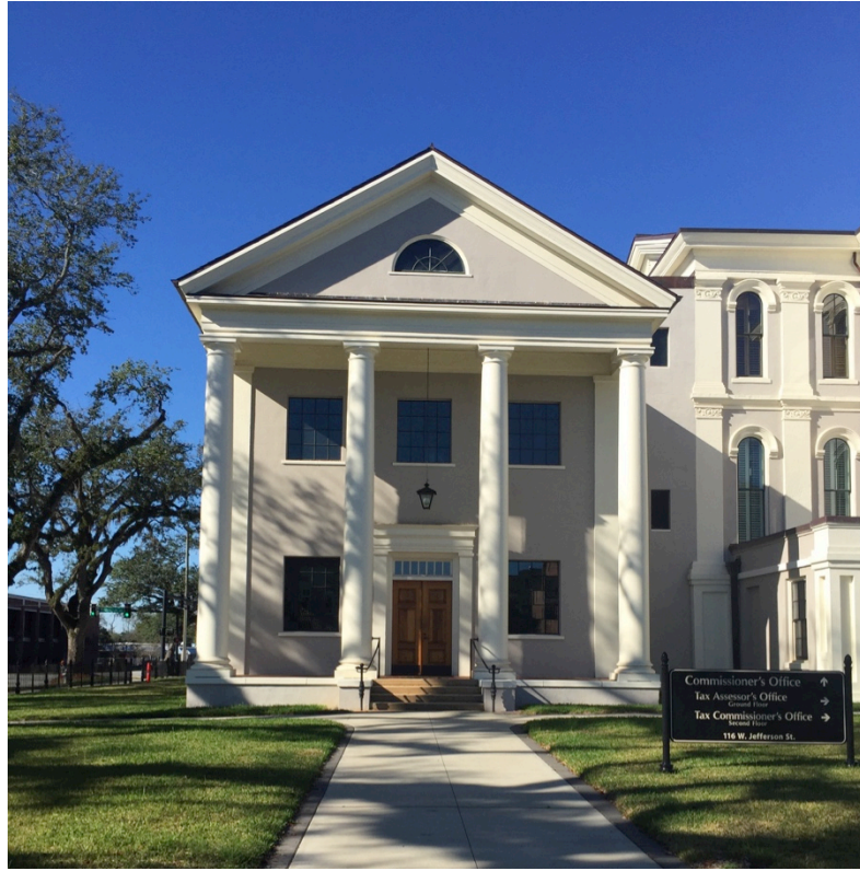
Figure 29 Thomas County Courthouse, annex; taken February 2016
