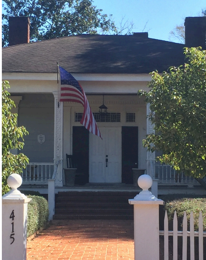
Figure 13 Wright House, door surround; taken February 2016
