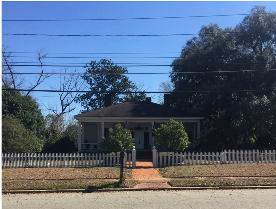
Figure 13 Wright House, front elevation; taken February 2016
