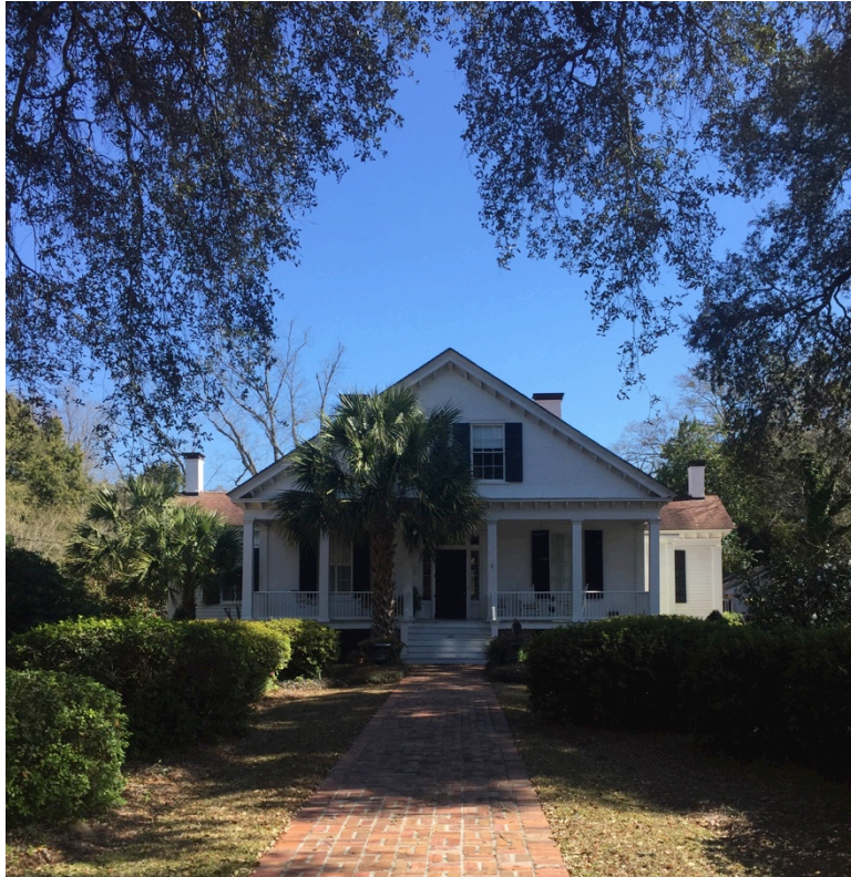
Figure 8 Hansell House, front elevation; taken February 2016
