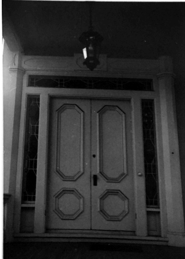
Figure 3 Hardaway House, door surround, date unknown; courtesy of Thomasville Landmarks, Inc.
