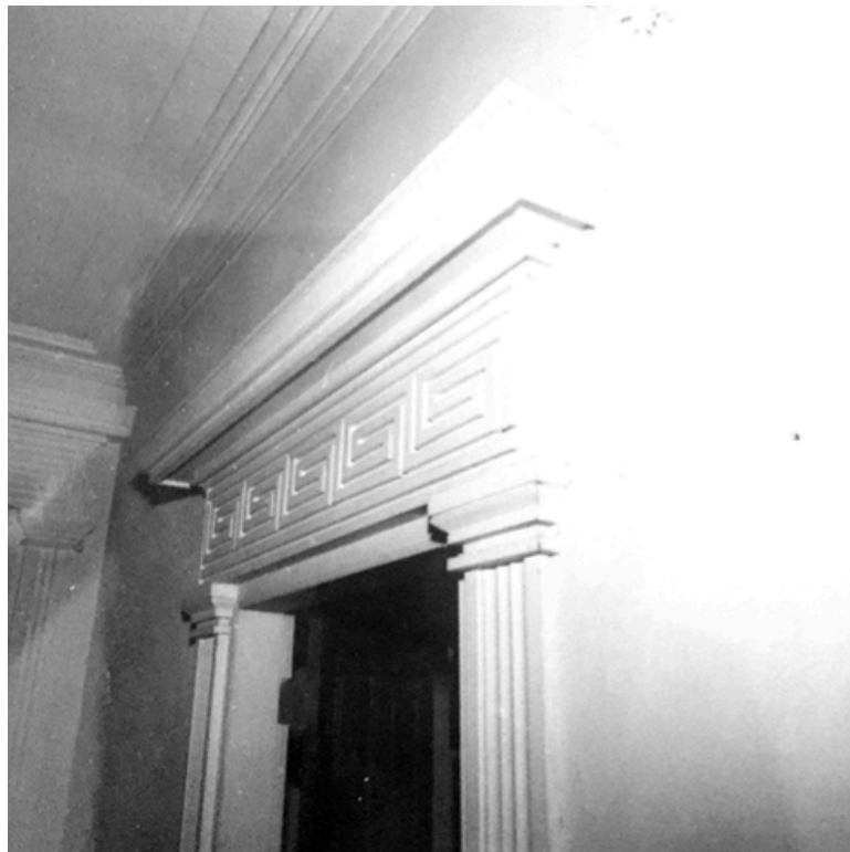
Figure 11 Hansell House, door head casing, date unknown; courtesy of Thomasville Landmarks, Inc.
