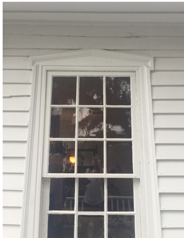
Figure 12 Susina Plantation, window head; taken December 2015
