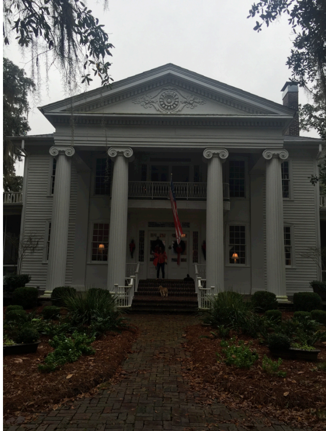
Figure 9 Susina Plantation, front elevation; taken December 2015
