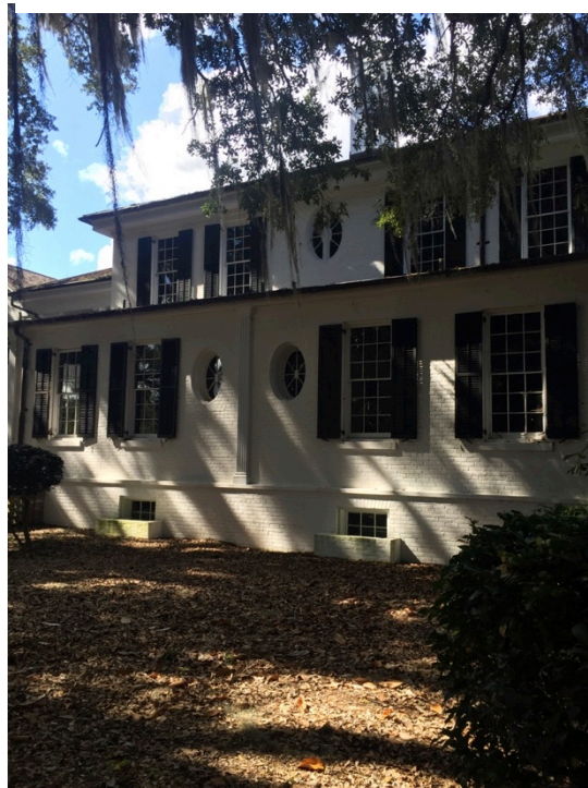
Figure 8 Greenwood Plantation, east elevation; taken October 2015
