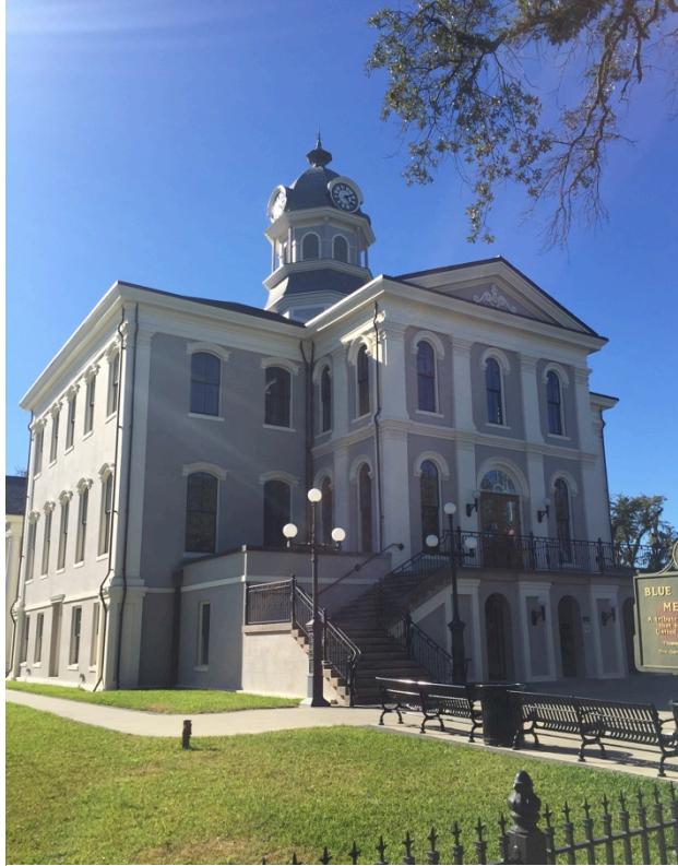
Figure 27 Thomas County Courthouse, front elevation; taken February 2016
