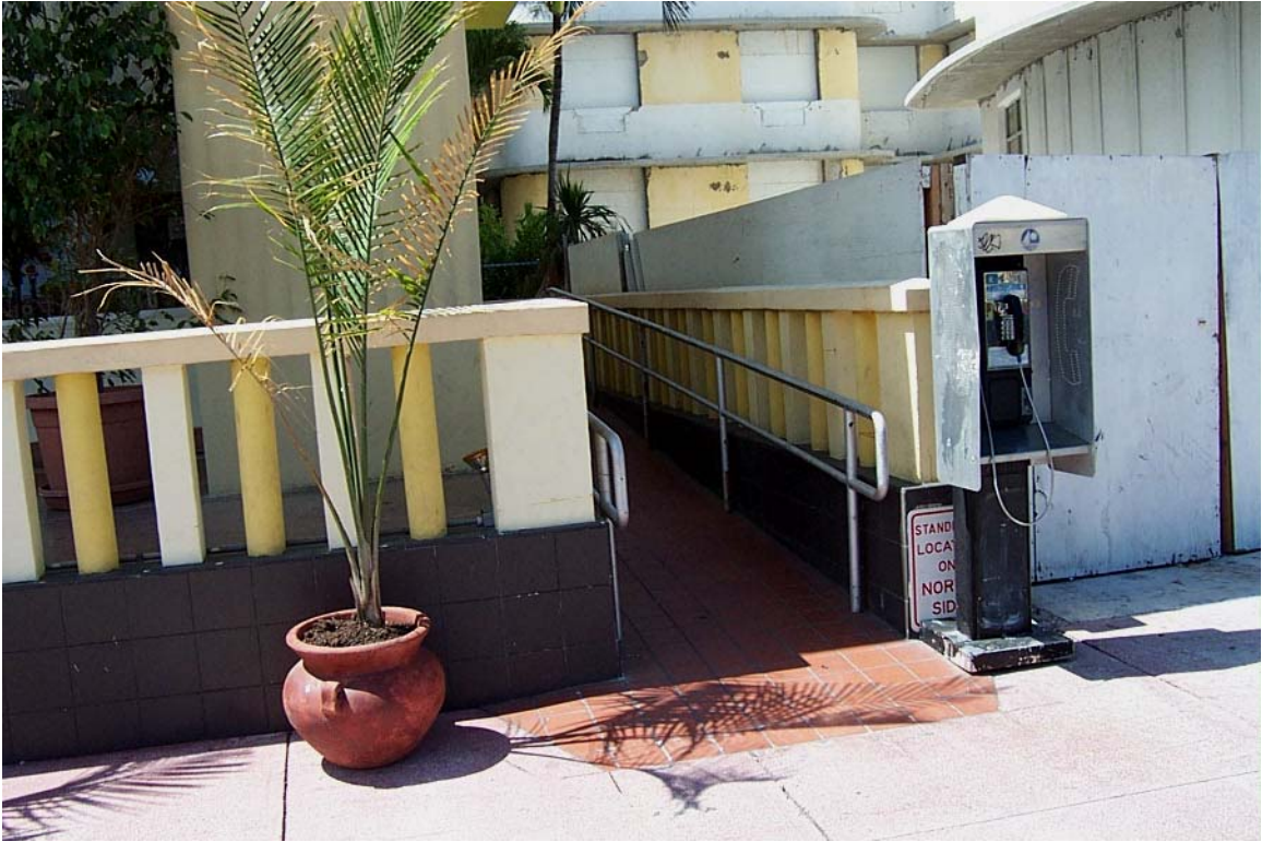
Photo 3: Close up of the ramp at the Leslie Hotel.
