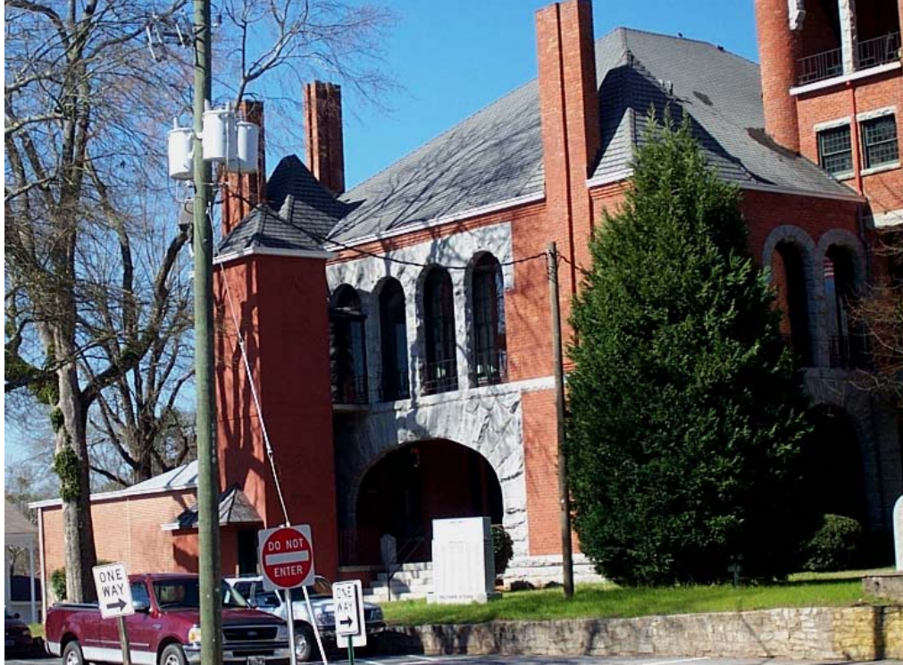
Photo 13: Close up of elevator tower.
