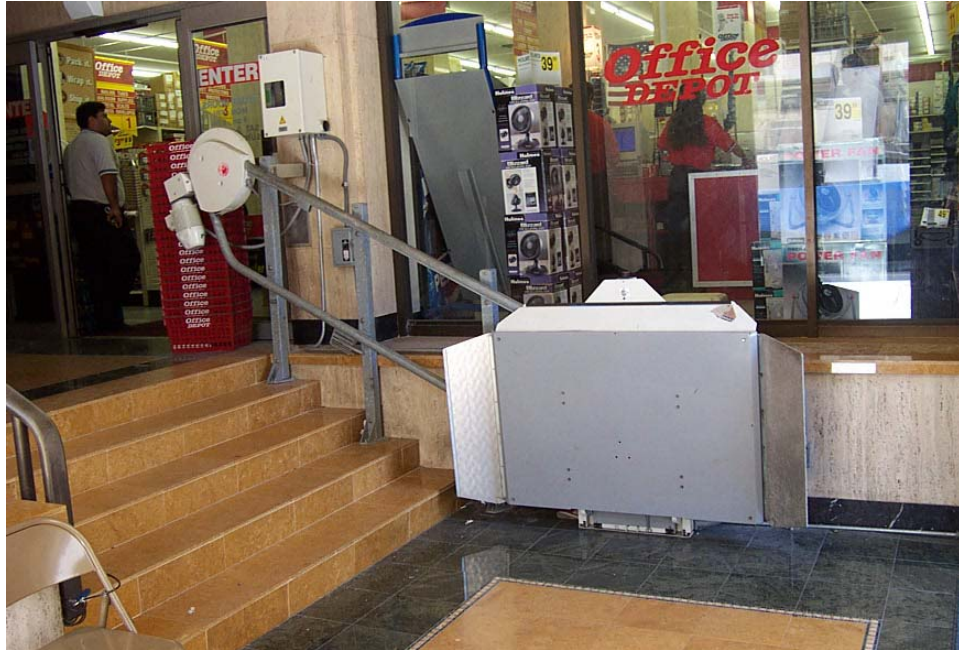
Photo 11: A side-view of the lift, while not in use.
