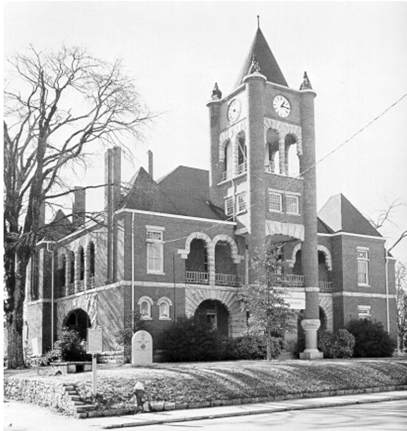
Photo 14: Oglethorpe County Courthouse prior to accessibility alterations (HABS photo, from The Georgia Catalog )
