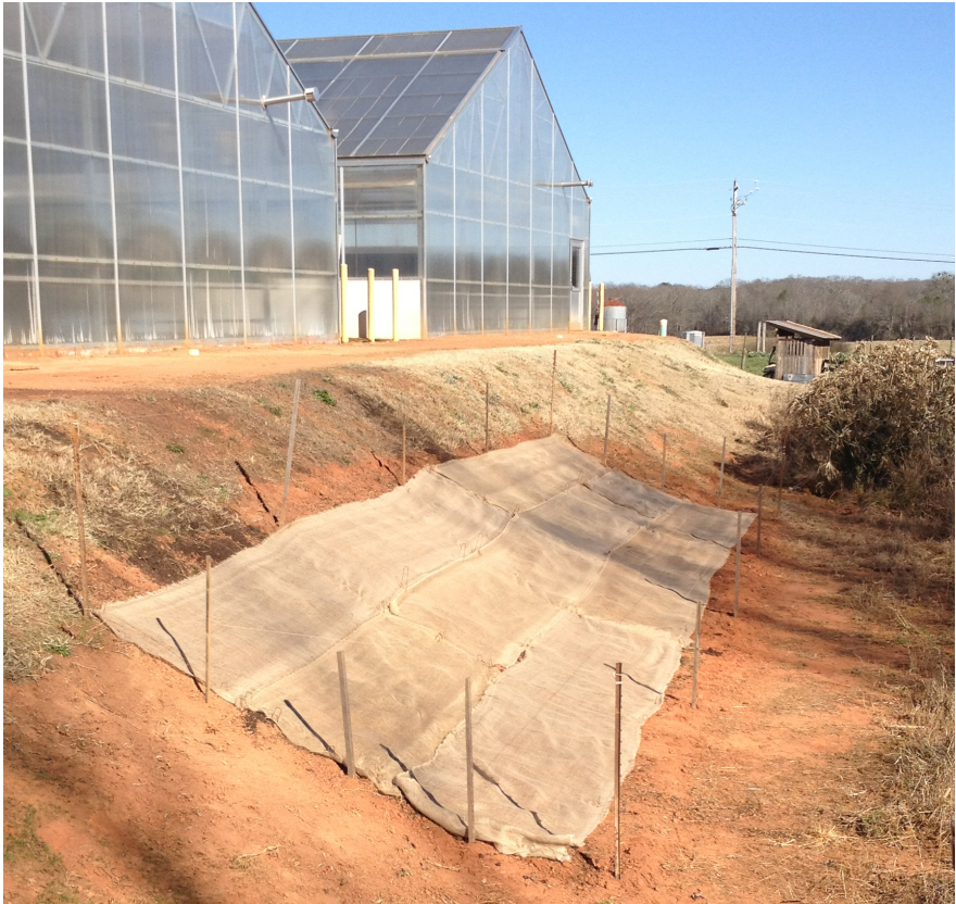
Figure 1-4. The tilled soil covered with Dewitt Natural Burlap set in place with landscape stakes. (photo credit: Jonathan Korman)
