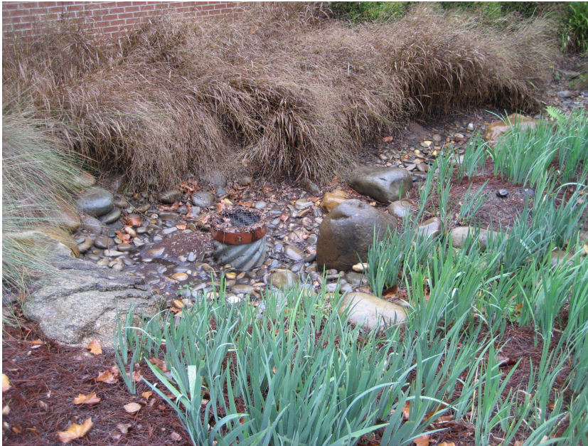
Figure 3-4. Overflow pipes control rain garden flooding. (photo credit: UGA, Office of Sustainability)
