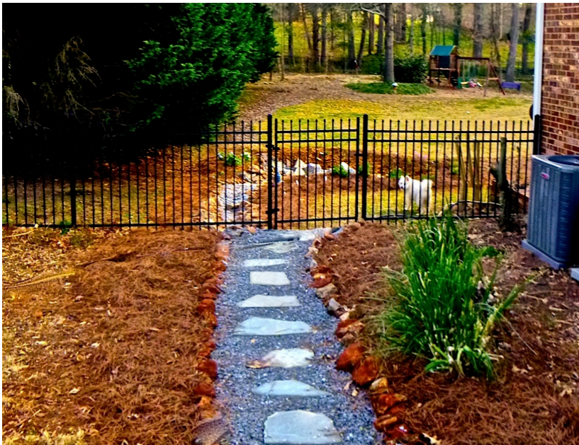
Figure 3-6. A French drain brings water to a residential rain garden in Watkinsville, GA (photo credit: Thomas Peters)
