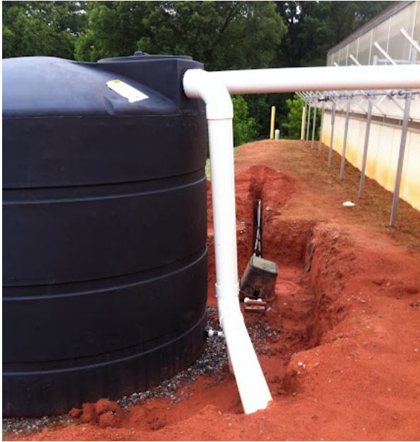
Figure 2-2. Large above ground cistern installation in Athens, GA. (photo credit: Frank Henning)
