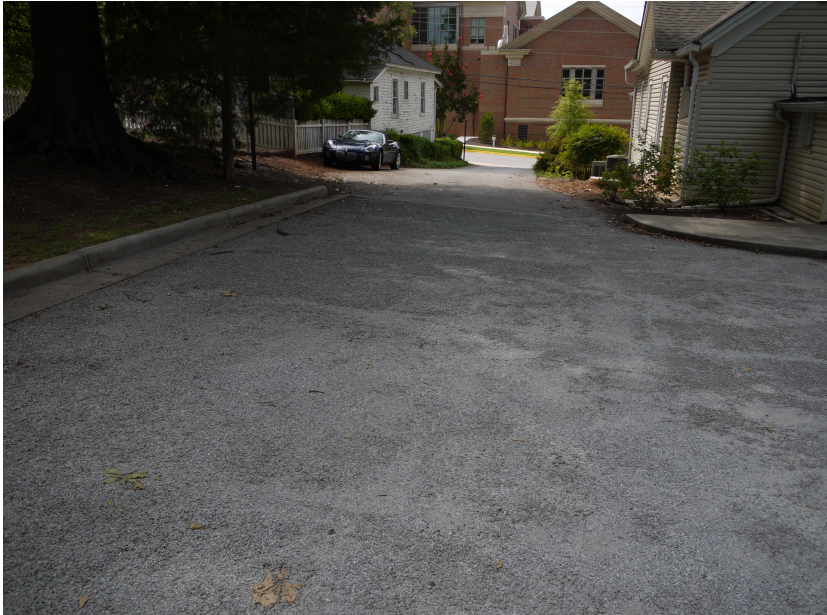
Figure 2-4. Porous pavement installation in Athens, GA. (photo credit: Jonathan Korman)
