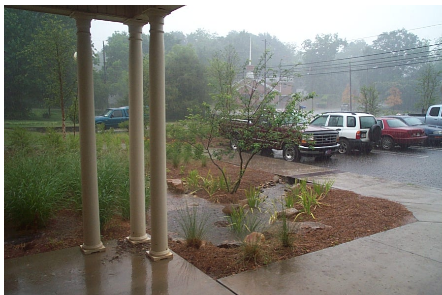
Figure 3-5. Rain garden parking lot flow. (photo credit: UGA, Office of Sustainability)
