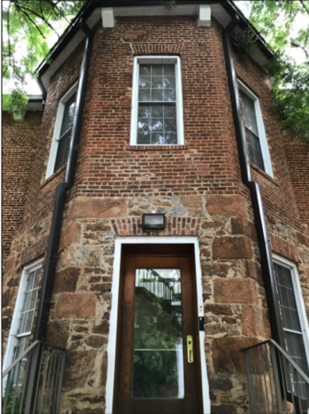
Figure 58, Central Tower of the main Cook and Brother Armory façade.
