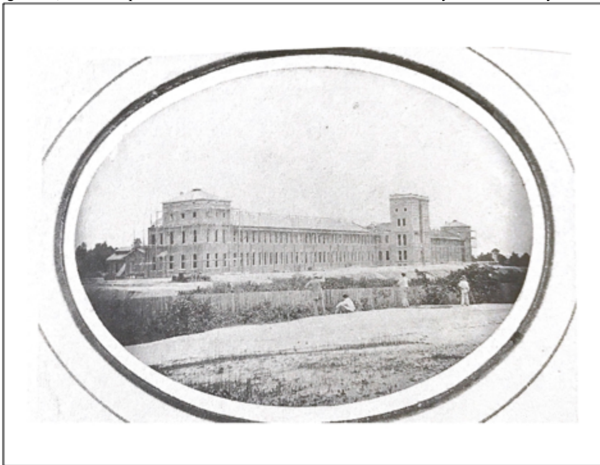
Figure 16, Construction at Confederate States Armory in Macon, Georgia.
