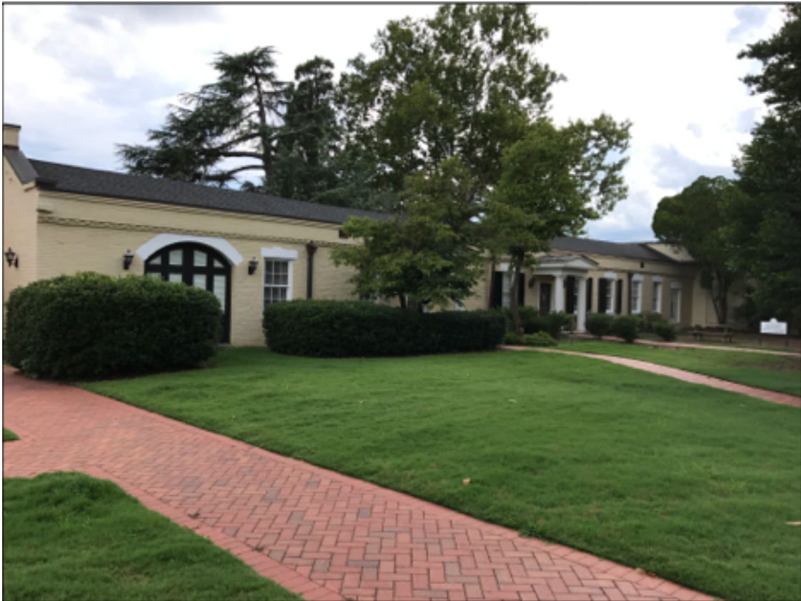
Figure 44, Augusta Arsenal Kitchen and Mess Hall now Quad Wall Building.
