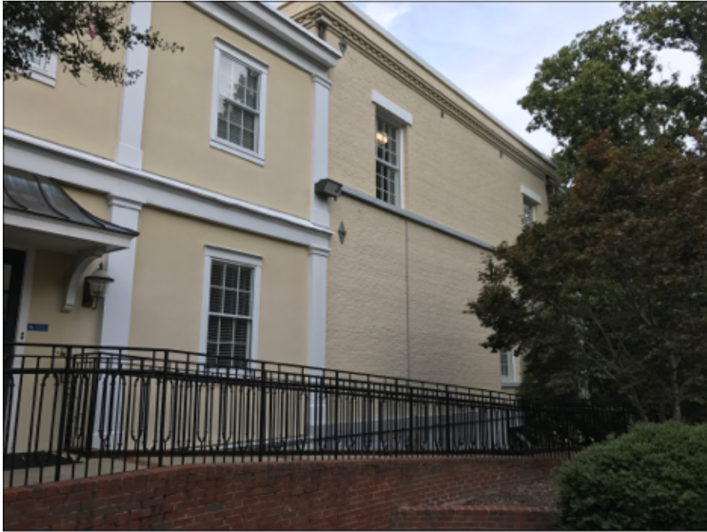
Figure 35, Southern façade and addition of Rains Hall.
