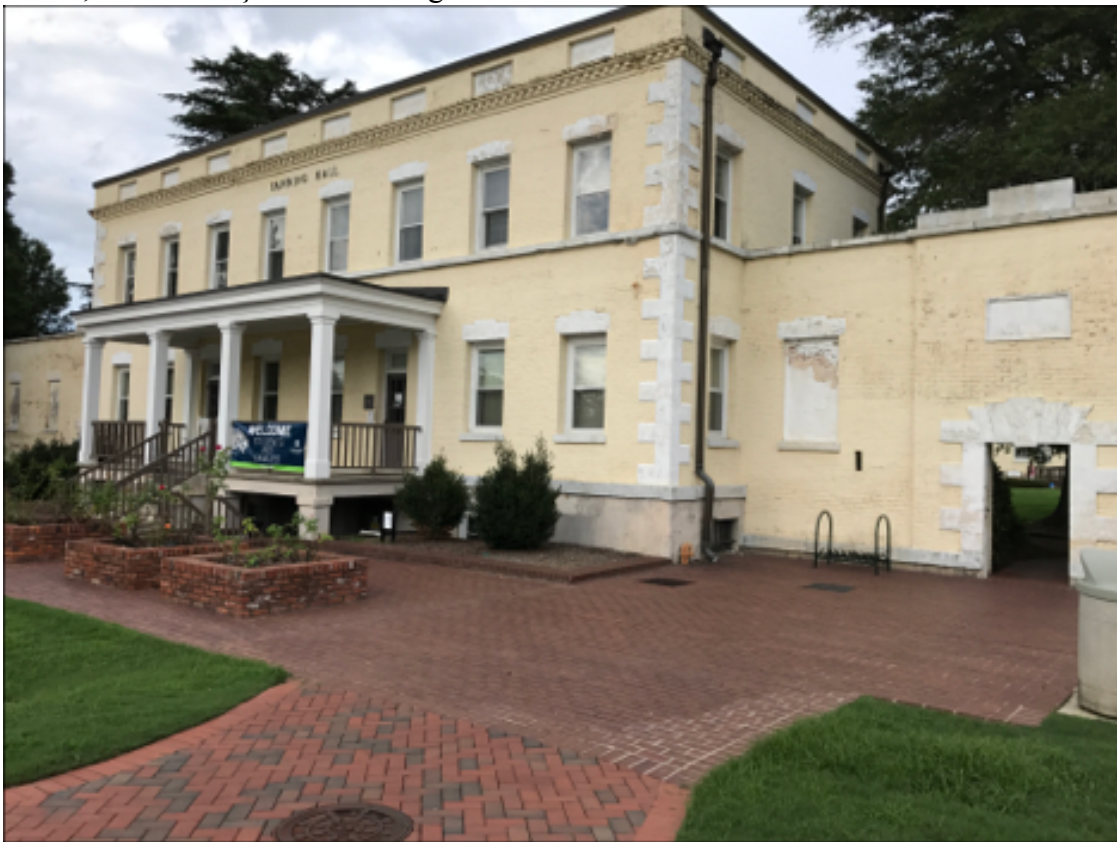
Figure 40, Close-up of western façade of Fanning Hall.
