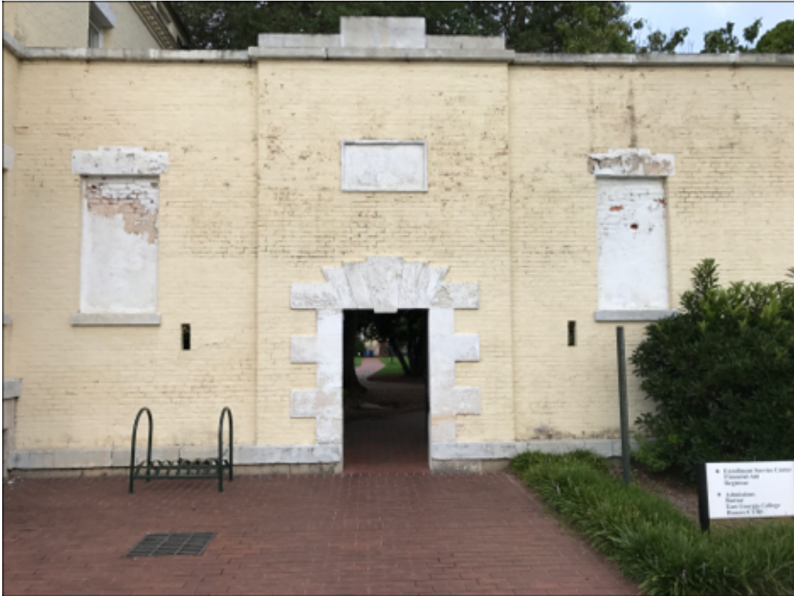
Figure 41, Loopholed wall connected to Fanning Hall.
