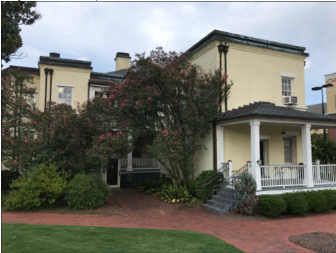
Figure 32, Western façade of Benet House.
