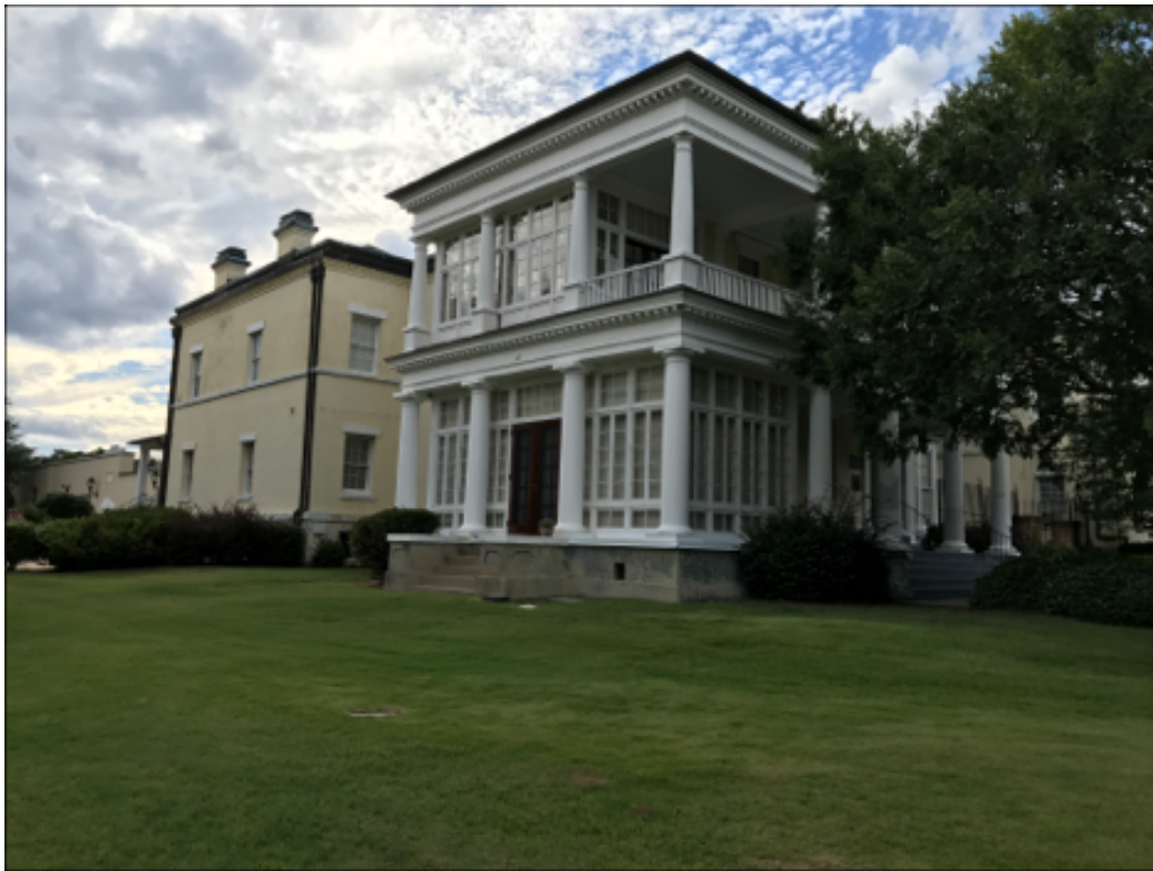
Figure 30, Southern façade of Benet House.
