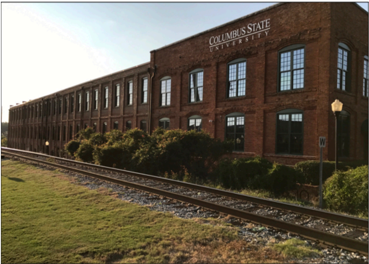
Figure 74, Current photograph of Drop-forge building with elevated railway and Columbus State University sign.
