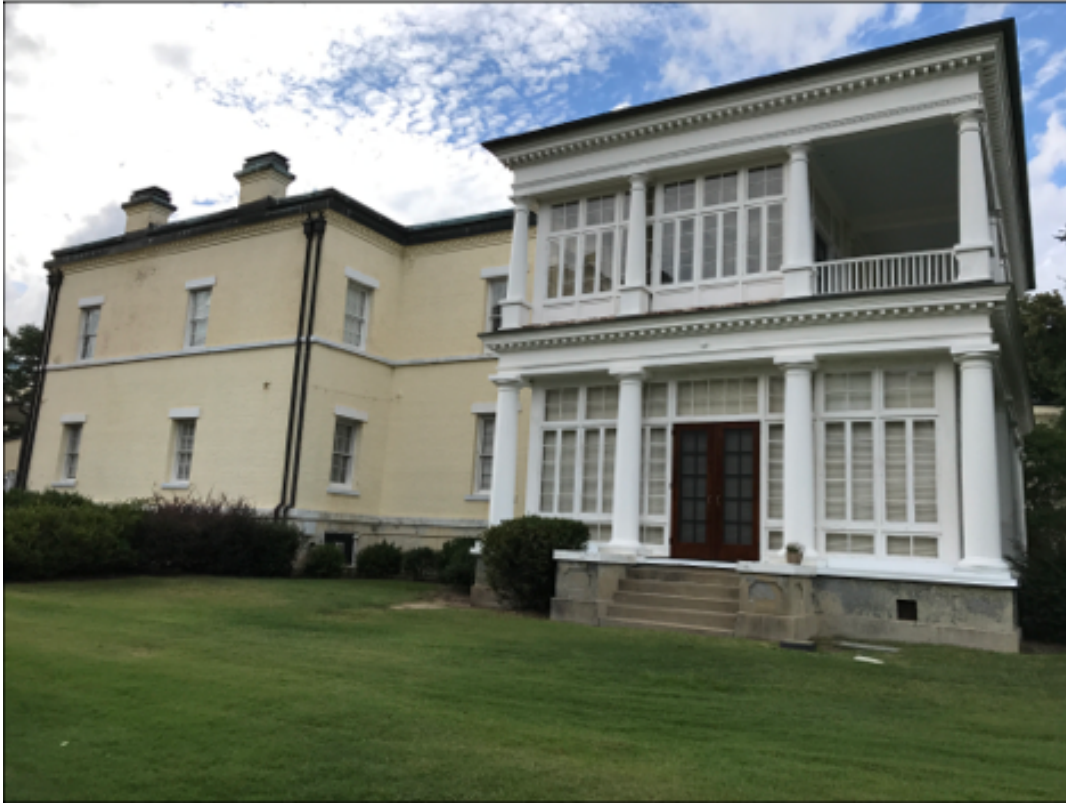
Figure 31, Southern façade of Benet House.
