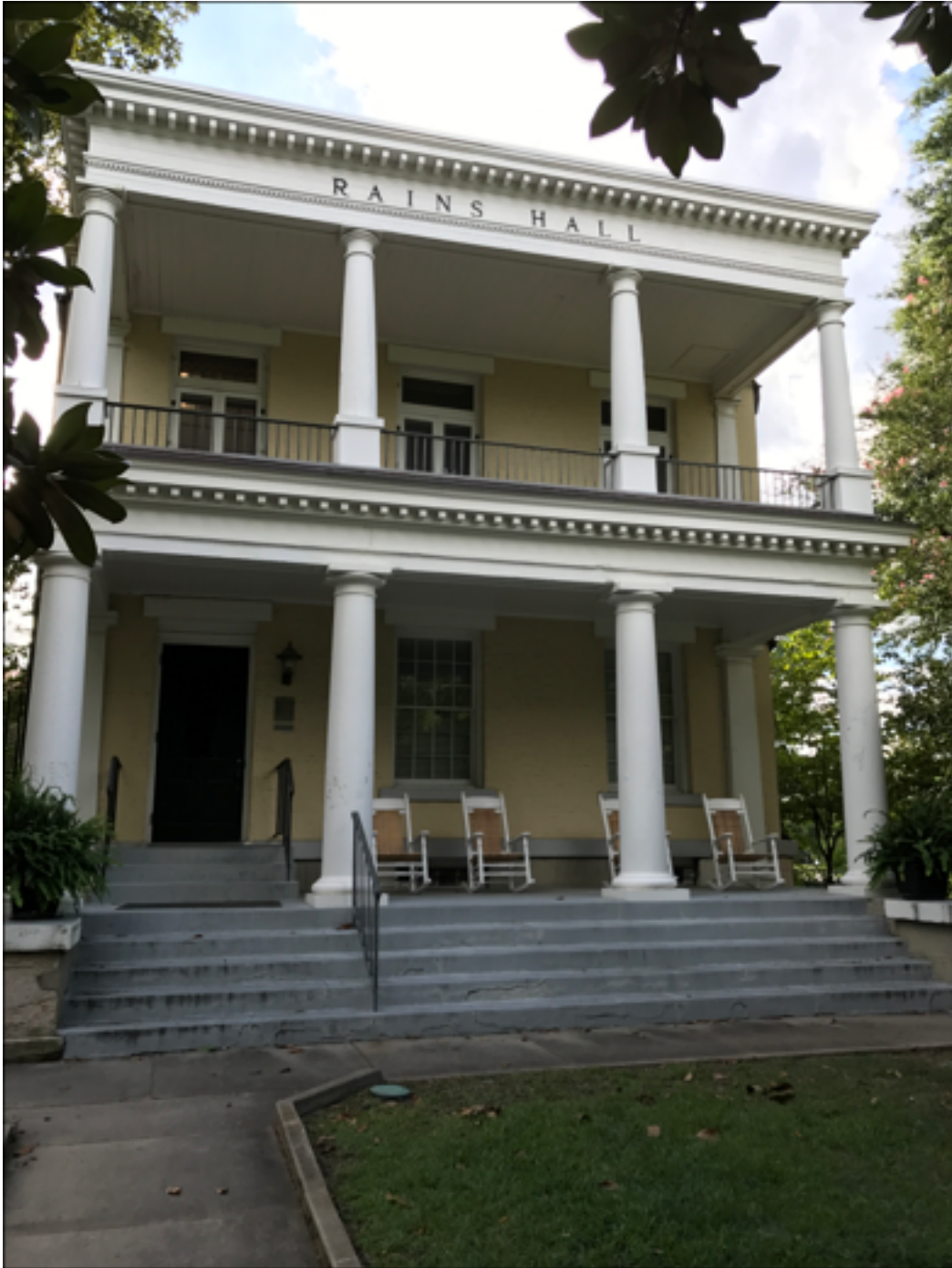
Figure 34, Close-up of eastern façade of Rains Hall.
