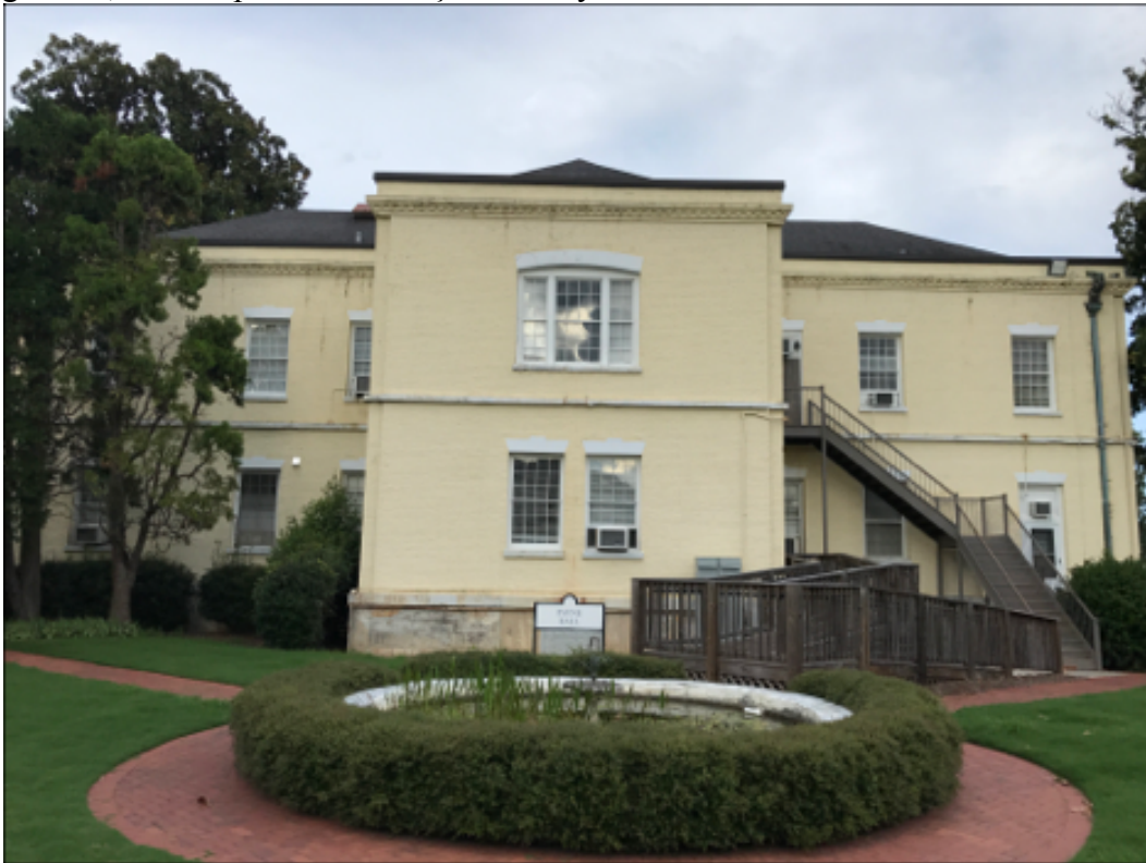
Figure 38, Western façade of Payne Hall.
