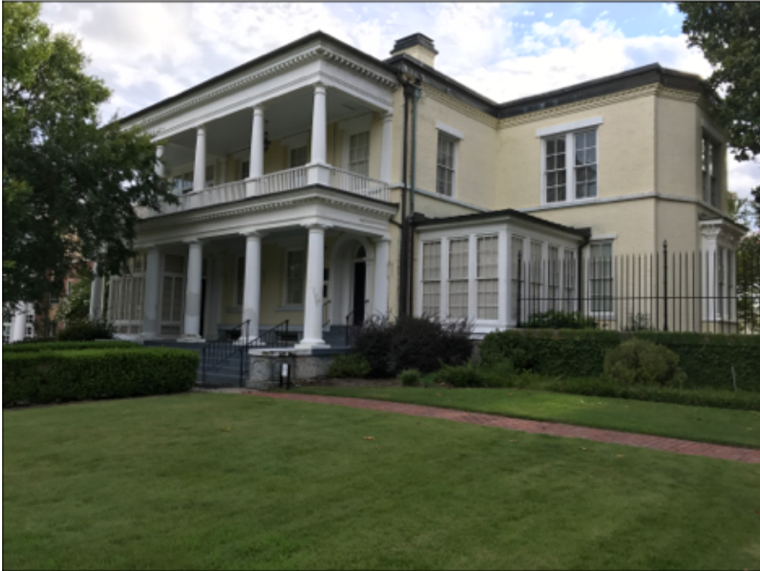
Figure 29, Eastern façade of Benet House.
