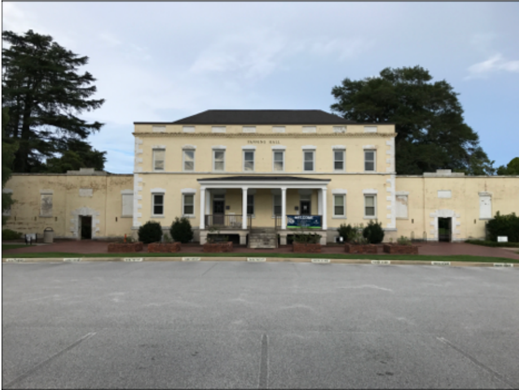
Figure 39, Western façade of Fanning Hall.
