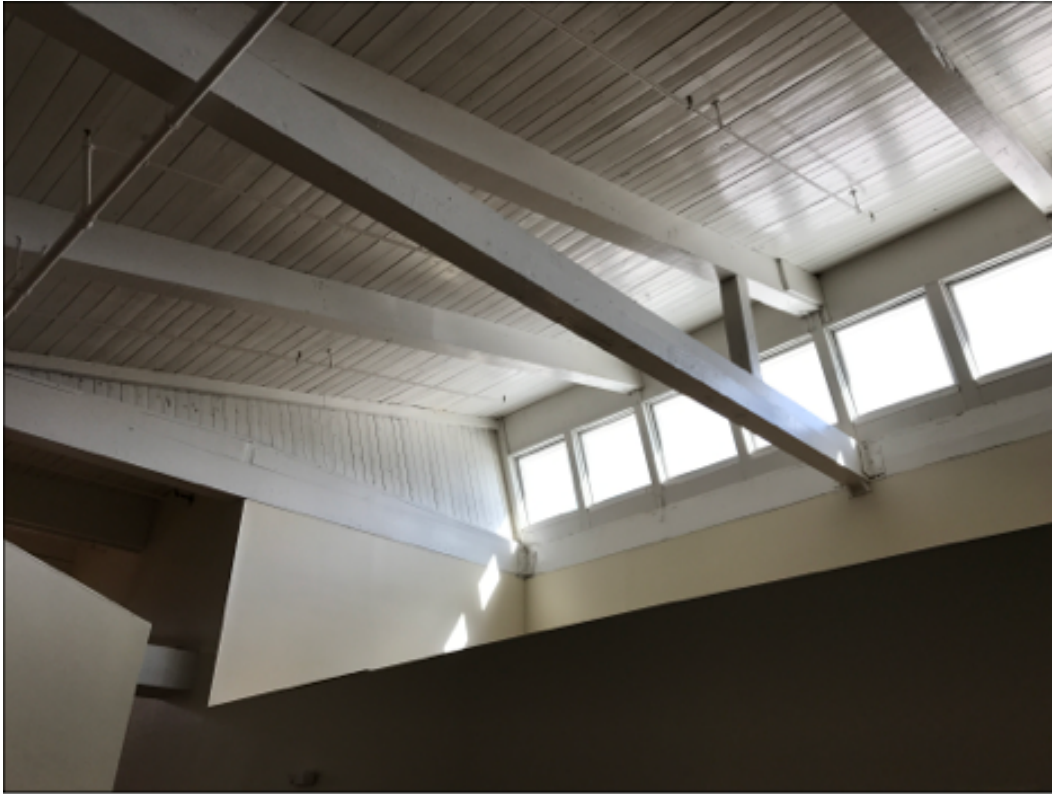
Figure 59, Massive timbers supporting roof of Cook and Brother Armory.
