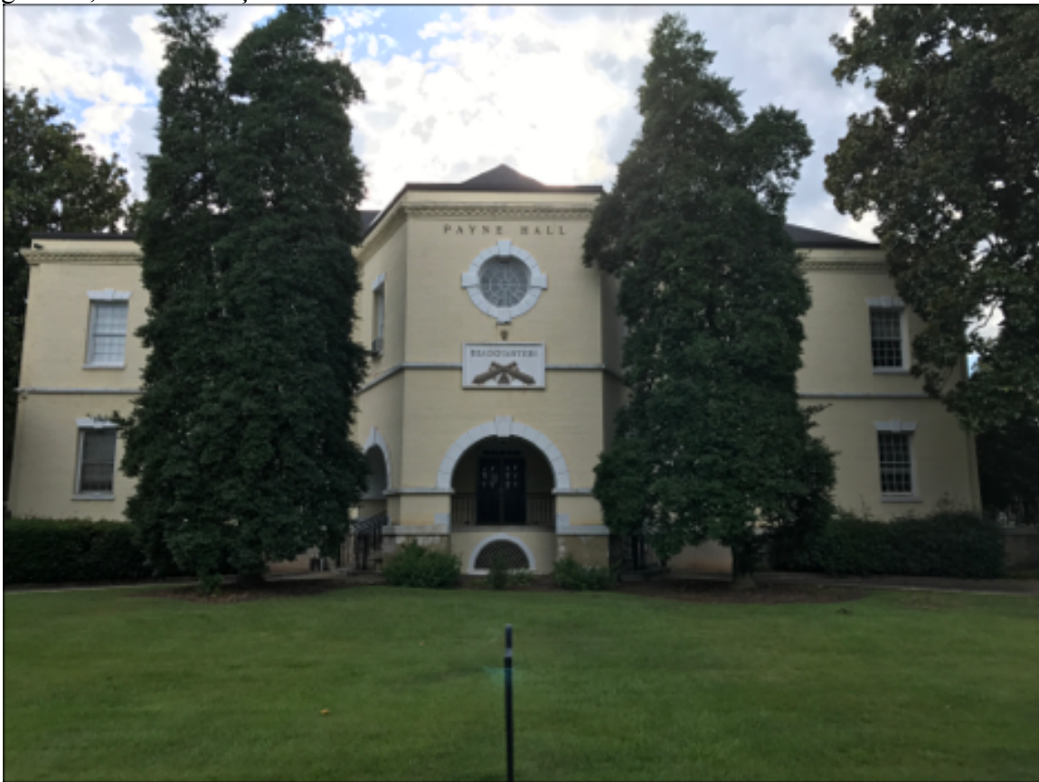
Figure 36, Eastern façade of Payne Hall.
