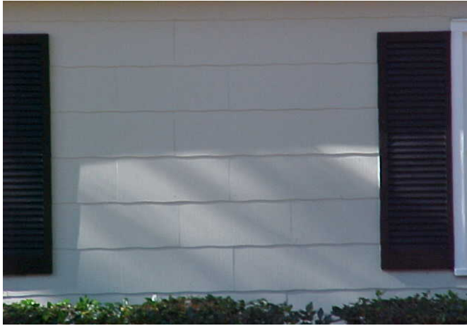
Figure 6. Example of asbestos shingle siding.
