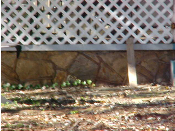
Figure 5. Example of continuous masonry foundation.
