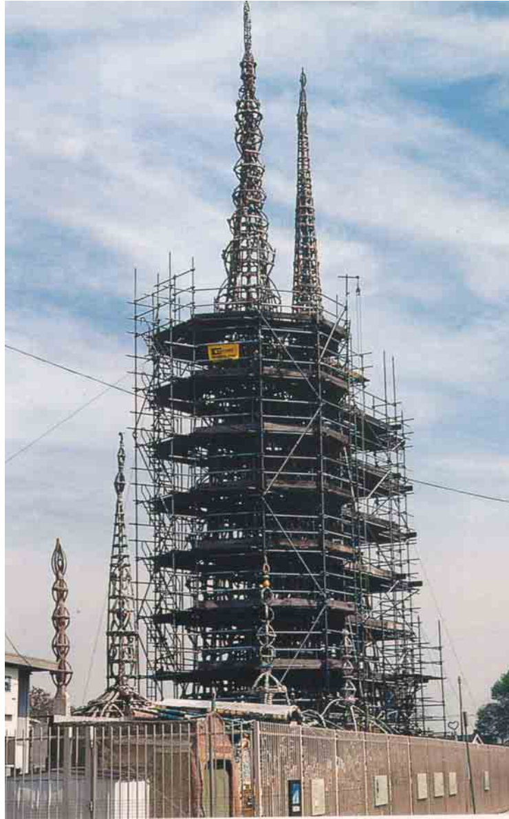
Figure 2.10 Preservation work on the Watts Towers in the early 1990s. From Goldstone.
