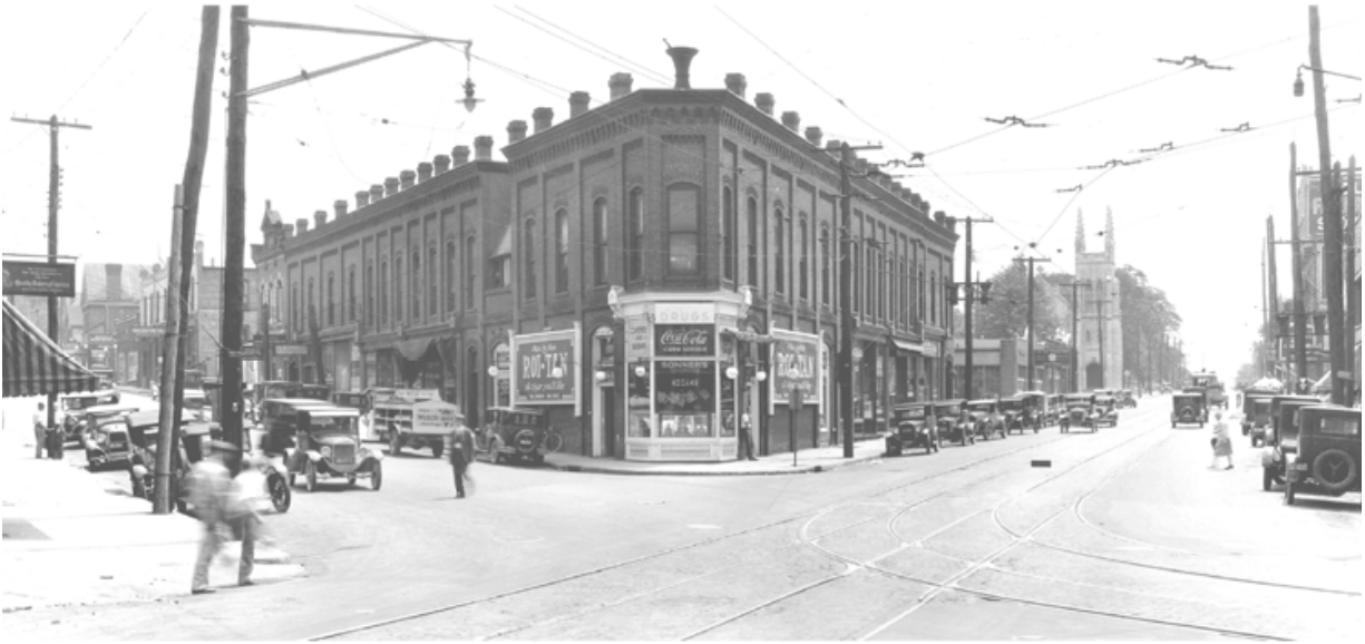
Figure 1.1: Intersection of North Central Street and Broadway, view South. (Knox MPC, 2007b)
