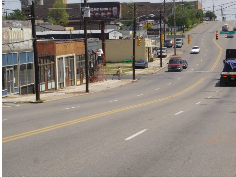
Figure 5.5: Existing Streetscape of North Central Street, view north from Oklahoma Avenue intersection. Photo by R.J. Justice
