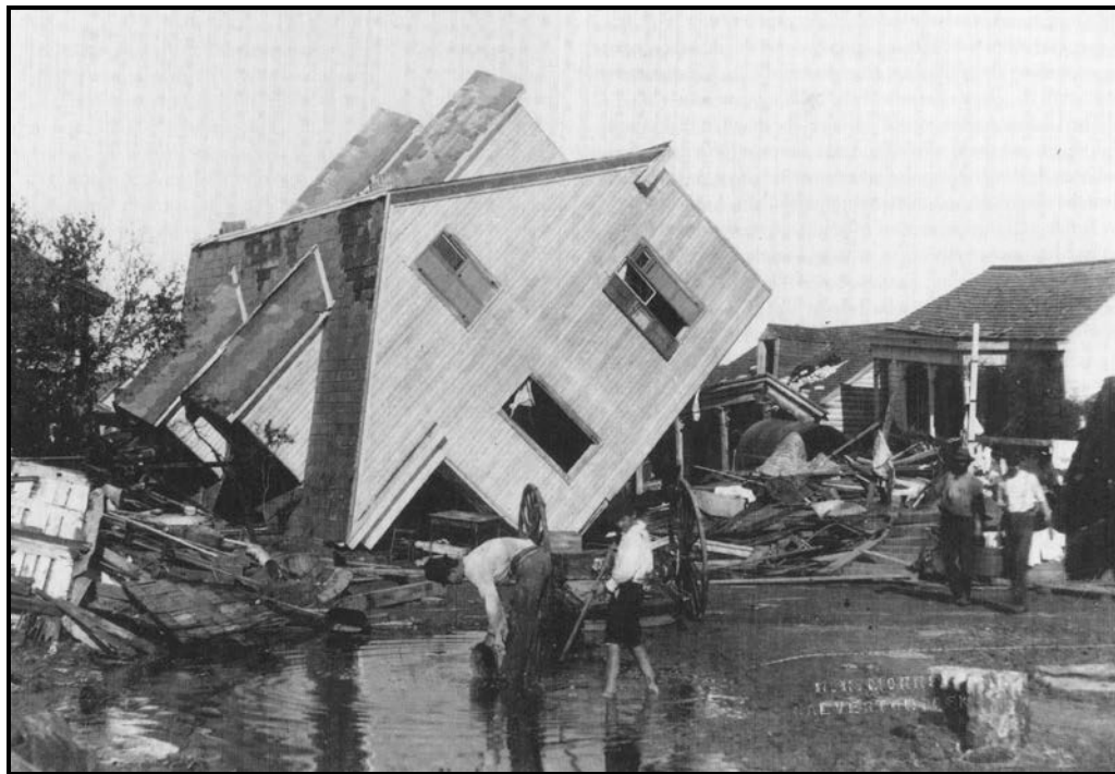
Figure 4. House wrecked after floating off its foundation. Source: Galveston Historical Society.
