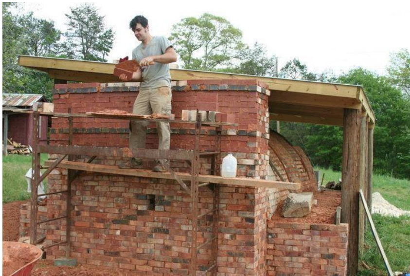
Figure 36. Alderman, Clint (2013). Clint rebuilding the kiln chimney.
