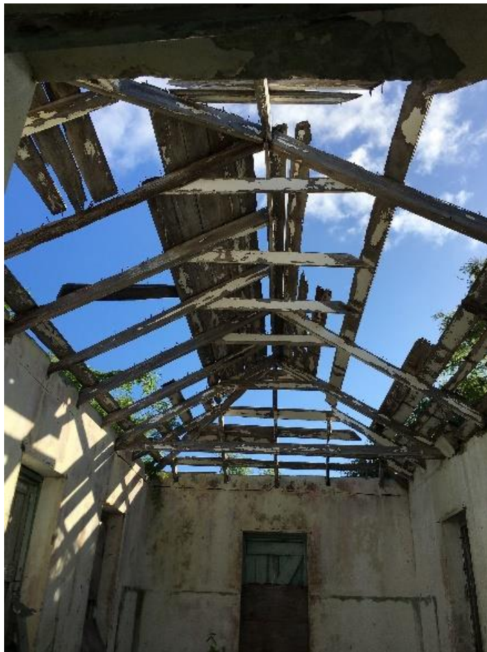
Figure 4.34 Original Lignum Vitae Framing – Dixon Hill Lighthouse. (Photo taken by the author, November 2017)
