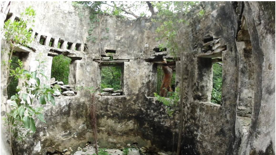
Figure 4.17 Latrine Interior – Fortune Hill Manor House Complex. (Photo by the author, November 2017)
