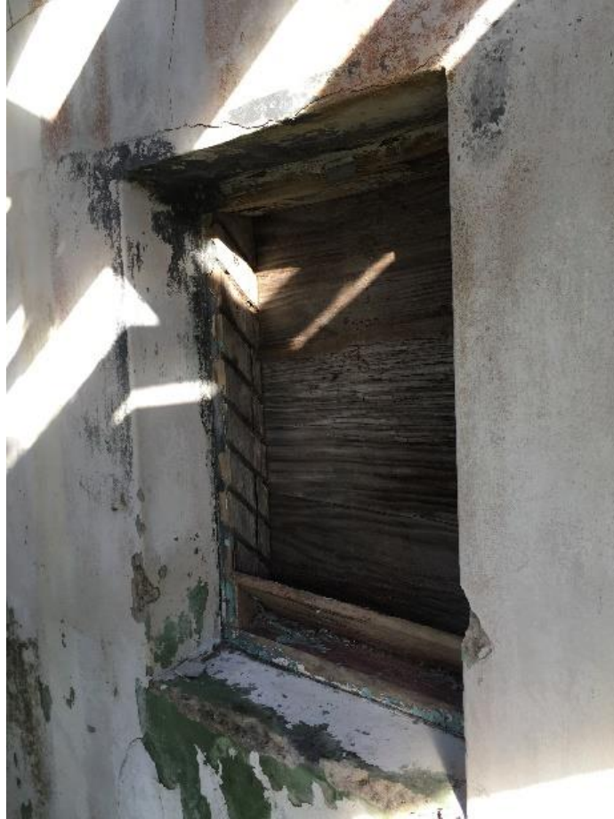
Figure 4.35 Original Window Framing for Fixed Louvers – Dixon Hill Lighthouse. (Photo taken by the author, November 2017)
