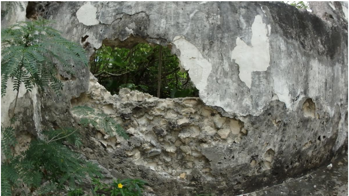
Figure 4.12 Detail of Tabby Wall Construction – Fortune Hill Manor House. (Photo by the author, November 2017).
