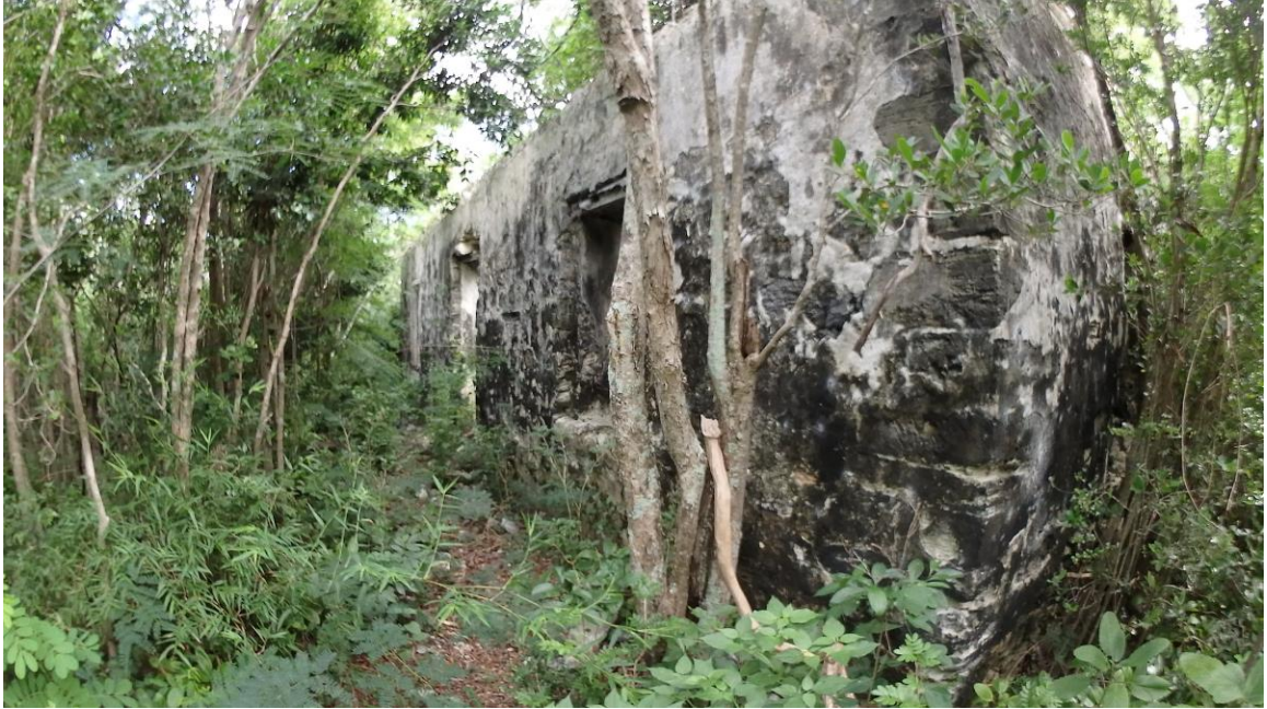
Figure 4.5 Industrial Building 'J' - Near cotton ginning circle in the Fortune Hill Plantation District Manor House Complex. (Photo by the author, November 2017)
