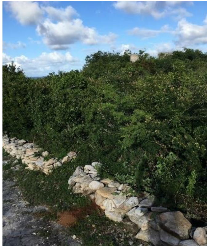
Figure 4.27 Stacked Rock Wall at Dixon Hill Lighthouse Driveway – Notice the walk-through opening. (Photo taken by the author, November 2017)
