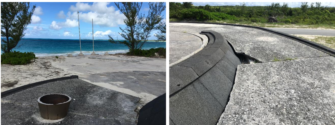
Figure 4.63 Poor Condition of Concrete and Flag Poles on the South Side of Land Fall Park. (Photo taken by the author, November 2017).
