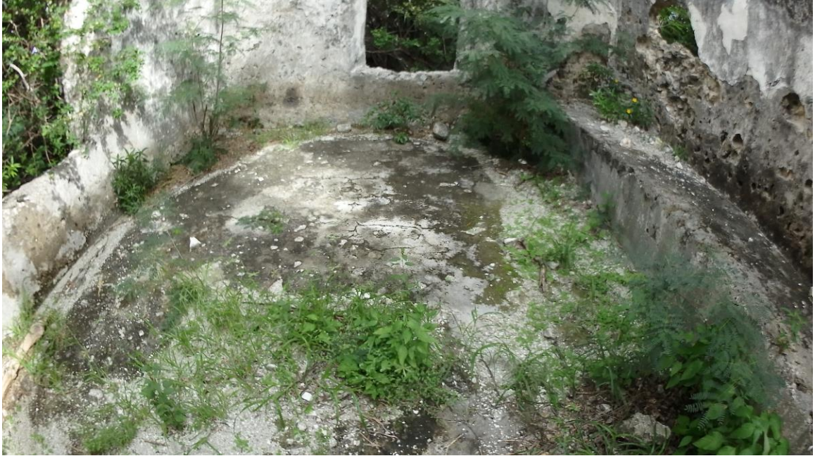
Figure 4.13 Raised Mortar Floor and Tabby Bench – Fortune Hill Manor House. (Photo by the author, November 2017)
