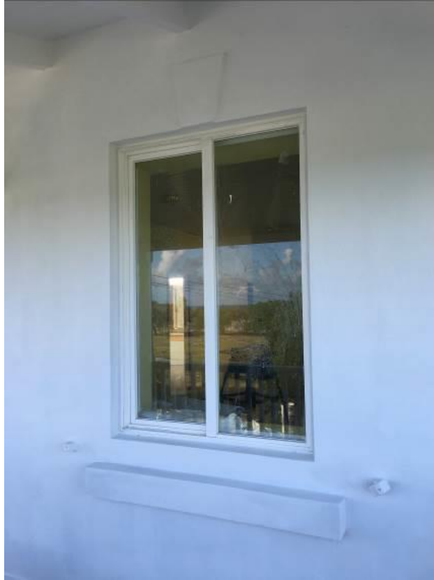
Figure 4.43 Glider Windows on North Keeper’s Quarters Building – Dixon Hill Lighthouse. (Photo taken by the author, November 2017)
