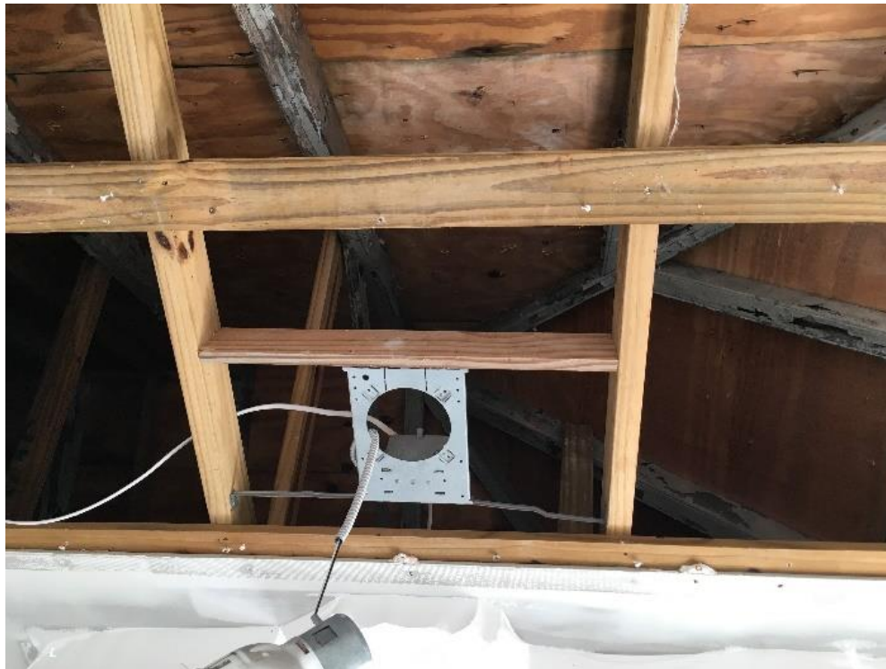
Figure 4.45 Old and New Framing Retrofit inside Public Bath House – Dixon Hill Lighthouse. (Photo taken by the author, November 2017)
