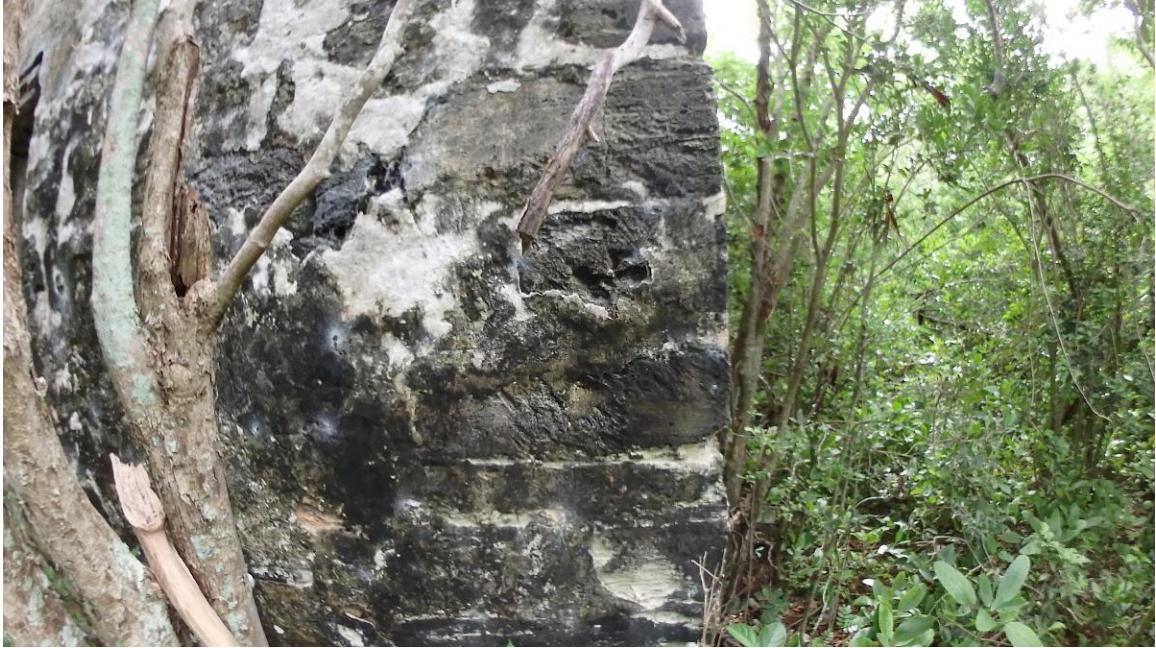
Figure 4.7 Detail of Cut Limestone Block Construction – Northeast corner of industrial building 'J' near cotton ginning circle in the Fortune Hill Plantation District Manor House Complex. (Photo by the author, November 2017)
