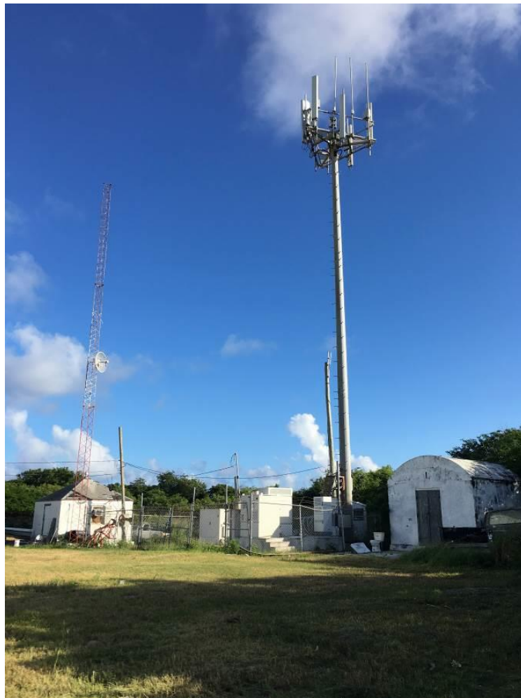
Figure 4.46 Communications Objects and Shed Buildings – Dixon Hill Lighthouse. (Photo taken by the author, November 2017)
