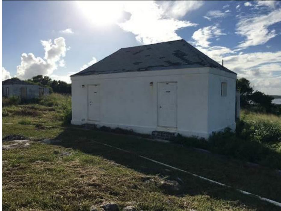
Figure 4.44 Exterior Condition of Public Bath House – Dixon Hill Lighthouse. (Photo taken by the author, November 2017)
