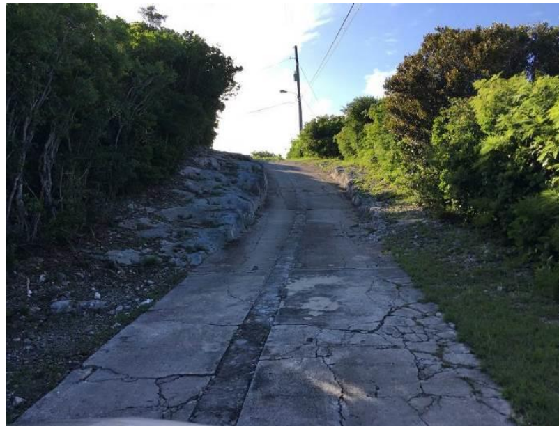
Figure 4.25 Driveway to Dixon Hill Lighthouse Facing West – Notice the exposure of cut-out in bedrock. (Photo taken by the author, November 2017)
