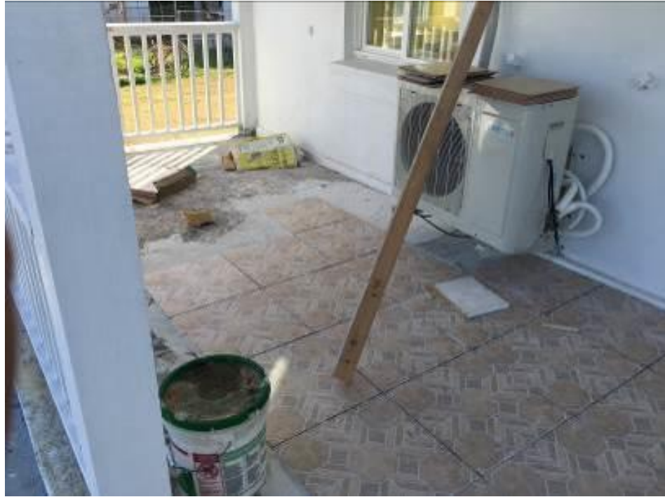
Figure 4.41 Tile Installation on Front Porch of South Keeper’s Quarters Building – Dixon Hill Lighthouse. (Photo taken by the author, November 2017)
