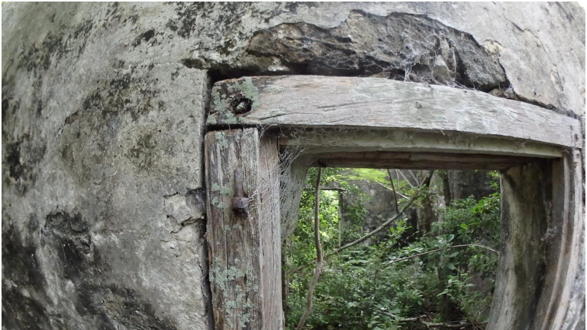
Figure 4.6 Lignum Vitae Window Framing – Industrial Building 'J' near cotton ginning circle in the Fortune Hill Planation District Manor House Complex. (Photo by the author, November 2017)
