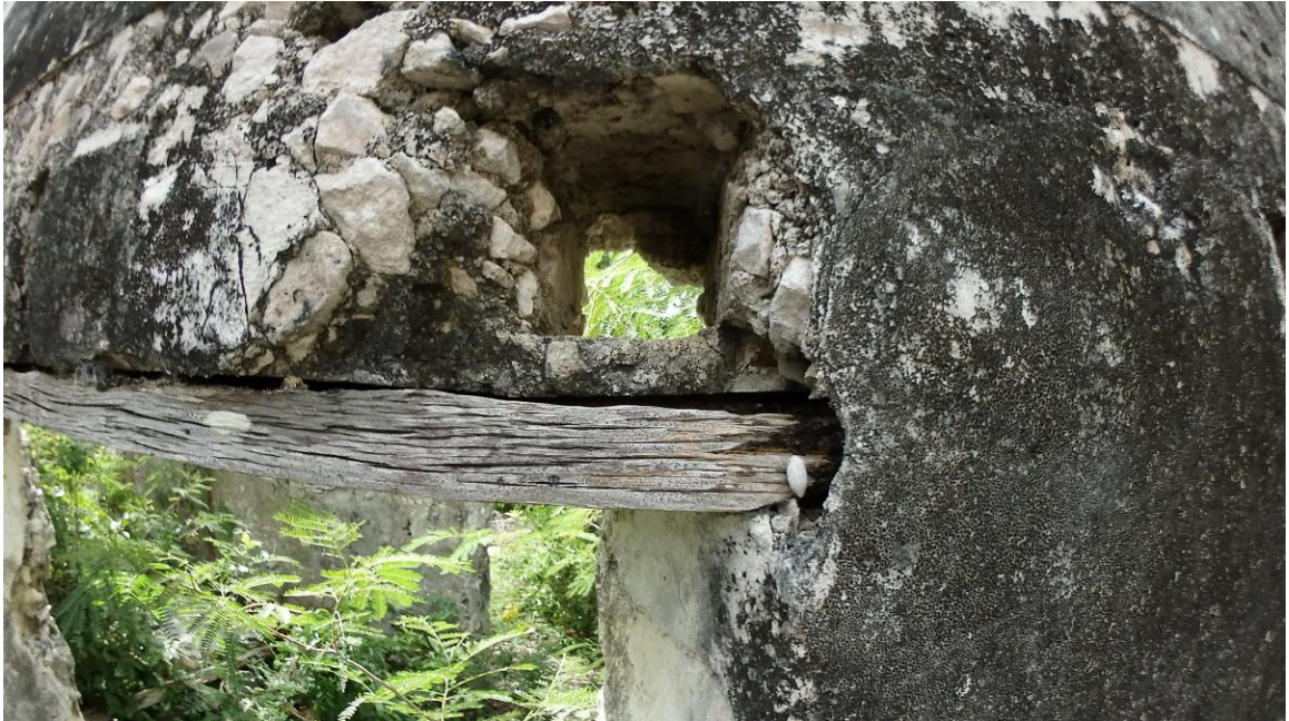
Figure 4.16 Detail of Lignum Vitae Lintel – Library at Fortune Hill Manor House Complex. (Photo by the author, November 2017)
