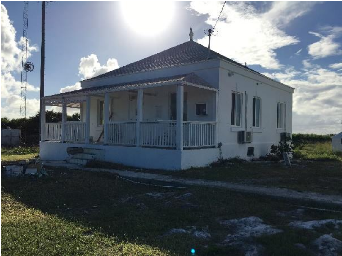
Figure 4.40 South Keeper's Quarters Building – Dixon Hill Lighthouse. (Photo taken by the author, November 2017)
