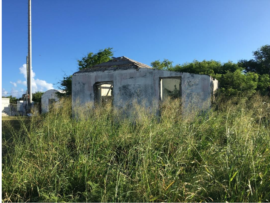
Figure 4.47 Abandoned Structure – Dixon Hill Lighthouse. (Photo taken by the author, November 2017)
