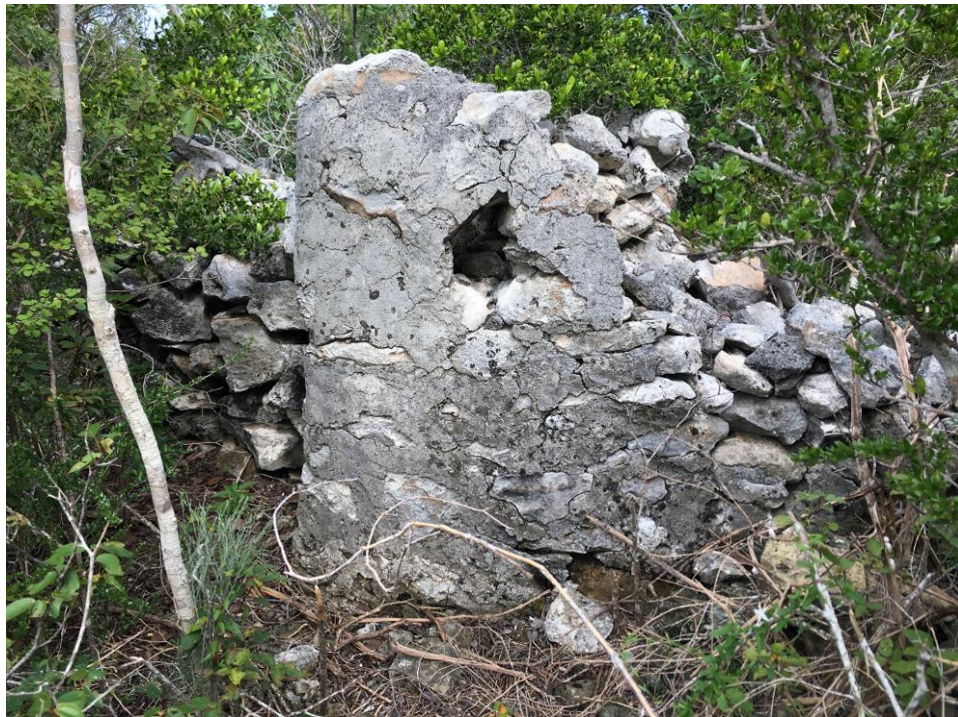
Figure 4.20 Stone Wall with Lime Mortar – Fortune Hill Plantation District. (Photo by the author, November 2017)
