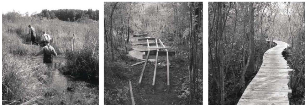
Figure 27. Constructed by hand to limit impact on surrounding ecosystem (SOURCE: Amazing Trace, Landscape Architecture Magazine, August 2012)
