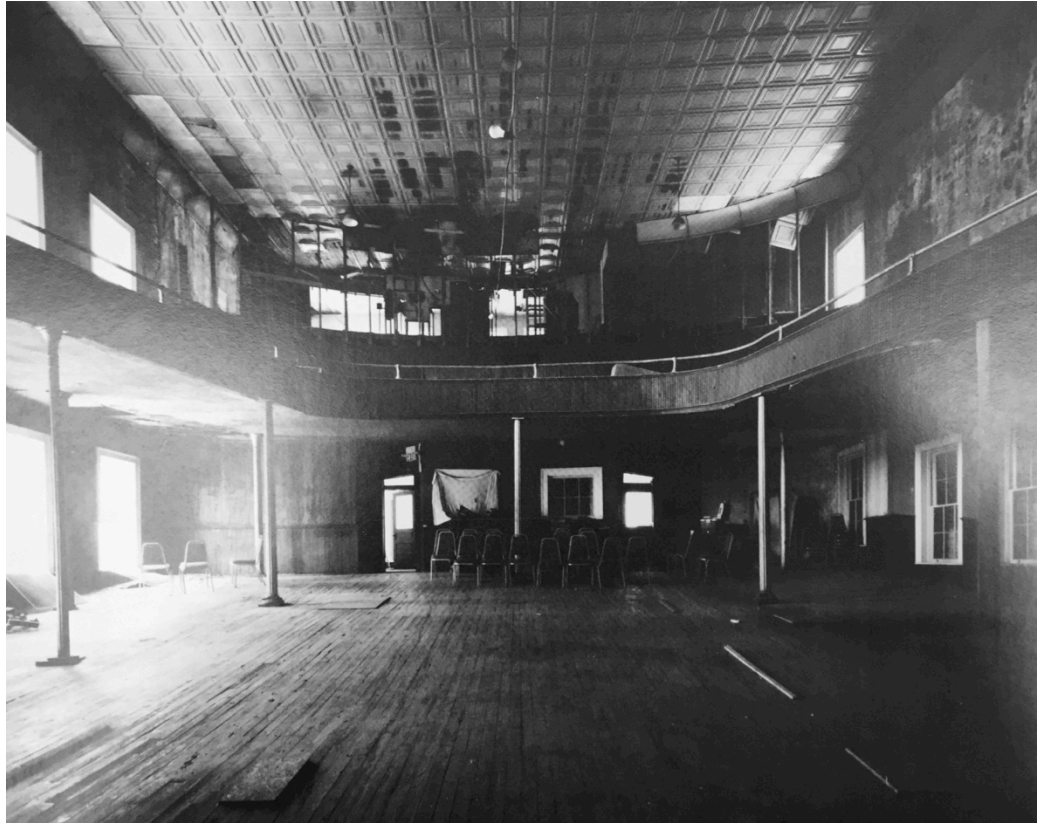
Figure 41 - Morton Theatre before restoration. Courtesy of Morton Theatre.
