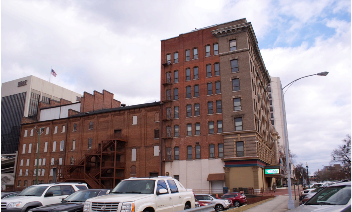
Figure 37 – Macon Grand Opera House side elevation as seen today. Photograph by the author.
