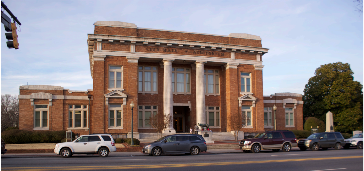
Figure 71 - Rome City Auditorium façade as seen today. Photograph by the author.
