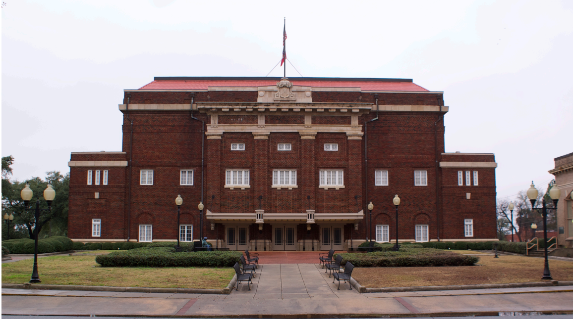
Figure 60 - Albany Municipal Auditorium façade as seen today. Photograph by the author.
