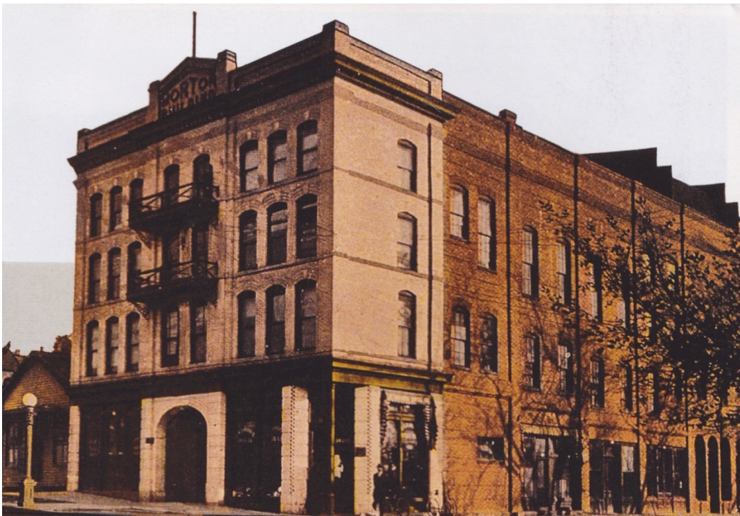
Figure 4 - Morton Building with "Pink" Morton. From "Encore Performance." Preservation , August 1, 2012.
