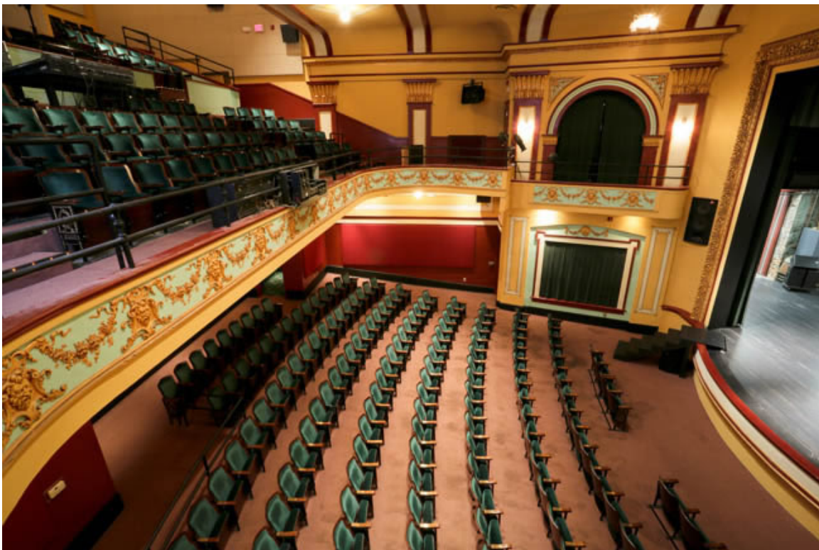
Figure 40 - Douglass Theatre interior as seen today. Photograph from Charles R. Sheridan & Co. General Contractors website ( http://www.chrissheridan.com/douglasstheatre.html )
