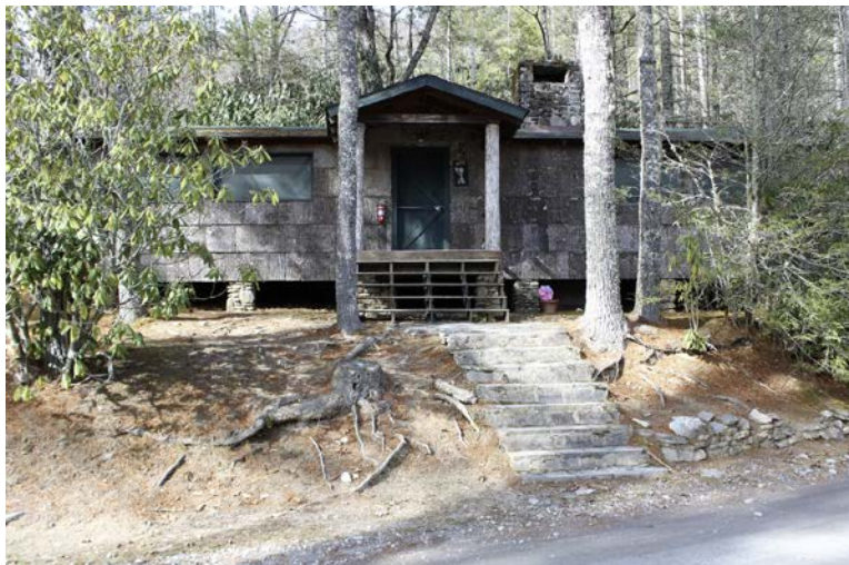
Figure 6.53. A view of Wit's End from the road (Source: Author)
