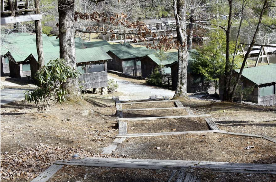
Figures 6.10: View of mulch-filled and stone stairs down to cabin lines (Source: Author)
