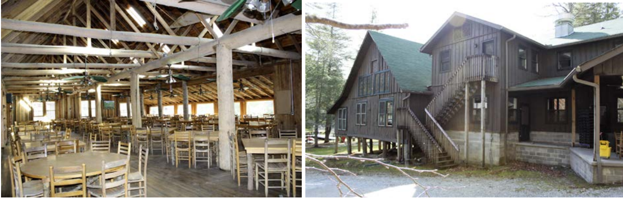
Figure 6.14 and 6.15. Interior of Dining Hall and rear with attached two-story housing and kitchen (Source: Author)
