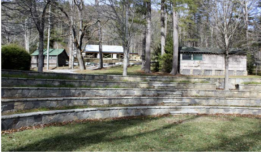
Figure 6.32. Close-up of Chapel showing grass covered seating rows and trees in between seating rows (Source: Author)
