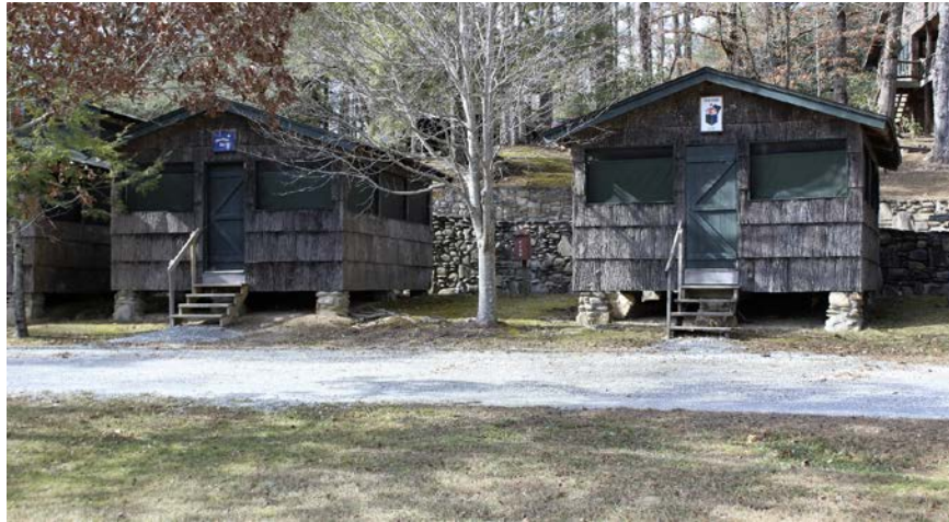
Figure 6.46. A close-up of two cabins, Moonlight Bay and Chatter Box (Source: Author)
