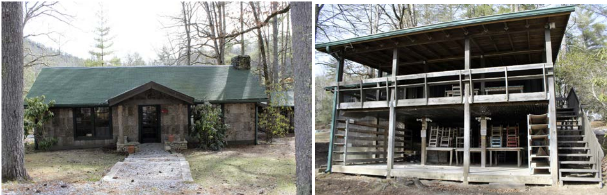
Figure 6.23 and 6.24. The front of the Arts & Crafts Lodge from the Merrie-Woode Road and the rear of the Arts & Crafts Lodge, the area under the porch houses ceramics, (Source: Author)
