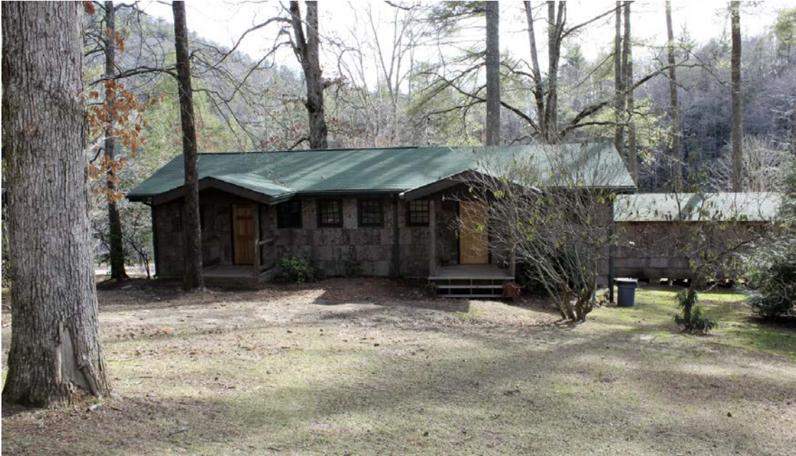
Figure 6.25. View of Bang Shop (on left) and Gem Box (on right) from Merrie-Woode Road (Source: Author)
