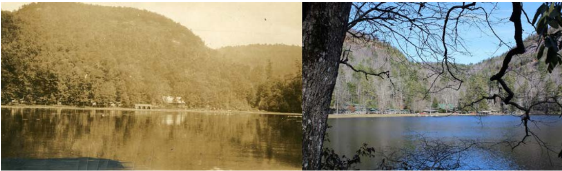
Figure 7.2. View of Merrie-Woode from Camp Road during 1920s (left) and 2017 (right). (Source: Camp Merrie-Woode Archives and Author)
