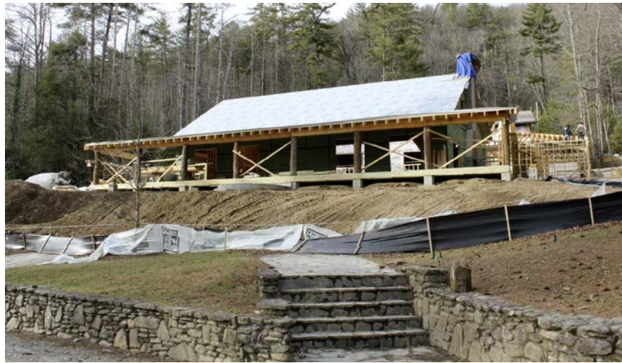
Figure 6.11: Castle reconstruction in progress (Source: Author)
