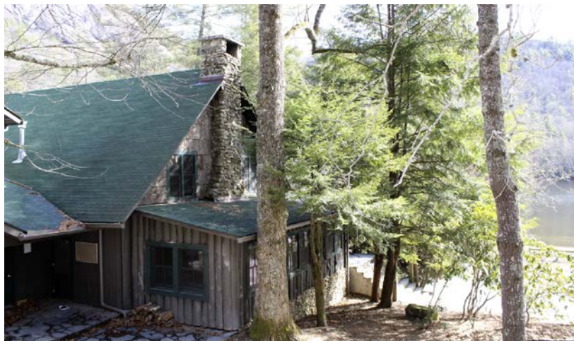
Figure 6.13. Western facade of Dining Hall, note the split log addition with shed roof that wraps around the chimney, (Source: Author)
