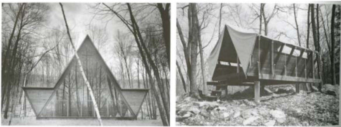
Figures 4.15 and 4.16. Village Hall and camper tent at Camp Bliss, 1953-1954, markedly more modern than the rustic buildings that dominated the first half of the twentieth century. (Source: Van Slyck, A Manufactured Wilderness, 216)
