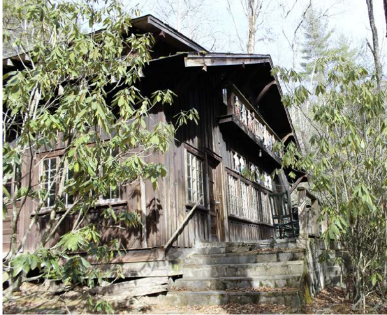
Figure 6.16. View of southwestern corner of Tajar (Source: Author)
