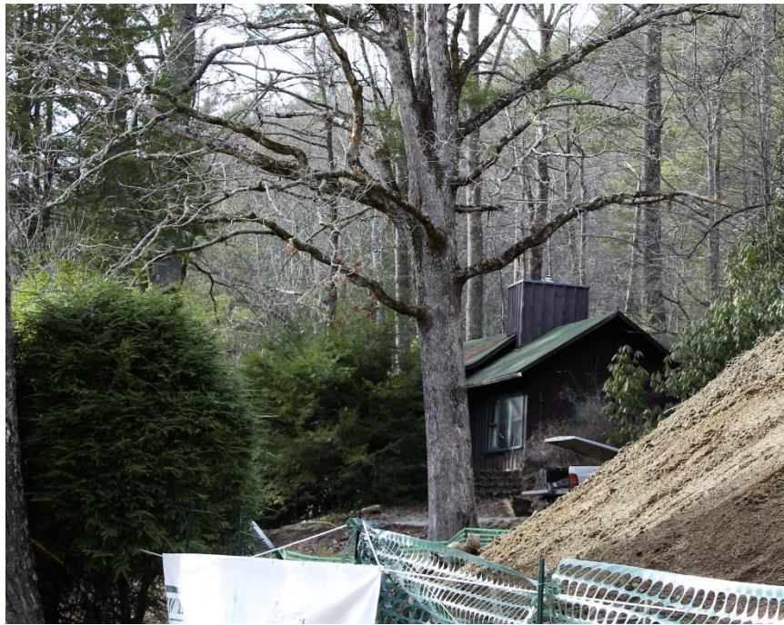
Figure 6.34: View of Gate House from Merrie-Woode Road over Castle construction site, (Source: Author)
