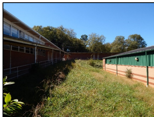
Figure 6.15 1956 Cafeteria Building (Photo credit: Bryan Hardman)
