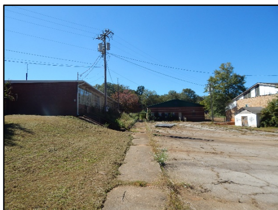
Figure 6.18 Front View of 1996 Gym (Photo credit: Bryan Hardman)
