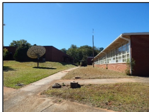
Figure 6.14 1956 Classroom Building (Photo credit: Bryan Hardman)
