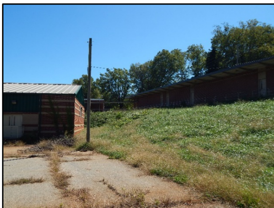
Figure 6.16 View of 5 th Grade Building (Photo credit: Bryan Hardman)
