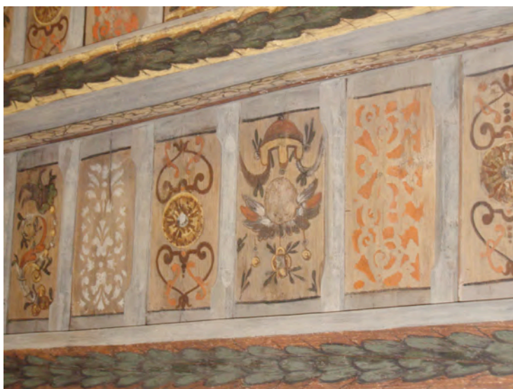
Figure 29: Painted Roof Rafters in the Schoenborn Palace 31
