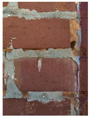
Fig. 5.17: Author. *Brick in downtown* commercial district with deteriorated mortar, which has been haphazardly covered with concrete as a "quick fix." 2016. Photograph.
