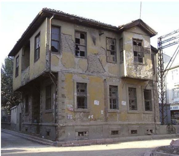
Figure 4.1. Original (pre-fire) condition of the subject building in Konya. 61
