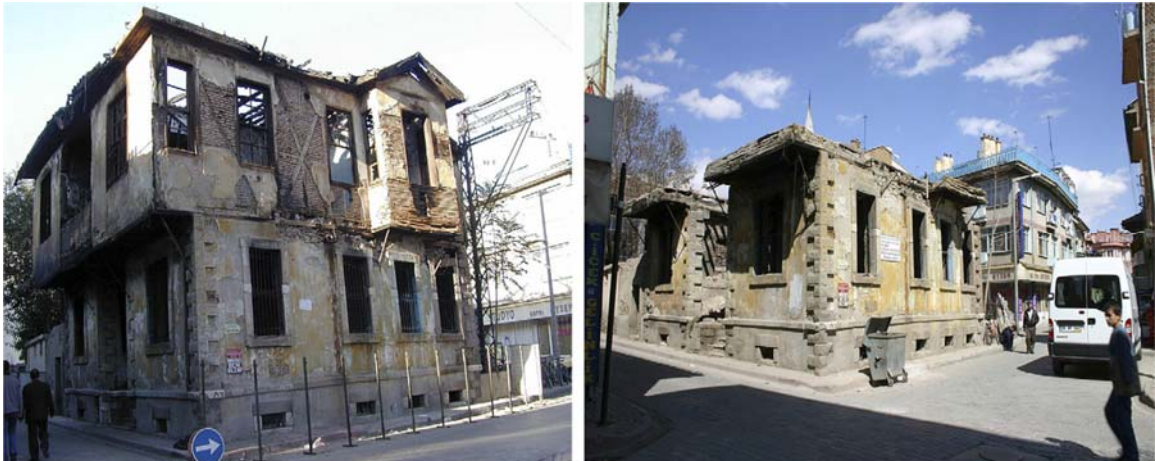
Figure 4.2. Post-fire conditions after fire one (left) and fire two (right). 61
