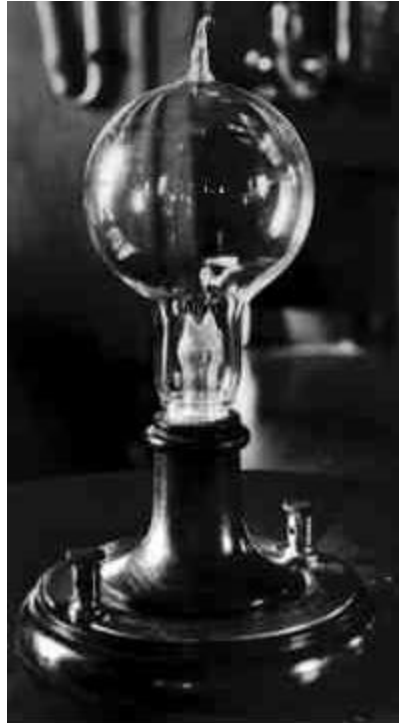
FIGURE 4: Replica of the First Incandescent Bulb Demonstrated by Thomas Edison in 1879 (Source: The Inventions of Thomas Edison, url: http://inventors.about.com/library/inventors/bledison.htm )
