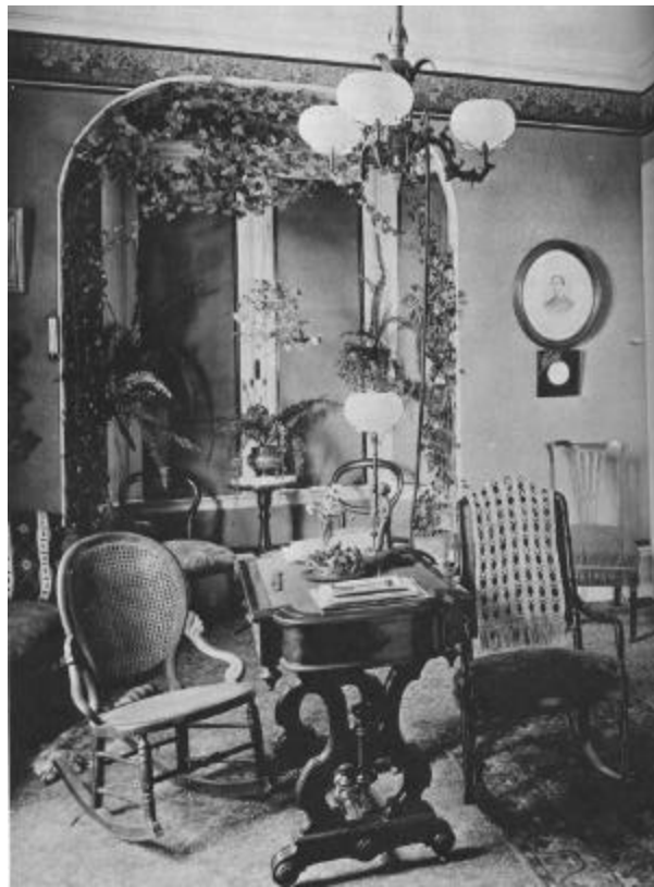
FIGURE 59: Gas Table Lamp being Supplied Gas by a Flexible Hose from the Gasolier (Published in Myers, Gaslighting in America: A Guide for Historic Preservation , 1978)
