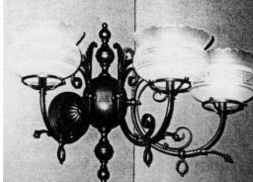
FIGURE 123: Fiber optics Used to Retrofit Period Gas Fixtures in the Georgia State Capitol (Published in Kay, "Historic Lighting- Saint or Sinner?," Journal of Architectural Conservation , (March 2002)
