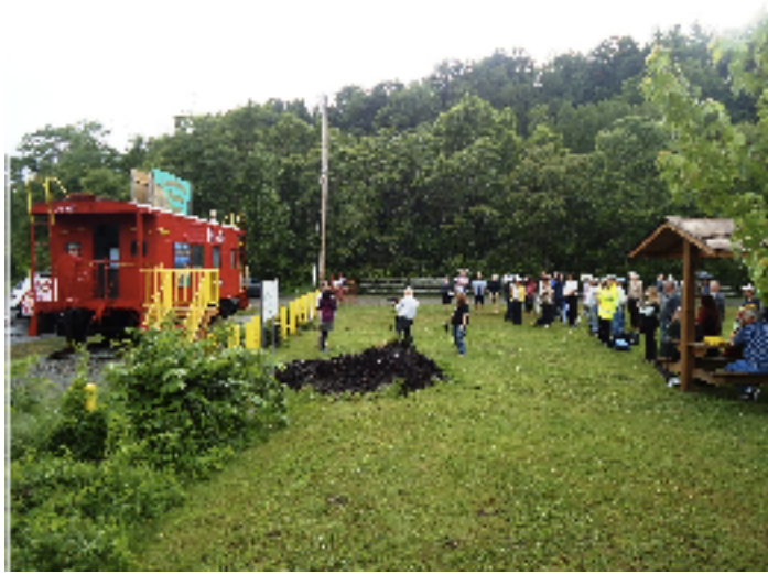
Figure 3.1: The Connellsville, Pennsylvania caboose rehabilitated into a Visitor's Center. 157
