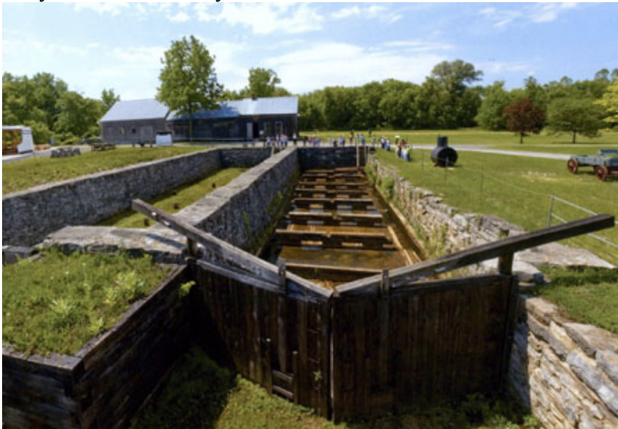
Figure 2.13: A dry dock at the Chittenango Landing Canal boat Museum. Dry docks were used to aid in boat repair, particularly to the underside of the vessel. 149
