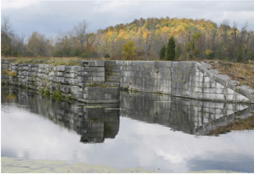
Figure 2.12: A historic lock on the Erie Canalway Trail in Lyons, New York. Less than 100 of the early stone locks remain; most were replaced by concrete in the early twentieth century. 148
