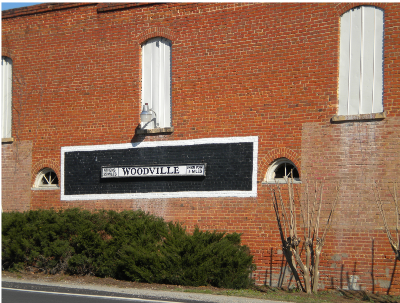
Figure 4.13: The Woodville Depot sign is located on the side of a building. It is unclear whether this was the original depot, or if the sign has been moved. 231
