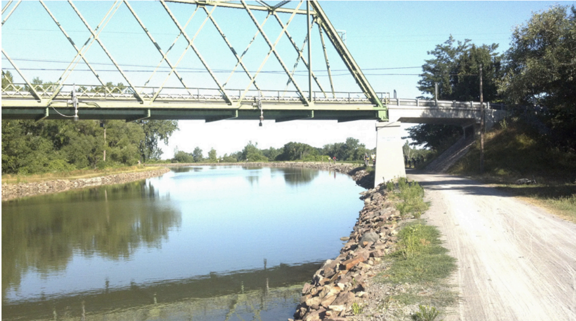
Figure 2.4: The former towpath now serves as the primary trail along the Erie Canalway. 66
