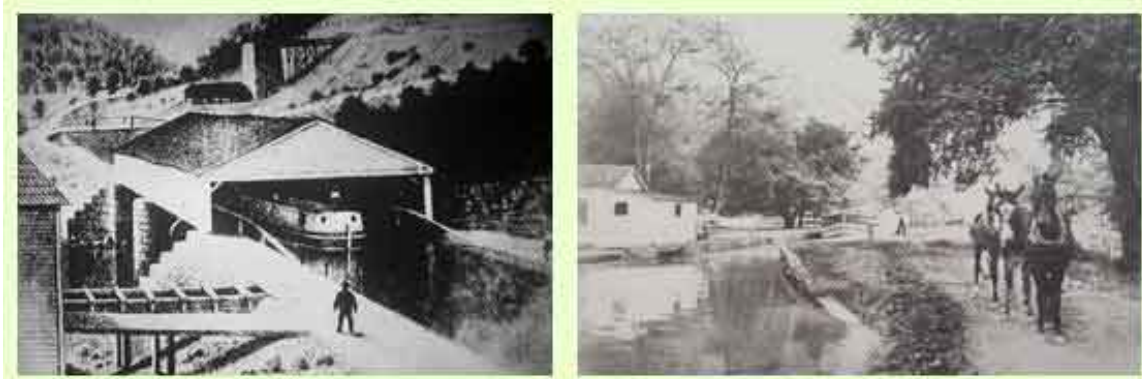
Figure 2.6: Cargo traveling on the Main-Line Canal had to complete several steps to cross the Allegheny Mountains. Cargo was loaded onto a barge, then transferred to a railroad car to cross the Allegheny Mountains, and then reloaded onto barges to complete the journey across the state. 77
