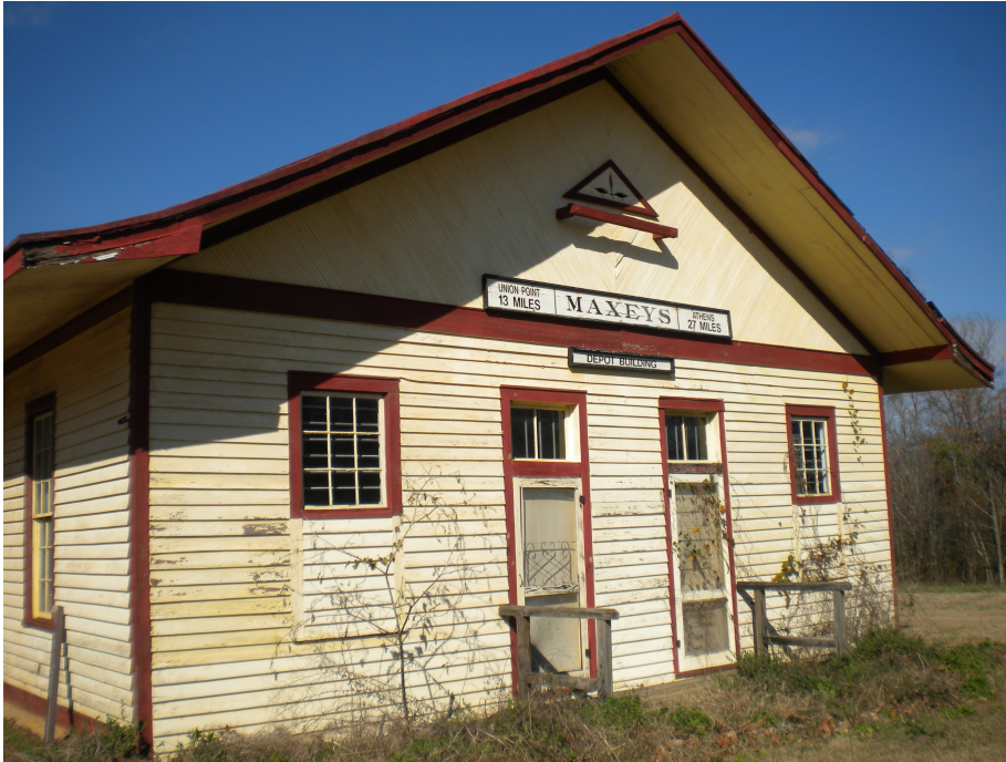
Figure 4.12: The Maxeys Depot. The structure was for sale at the time of this photo and is in obvious need of repair. 230
