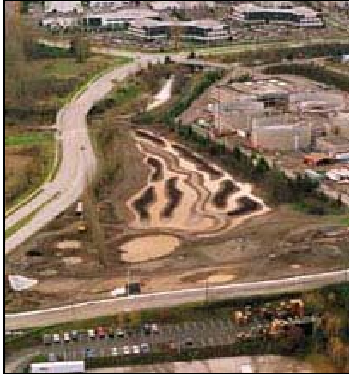
Figure 3 - Aerial view of Waterworks Gardens during construction (Ned Ahrens)
