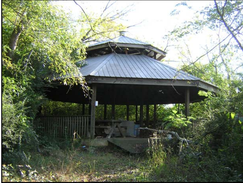
Figure 25 - Covered structure on south edge of granite outcrop
