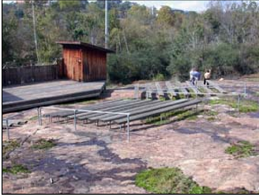
Figure 23 - Tommy Harris Amphitheater below retaining wall (David Porter)
