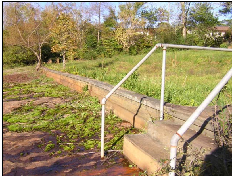
Figure 22 - Retaining wall on granite outcrop
