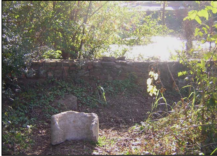
Figure 17 - Historic stone and brick wall
