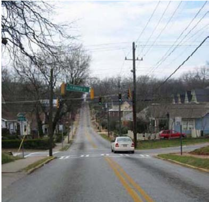
Figure 5.29. View looking east on Hancock
