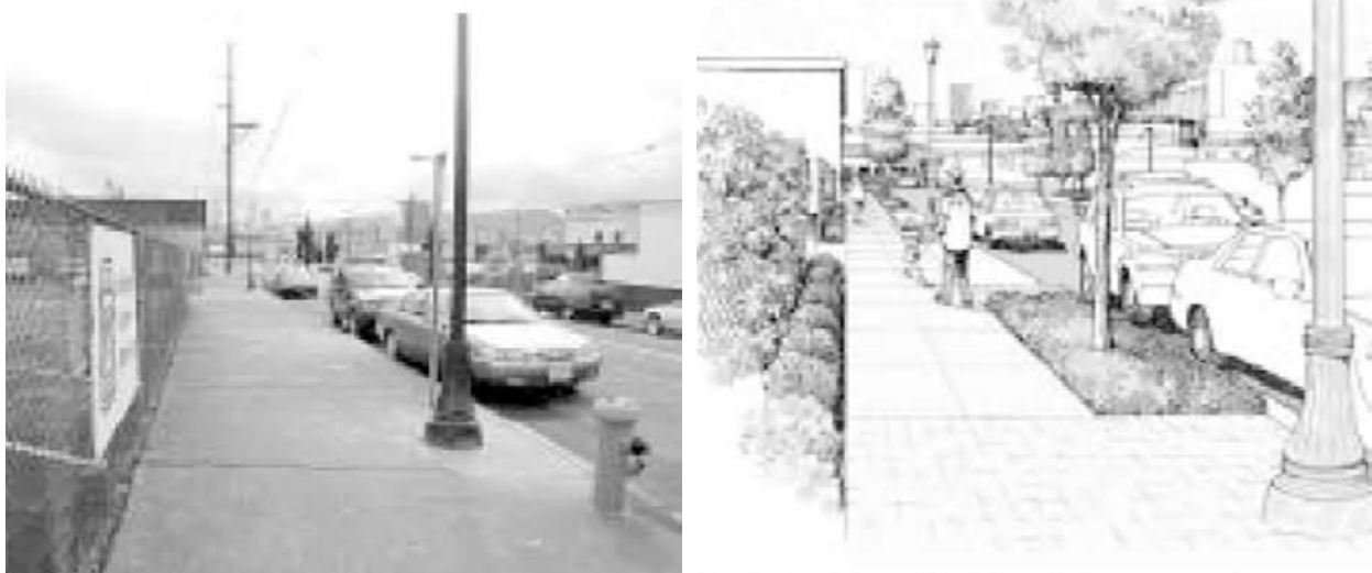
Figure 4.6. N. Mississippi Ave streetscape improvements. (City of Portland 2003)
