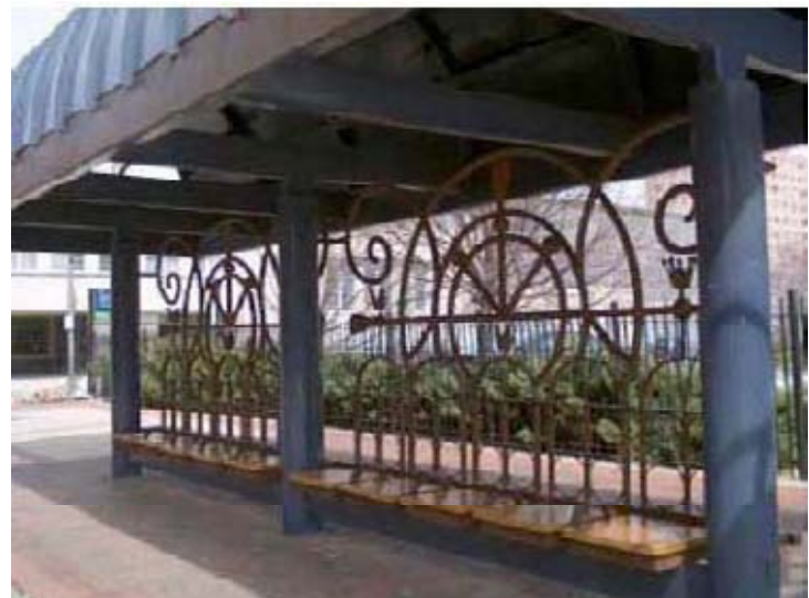
Figure 4.17. Unique bus shelter. (City of Baltimore 2005)
