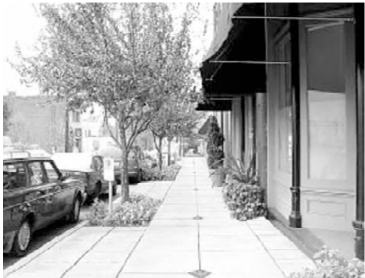
Figure 4.11. Sidewalk markers. (City of Portland 2003)
