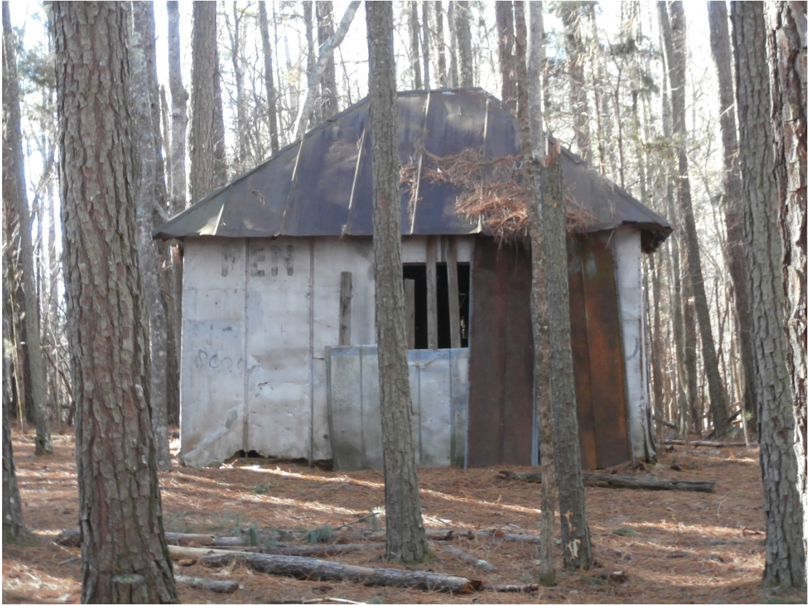
Figure 38. East elevation of men's restroom, facing the track. (Photo Credit Author)
