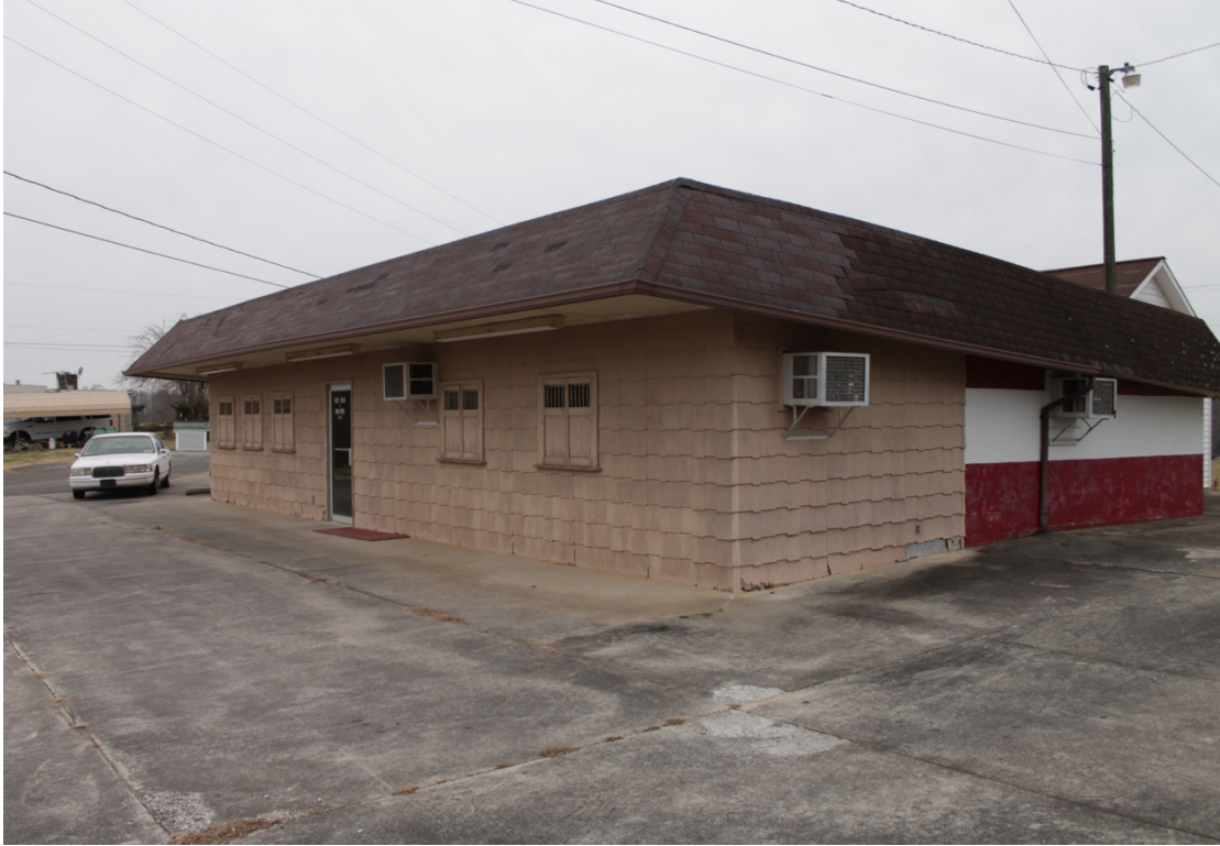
Figure 10. Ticket office with additions converted from what was once a chicken coop. (Photo Credit Jacob Cook).
