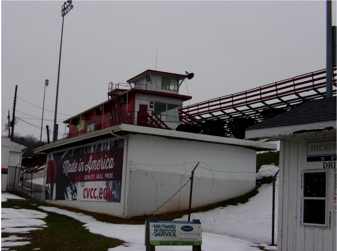
Figure 57. Northwest oblique of men's restroom, representative of three restrooms on the site. (Photo Credit Author)
