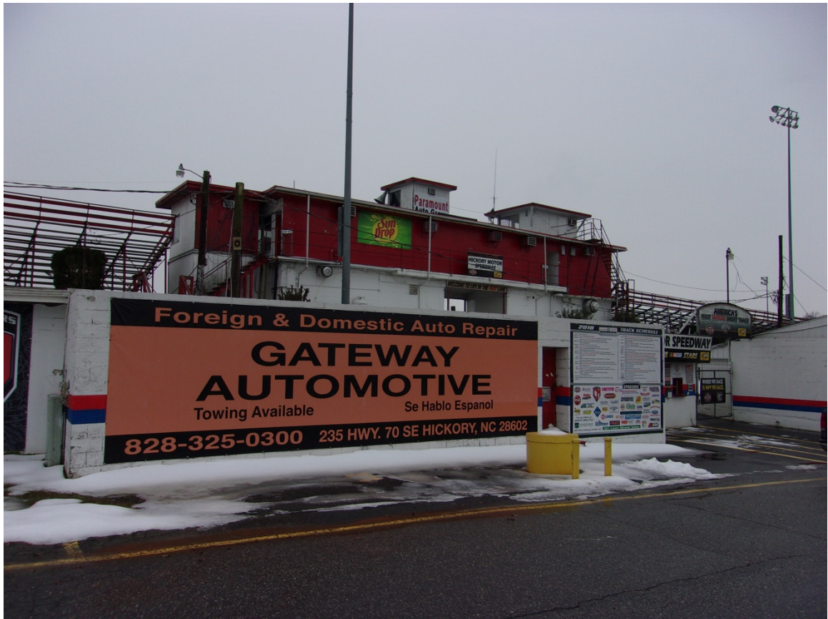
Figure 58. North elevation of ticket booth and storage area. Ticket booth is to the right next to the gate. (Photo Credit Author)
