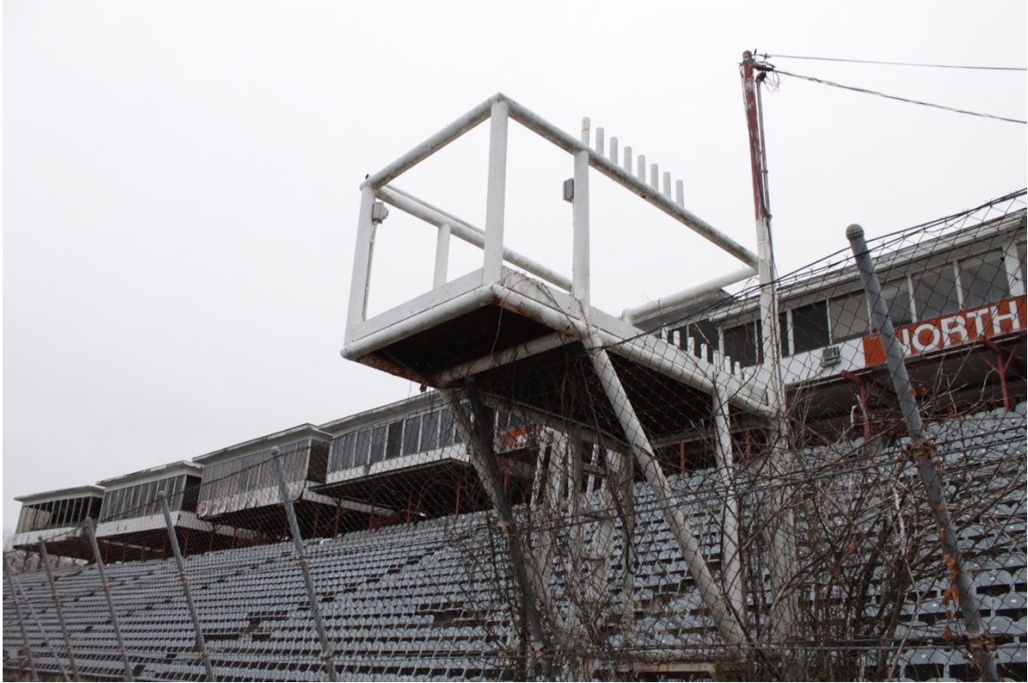
Figure 25. Metal flag stand located on the outside wall at the start/finish line. (Photo Credit Jacob Cook)
