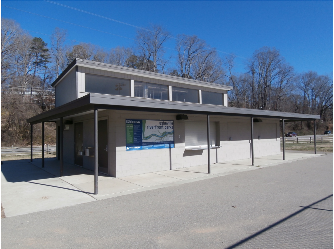
Figure 72. Building that served as the press box, concession stand, and restrooms, now concessions and restrooms for park visitors. (Photo Credit Author)
