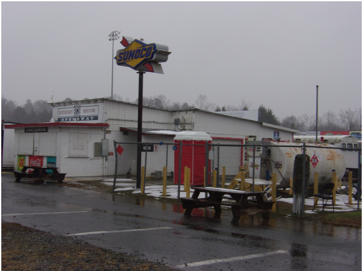
Figure 64. Infield concession stand with garage addition. (Photo Credit Author)
