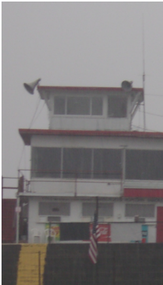
Figure 62. Original part of the media/control tower. (Photo Credit Author)
