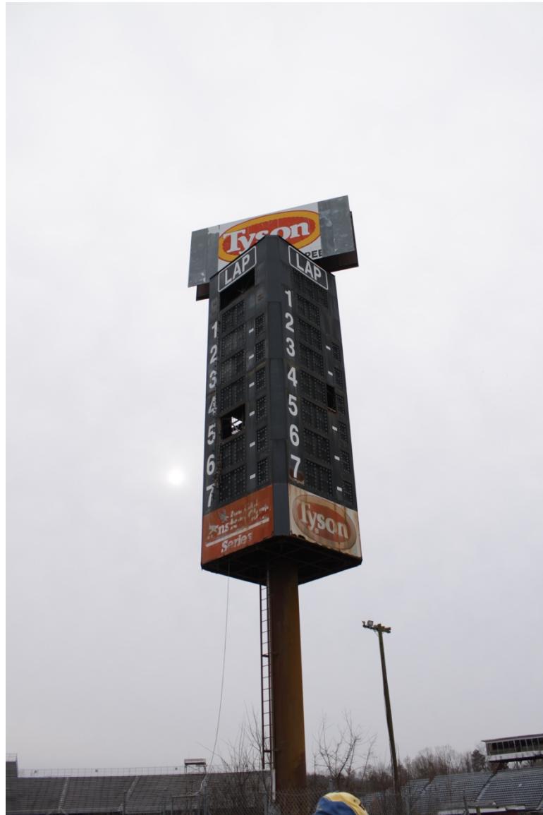
Figure 19. Scoring tower on infield no longer operational. (Photo Credit Jacob Cook)
