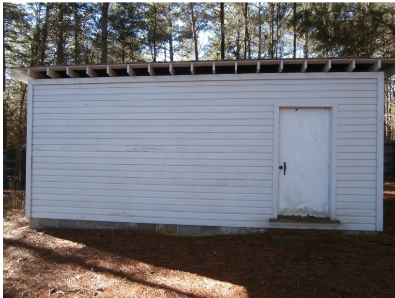
Figure 39. East elevation of women's restroom reconstruction. (Photo Credit Author)
