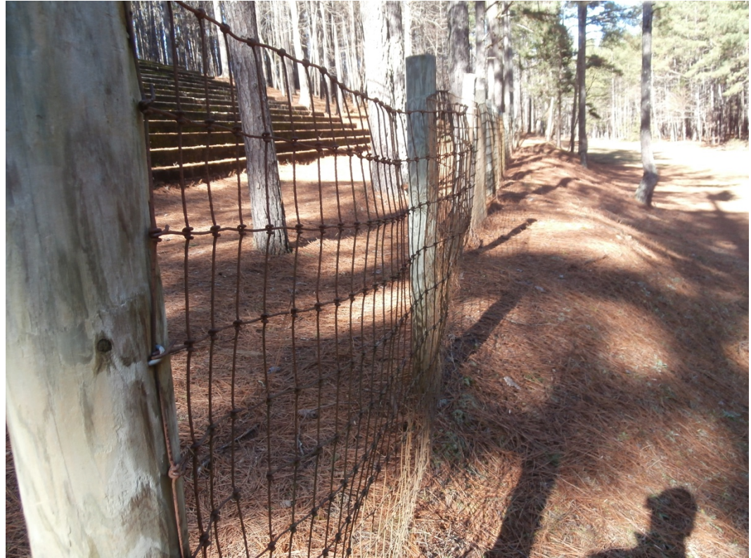
Figure 35. Woven wire fencing on front stretch, a rare sight at racetracks of today. (Photo Credit Author)
