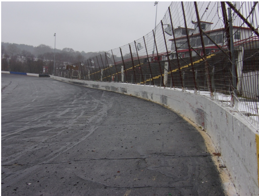
Figure 54. Outside concrete wall on front stretch with woven wire fence on top. (Photo Credit Author)
