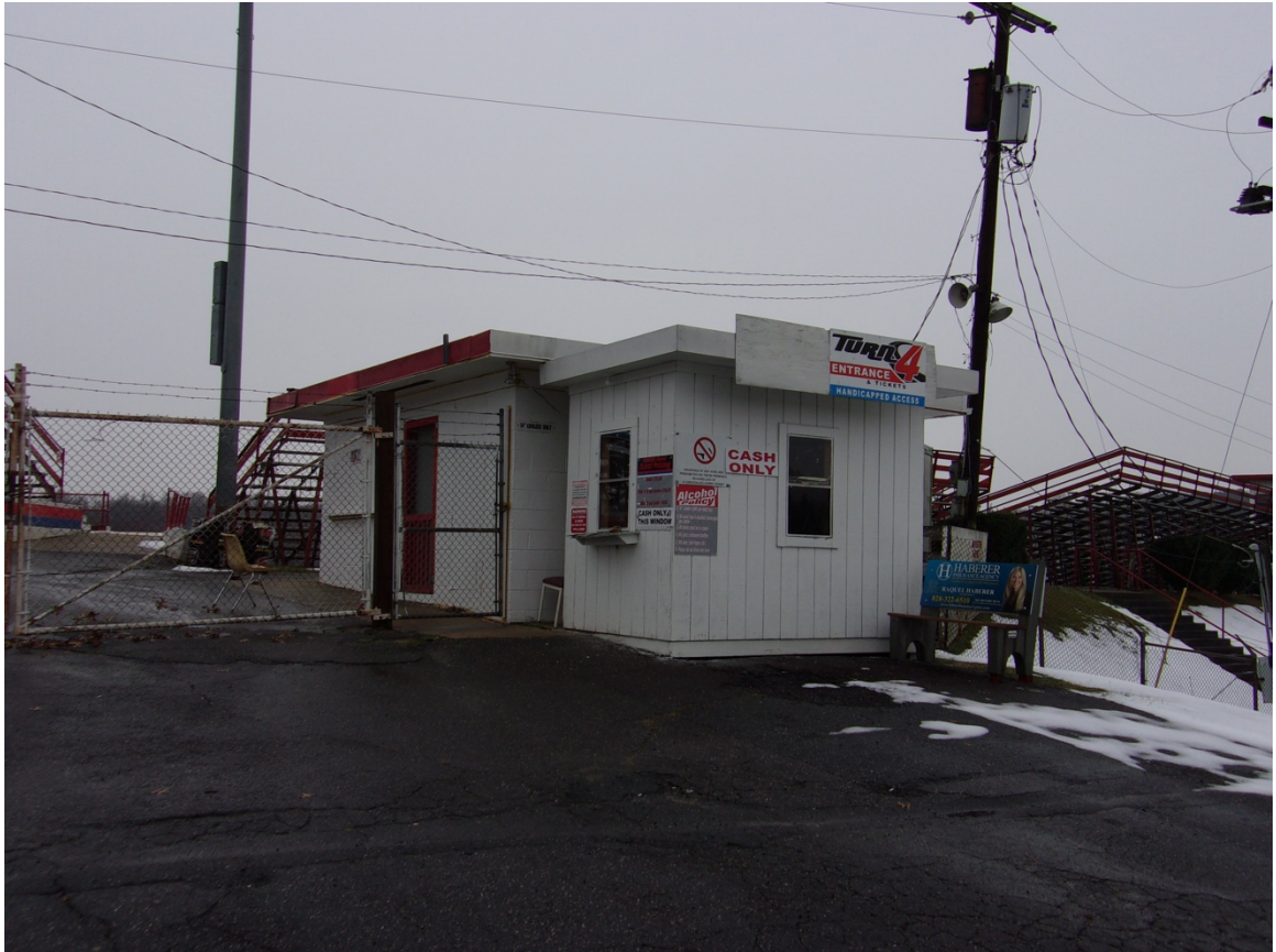
Figure 59. Concession stand in rear of ticket booth. Concession stand appears to be of similar construction to restrooms. (Photo Credit Author)
