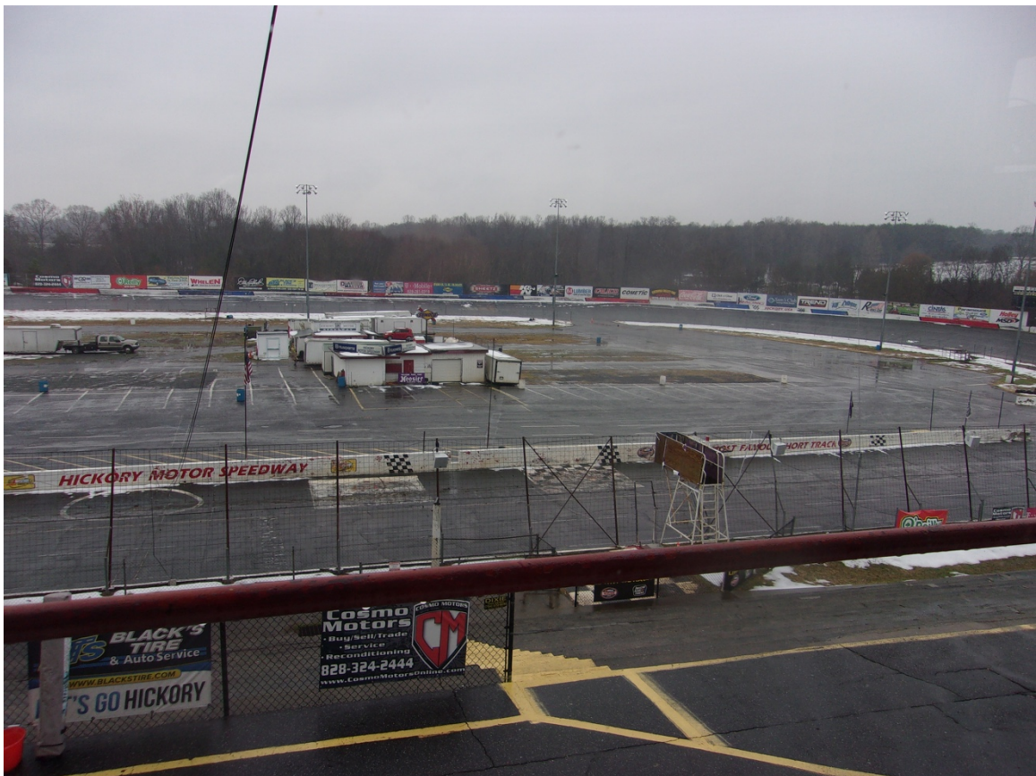
Figure 66. Overall view of buildings on the infield. (Photo Credit Author)
