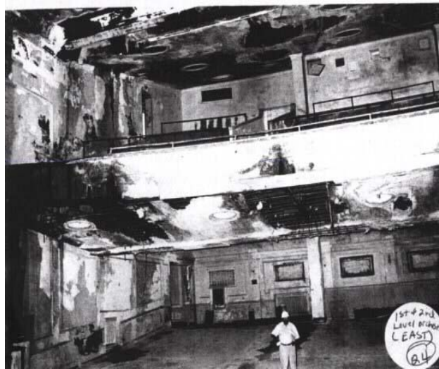
Fig. 27 Interior of the Albany Theatre, circa 1997. Photograph from the nomination form for the National Register of Historic Places.
