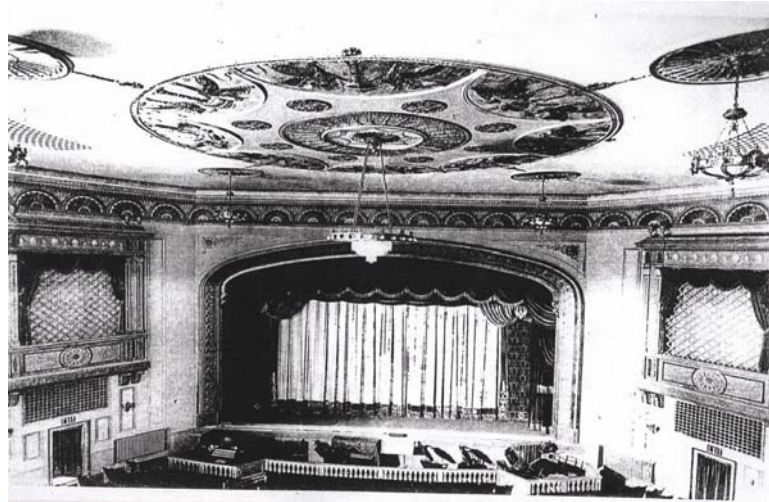
Fig. 25 Interior of the Albany Theater in 1927. Photograph from the nomination form for the National Register of Historic Places.
