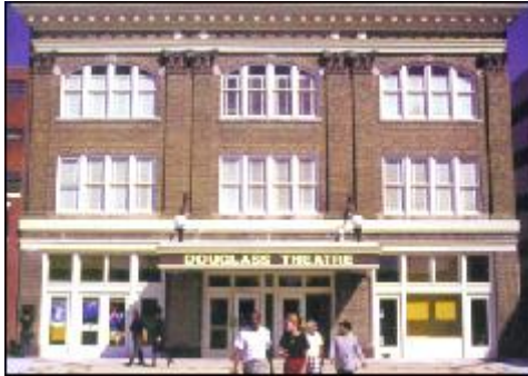
Fig. 16 The Douglass Theatre in Macon, Georgia. After restoration. Photograph from www.leftbankreview.com
