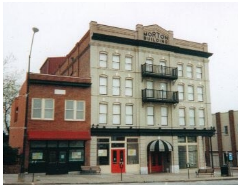
Fig. 4 The Morton Building in Athens, Georgia. After restoration. Photograph from www.morthontheatre.com
