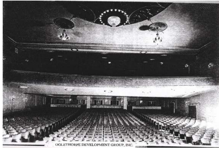
Fig. 24 Interior of the Albany Theatre in 1927. Photograph from nomination form for the National Register of Historic Places
