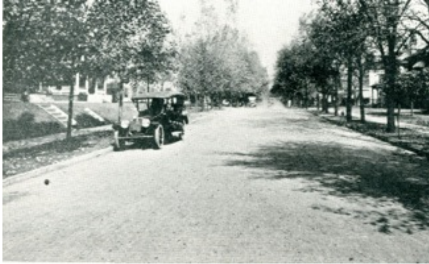
Figure 6: “Sand-Cushion Cement-Grouted Brick Pavement 28 Years Old.” 101
