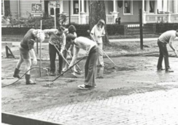
Figure 8: Residents of Wilmington, NC remove asphalt from a residential brick street, 1973. 149
