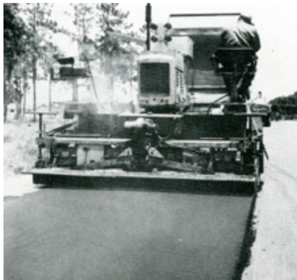
Figure 2: A man spreads asphalt mechanically. Using this method, 2,000 tons of asphalt pavement could be laid in an eight-hour day. 78
