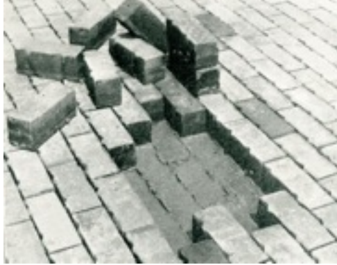
Figure 4: The construction of monolithic pavement as bricks are being laid into mortar 99
