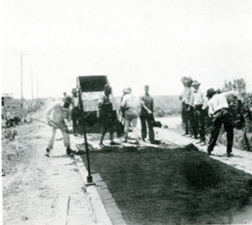
Figure 1: Men spread asphalt by hand. This method took ten men twelve hours to lay 300 tons of asphalt pavement. 77
