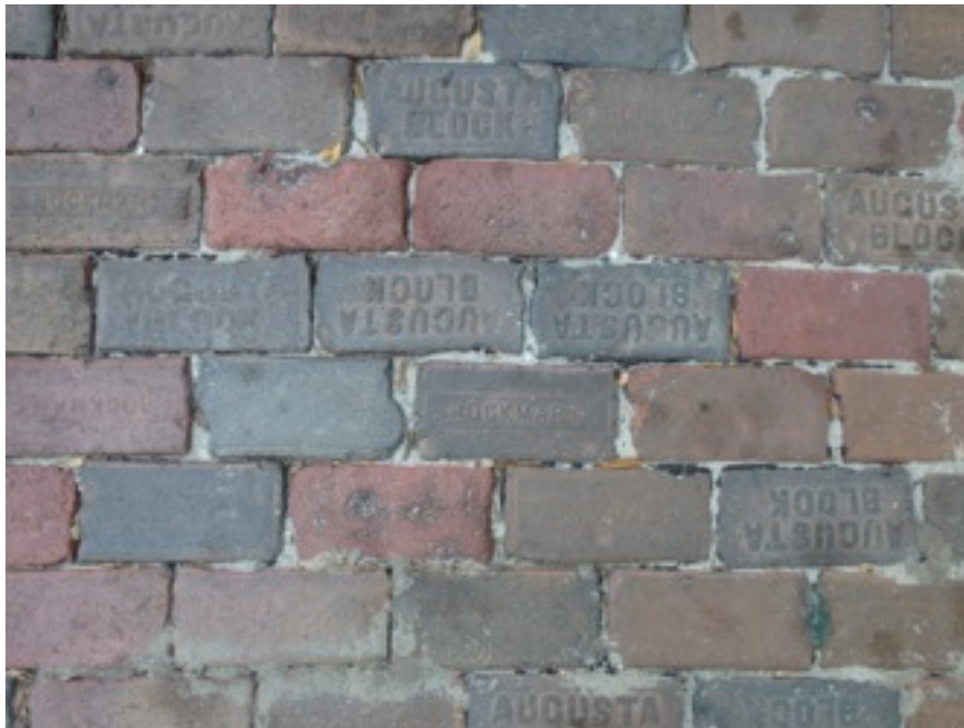
Figure 5: Brick pavement featuring sanded joints, Saint Petersburg, Florida. Photo by author.
