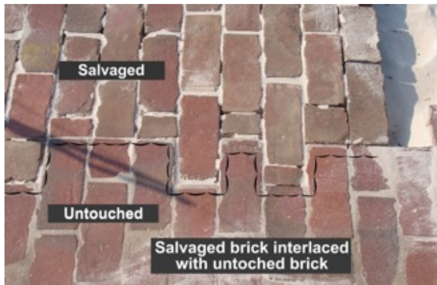
Figure 12: Patch showing the method of “weaving” replacement material into existing pavement 197
