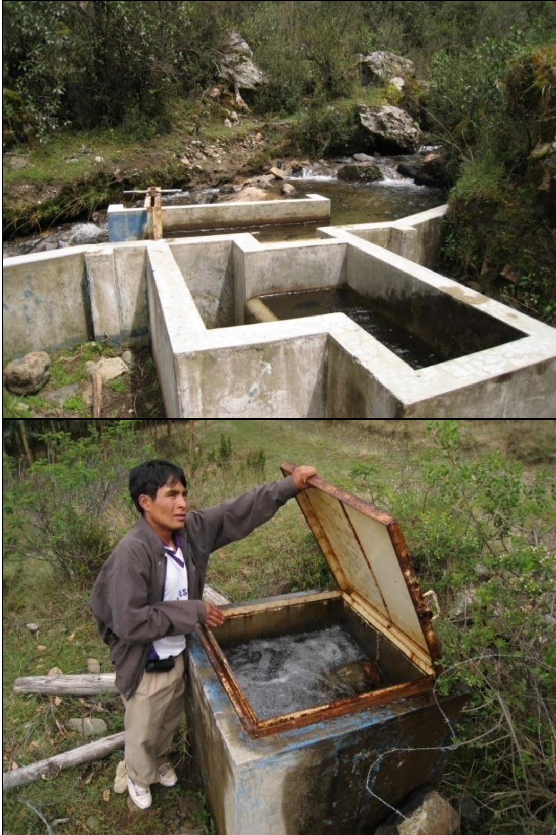
Figure 14 Marcará intake and pressure break system. Photographs by author.
