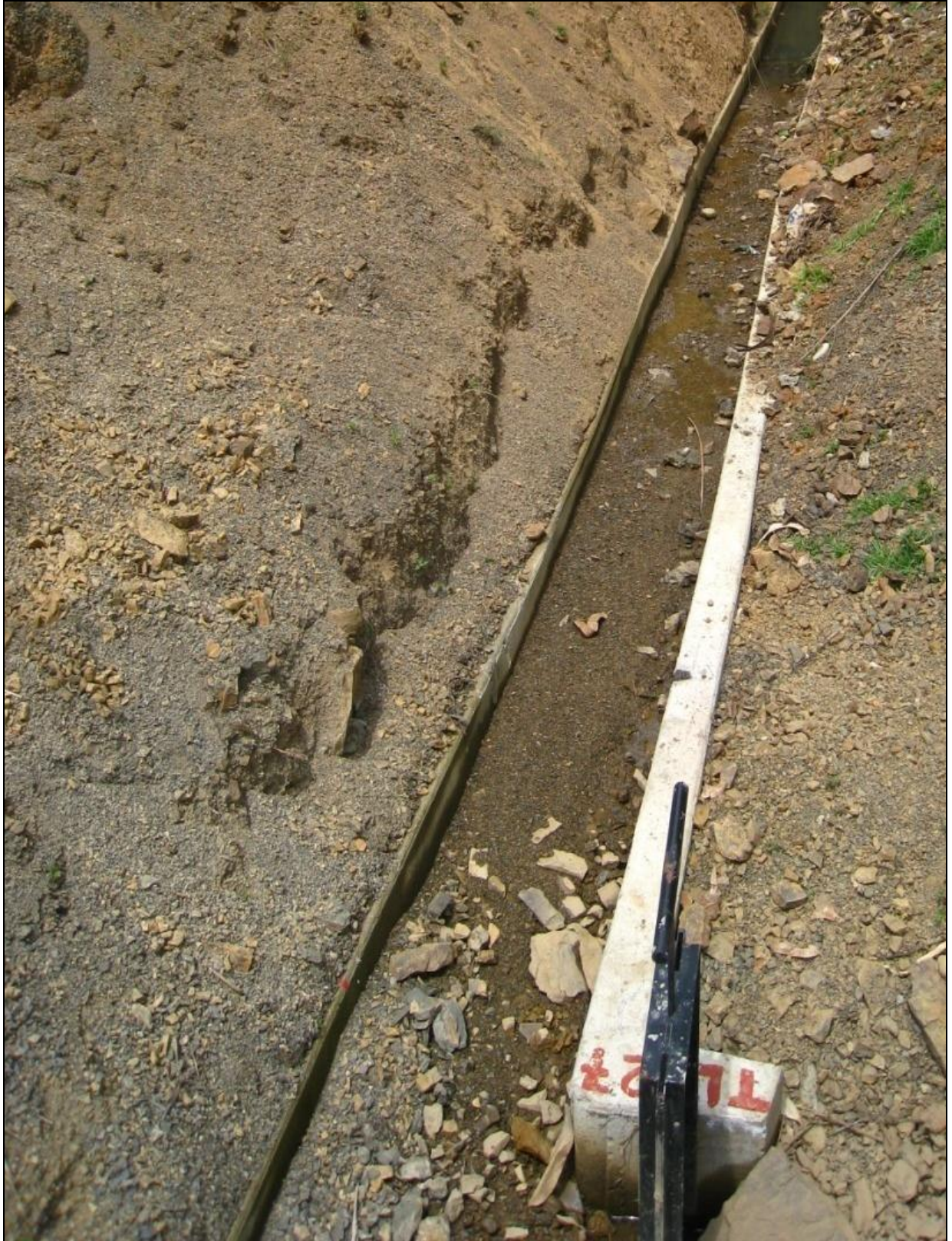
Figure 10 Metal diversion mechanism on concrete-lined canal. Photograph by author.
