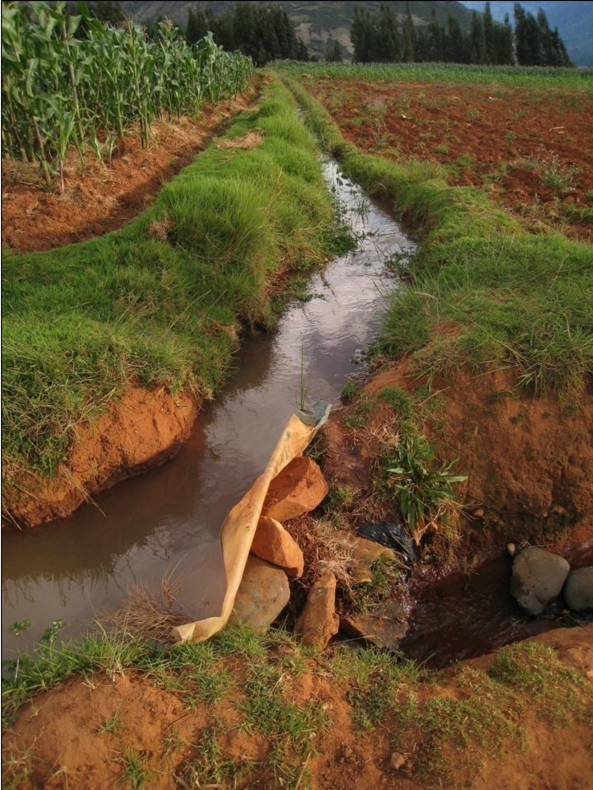
Figure 11 Example of makeshift diversion mechanisms on earthen canal. Photograph by author.
