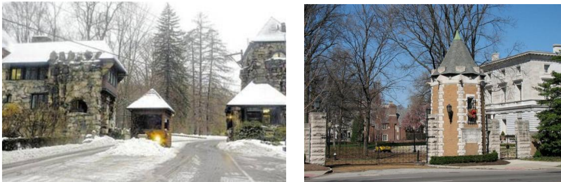
Figure 2-4: Tuxedo Park Gatehouse (left), St. Louis Gated Private Street (right). Sources: http://tuxedopark-ny.gov/ , http://www.thecwe.org/about-2/history/ .
