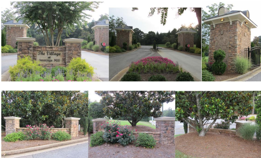
Figure 4-8: The Village gated entry design elements. Source: author photo.
