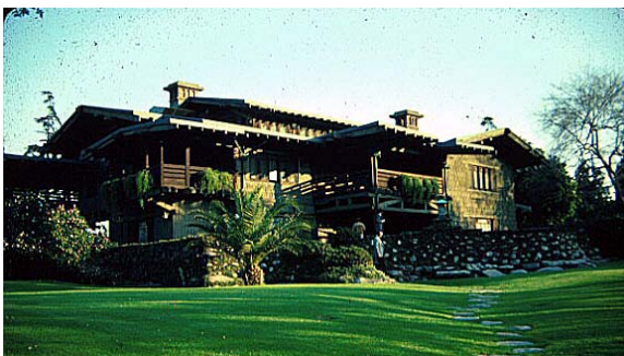
Figure 1 Gamble House, Pasadena, California
