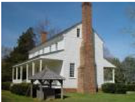
Figure 23: Alston House at House in the Horseshoe State Historic Site. 161
