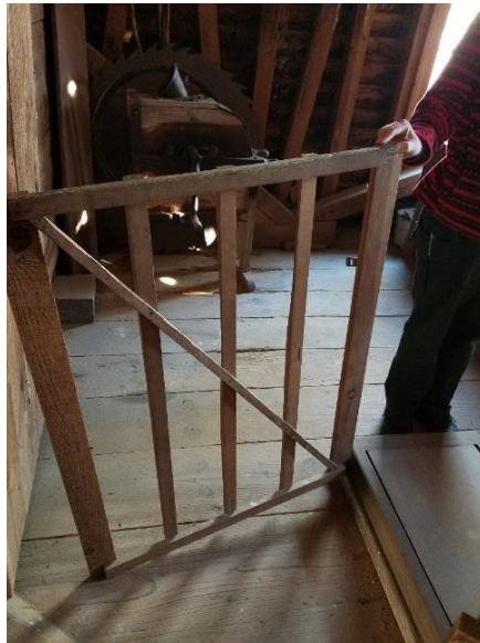
Figure 3.22: Jarrell Plantation- This is a Separation Gate placed in the doorways of each structure to control visitor traffic. (Author's Photo)
