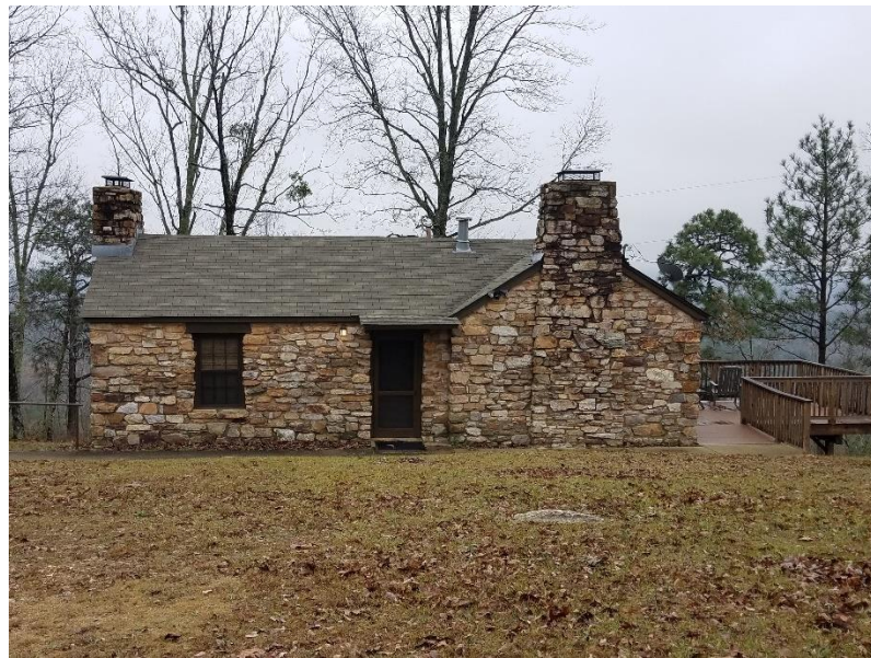
Figure 3.24 F.D. Roosevelt State Park- This is a CCC constructed cabin. It is constructed from local stones, and asphalt shingles. A chimney is visible on each end of the cabin for each of the rooms within the cabin. (Author's Photo.)
