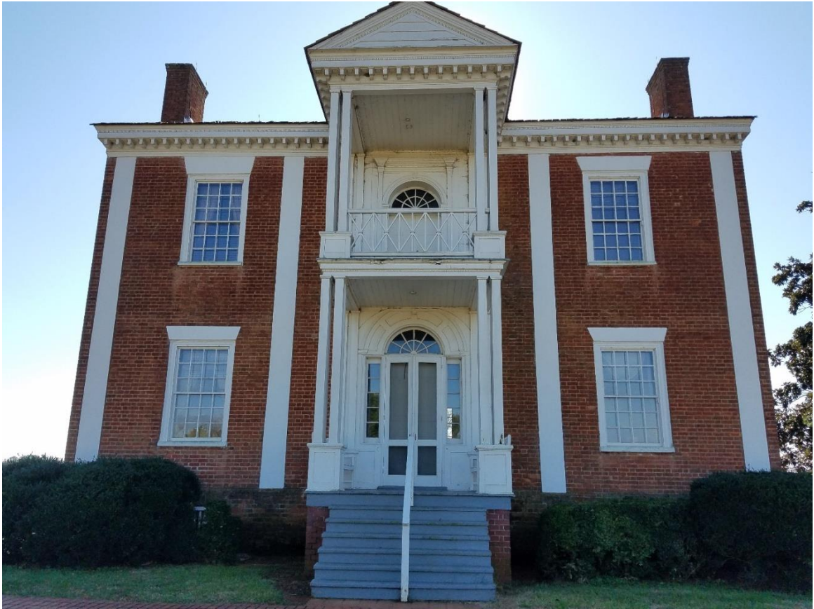
Figure 3.5: Chief Vann House-Front Exterior of the north elevation. The structure is a 2-story brick federal style building. Note the 3-bay design, the 9 over 9 double hung windows, the central entry on the first floor with fan and sidelights, as well as a 2nd story porch with pediment (Author's photo.)
