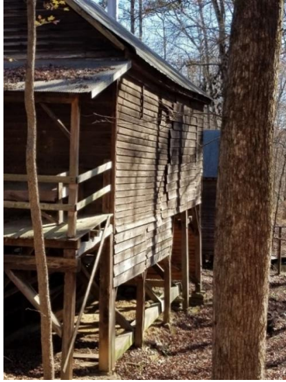
Figure 3.21: Jarrell Plantation- inferior repair work is obviously apparent in this image. The clapboards were not cut so that they would be flush with the rest of the clapboards on the structure and as a result present a visibly poor repair job. (Author's Photo)
