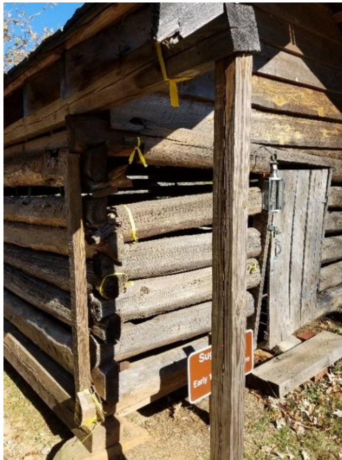
Figure 3.11: C.V.H. exterior cabin. Visible here is a structural issue where a supporting beam inside of the cabin was removed without proper consideration and as a result the wooden log twisted under the pressure cracking and separating from the corner joints causing additional damage around the door frame. (Author's Photo)
