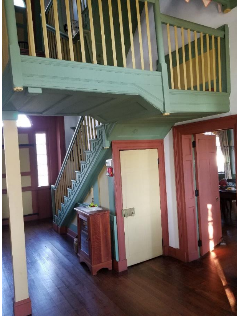
Figure 3.10: Chief Vann House- Cantilevered Stair featuring the wooden post added to support the landing to prevent further damaging stress to the structure and possible collapse. Also visible is the later addition of the basement entrance beneath the stair. (Author's Photo).
