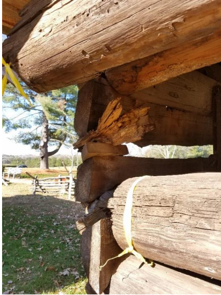
Figure 3.12 C.V.H. exterior cabin, Visible here is the point where the wooden log cracked from the pressure of the lost internal structural support and separated from the corner joint. (Author's Photo)
