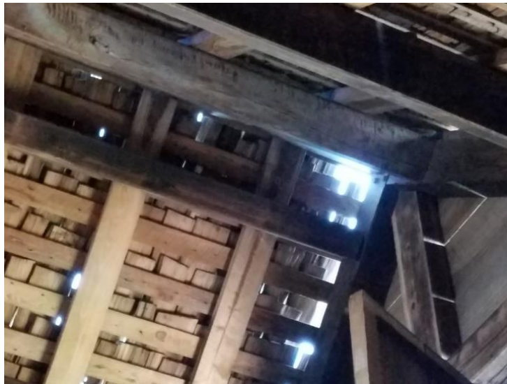
Figure 3.15 Fort King George- This image illustrates the loss of cedar shingles on the Blockhouse roof. The continued absence of these shingles leads to more water damage inside the cultural resource. (Author's Photo)
