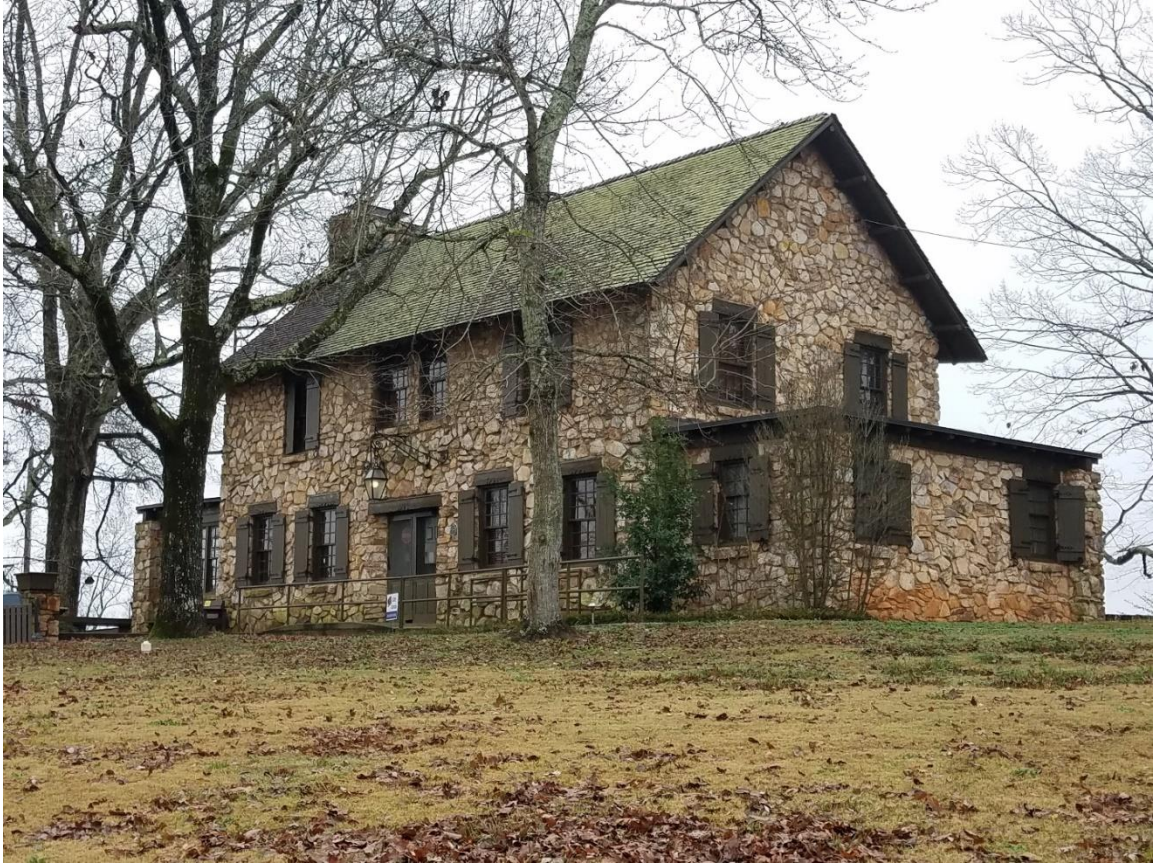
Figure 3.23: F.D. Roosevelt. – This is the Main office of the park and it represents the type of CCC construction that can be found on numerous cultural resources throughout the park. (Author's Photo)
