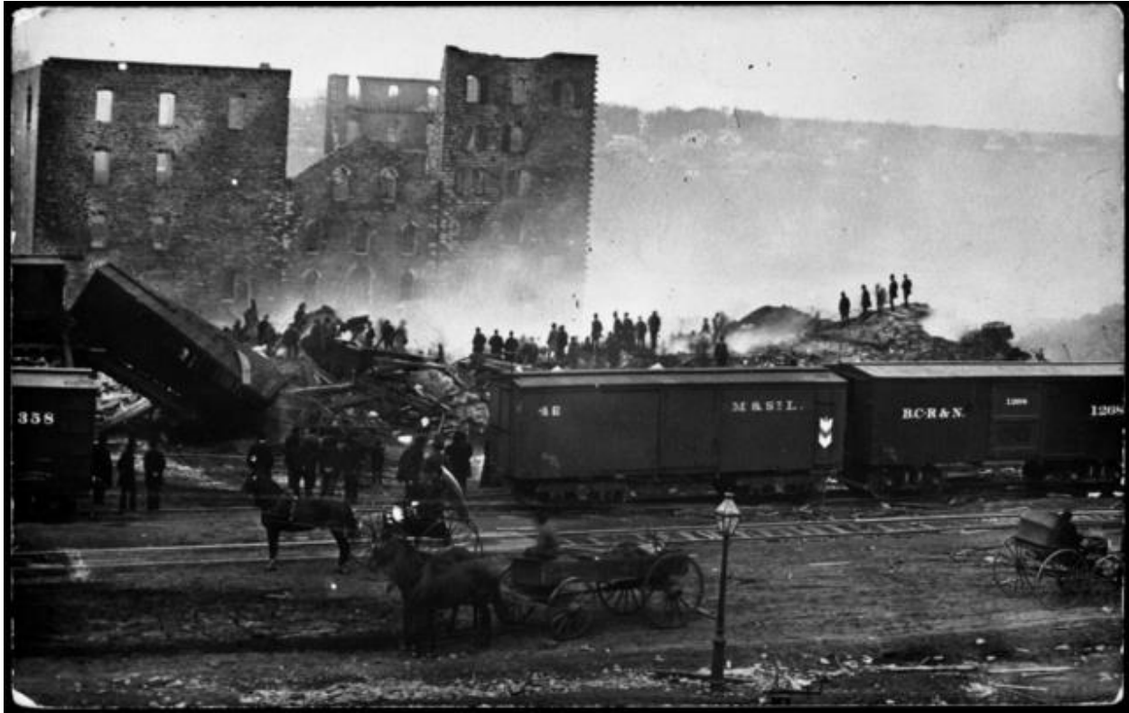
Figure 4.5: Washburn A Mill following the 1878 explosion. (Source: Minnesota Historical Society, Minneapolis Minnesota)
