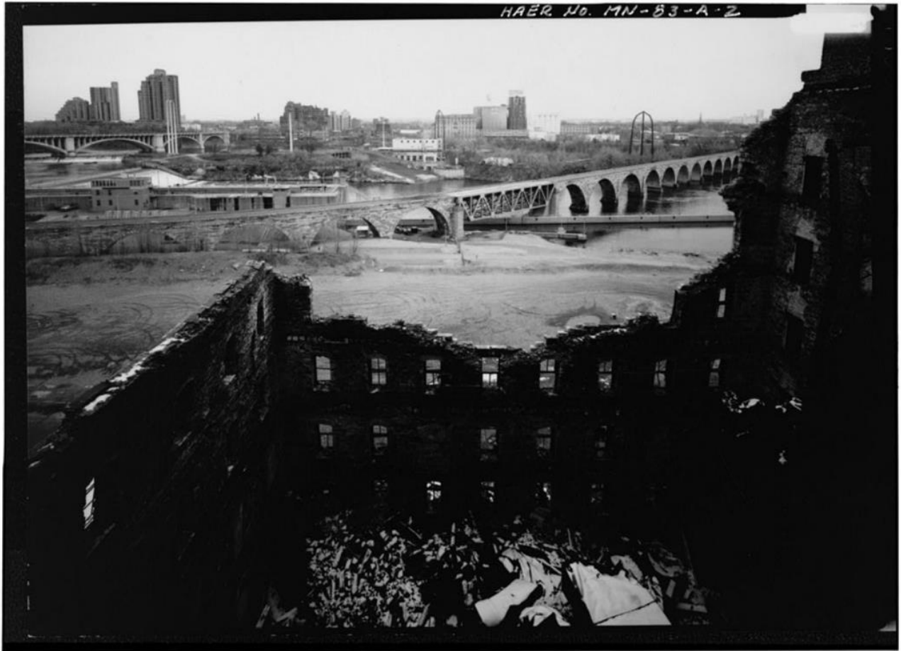
Figure 4.7: Washburn A Mill, view of northeast interior wall and debris from the 1991 fire, facing the Mississippi River and Stone Arch Bridge. (Source: Historic American Engineering Record, Minneapolis, Minnesota)
