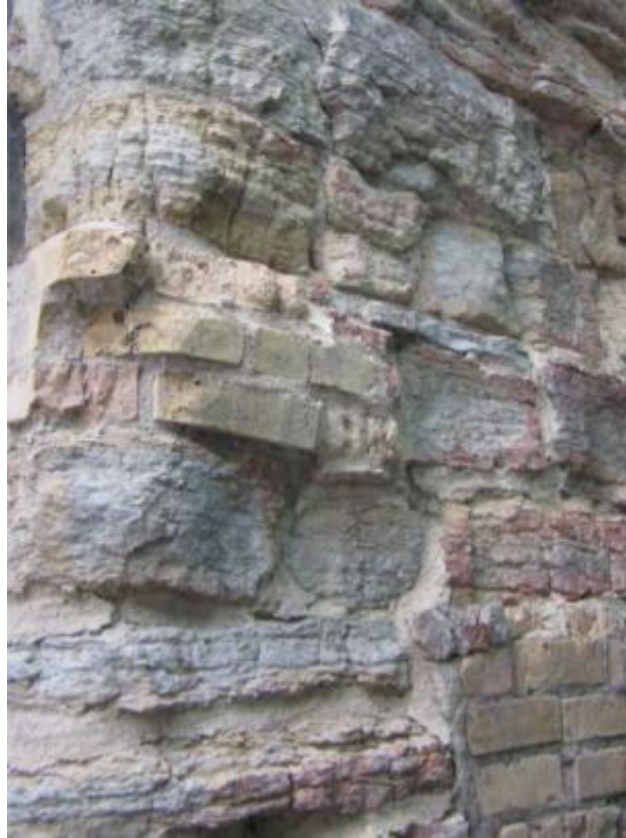
Figure 4.8: Photograph showing the combination of Platteville limestone and brick used on the ruin courtyard walls. (Source: MacDonald & Mack Architects, Minneapolis, Minnesota, 2016)
