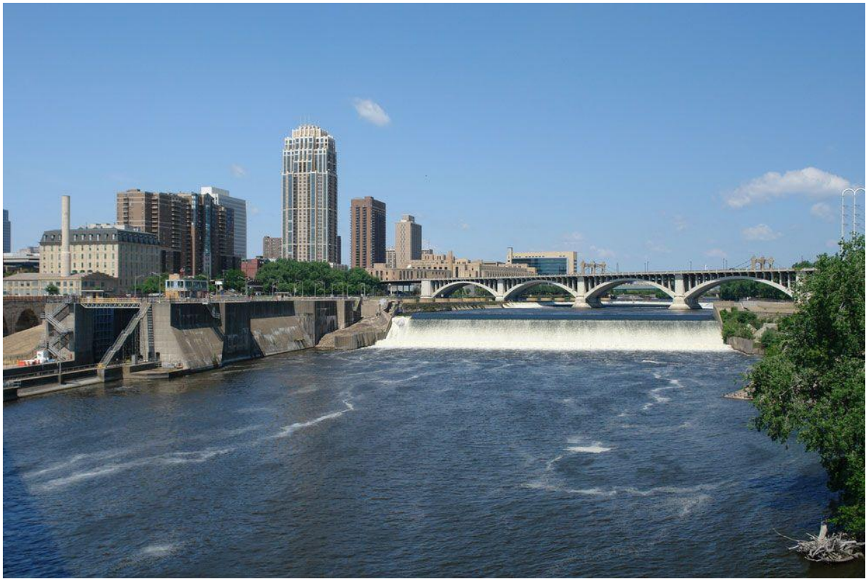
Figure 3.6: Spillway at St. Anthony Falls. (Source: Matt Hickman, Mother Nature Network)
