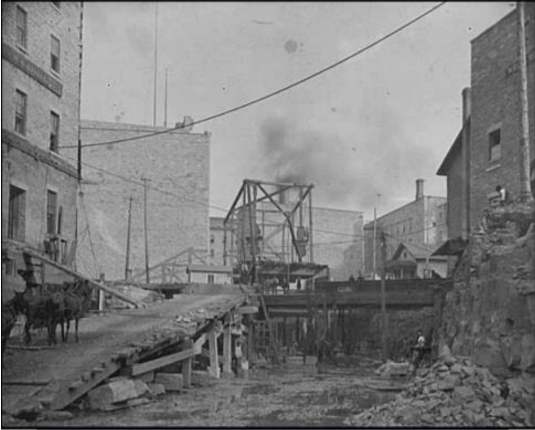
Figure 5.2: Working on the West Side canal at St. Anthony Falls, c. 1885. ( Source: Minnesota Historical Society, Online Collection)
