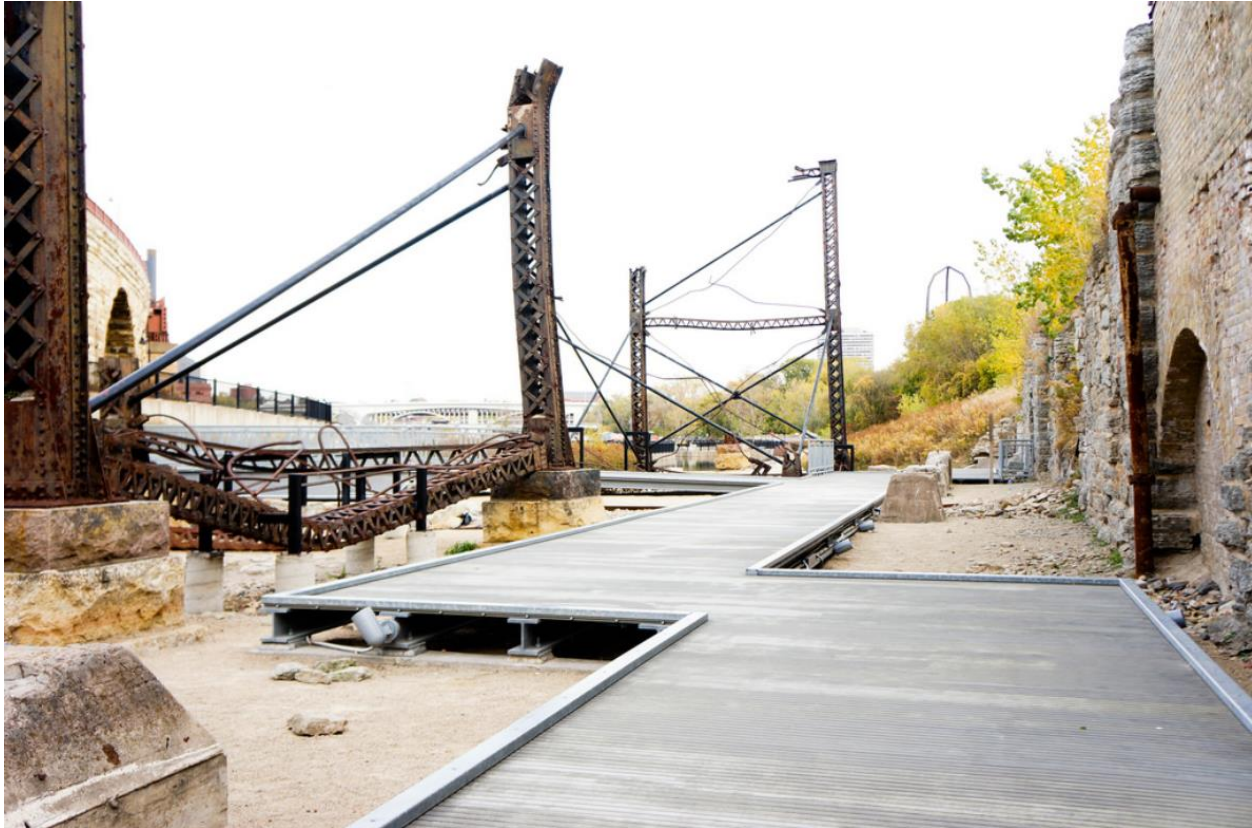
Figure 5.8: Photograph of walking paths and stabilization bracing at Mill Ruins Park. (Source: Landscape Voice, October 11, 2012. http://landscapevoice.com/mill-ruins-park/ )
