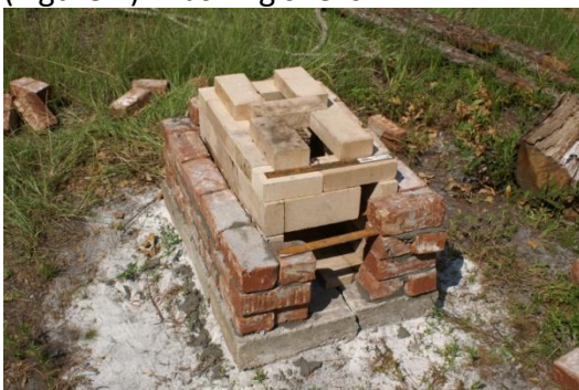
(Figure 3)-Kiln under construction
