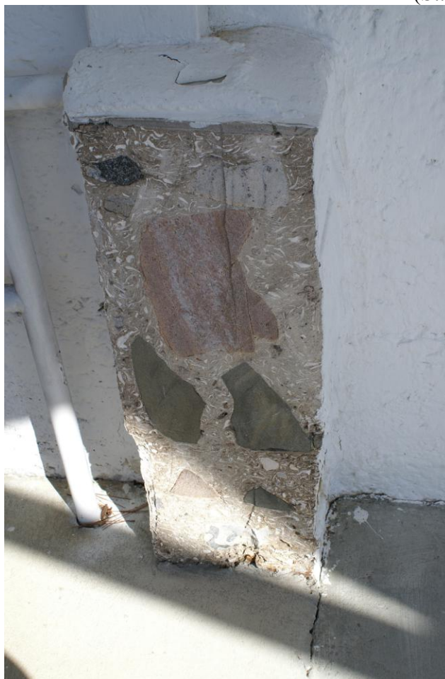
(Cross-section of wall showing tabby and ballast stone)
