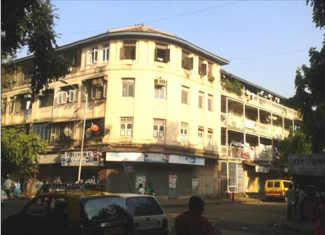
Figure 4.2: A chawl building with shops on the ground floor, facing the main road.
