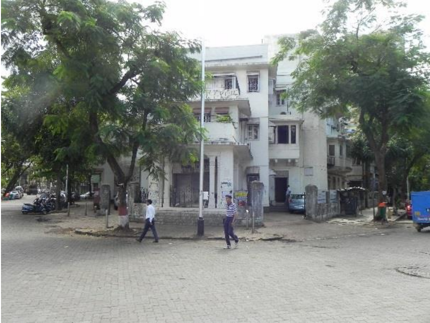
4.23: Front façade of Modak Bungalow
