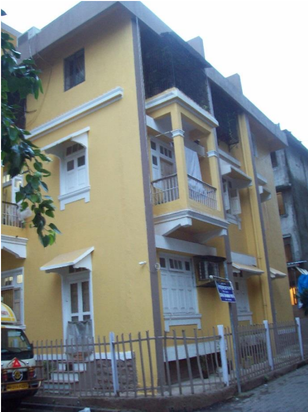
Figure 6.1: Vernacular bungalow residence along Shivsena Bhavan Path. Built in 1935, a unique blend of vernacular and European typology.
