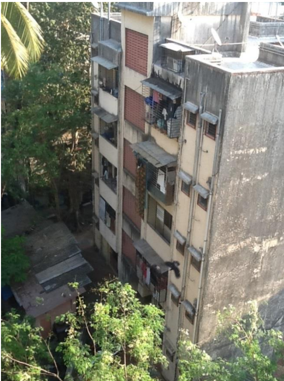
Figure 4.9: Recent development encroaching on wadi.
