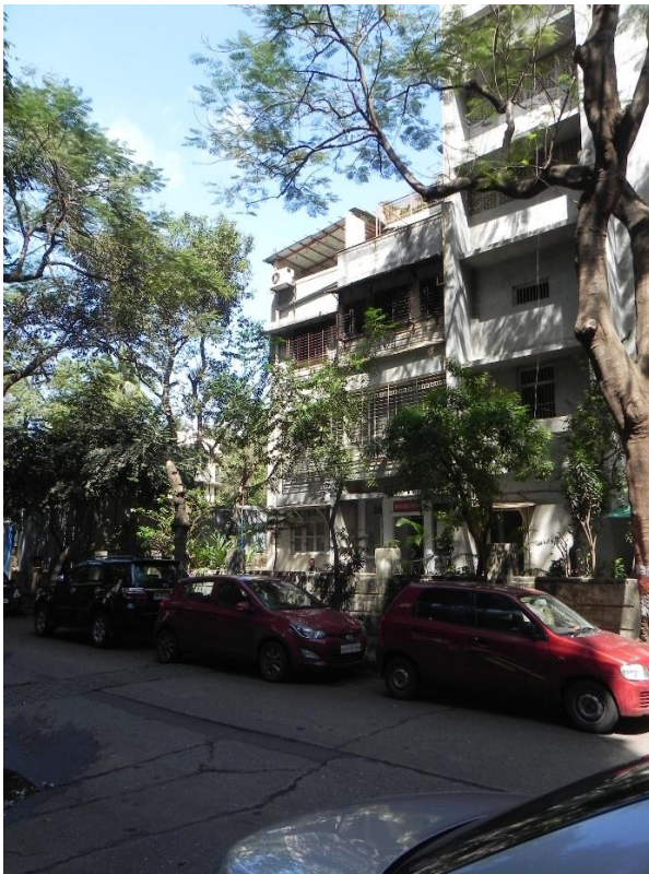
4.22: Building façade of Savarkar Sadan. Structure built in 1938, has been subjected to additions.
