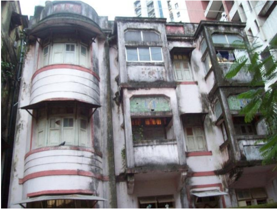
Fig 6.4: Art Deco-inspired vernacular apartment building. Located along Shivsena Bhavan Path.
