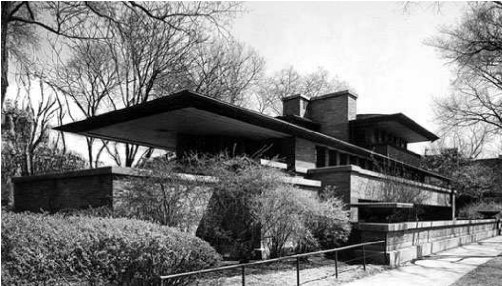
Figure 1: The Robie House, Frank Lloyd Wright, Chicago, Illinois
