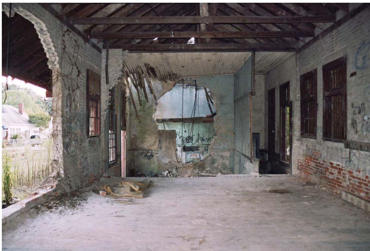
Figure 5.90: October 5, 2005. Pelzer interior, south view.
