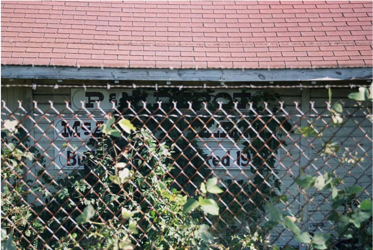
Figure 5.77: October 15, 2005. Like moss on a tombstone, the kudzu is reclaiming for the earth this sign left for posterity. Although the construction date is obscured, the right side of the bottom line may read, “Altered 1978.”
