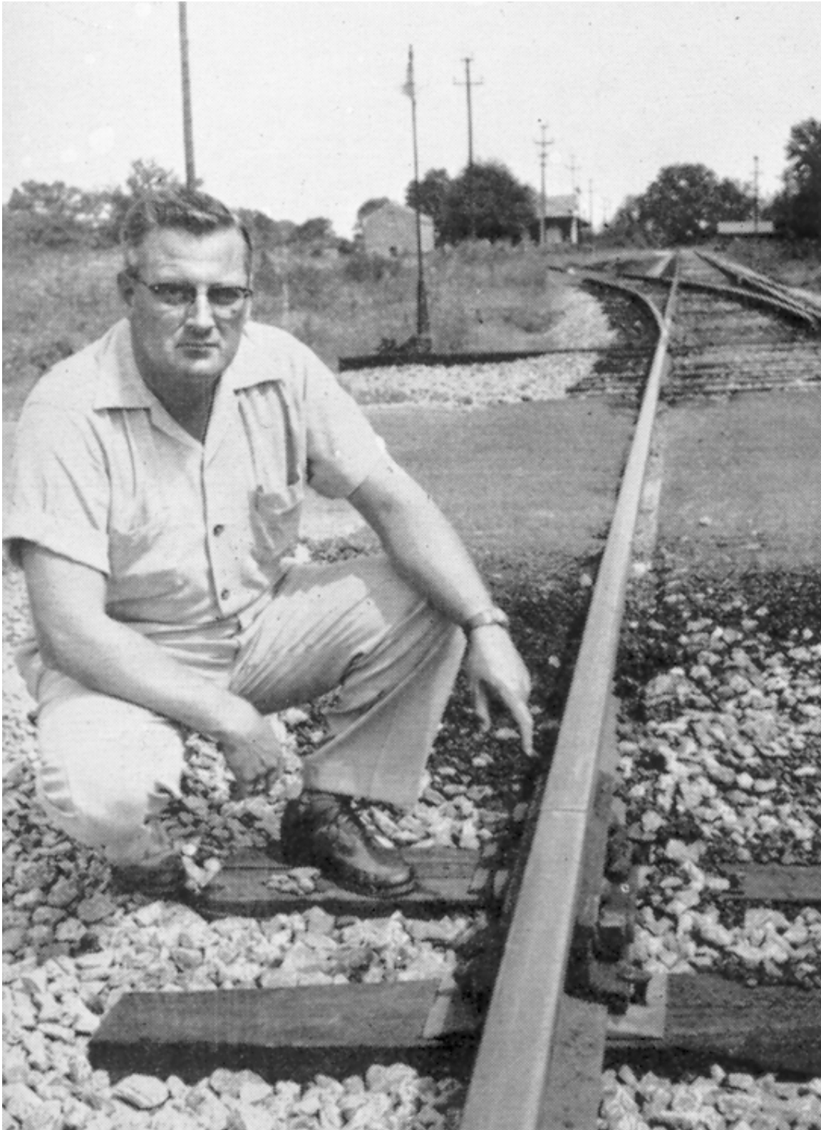
Figure 5.131: Williamston agent John Barr points to a joint in the rail in the September, 1956, issue of Semaphore . Behind the switchstand over his left shoulder are two buildings which appear to be an electrical substation and the Williamston depot. Unlike the previous photo (Figure 5.130), the building in this image appears to be one of C.C. Hook's single-story plans.
