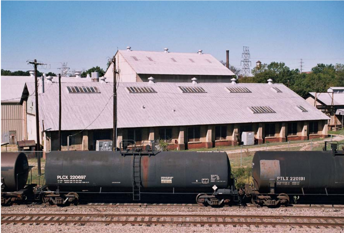
Figure 5.106: October 20, 2005. The P&N's "River Junction" shops in Greenville, South Carolina. The building immediately behind the tank cars is the original shop building; note that it matches Hook's stations in color, material, and to some extent in details. Windows are paired much as they are in the stations.
