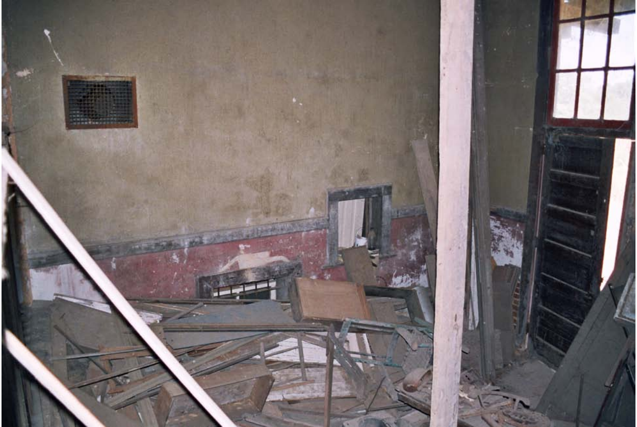
Figure 5.37: Interior, freight office (or segregated waiting room), Donalds. The small window in the wall, center, communicates with the stationmaster's office. This space was originally separated from the warehouse (from which the photograph was made) by a non-load-bearing brick partition wall, which collapsed during the Johnsons' early work on the building.
