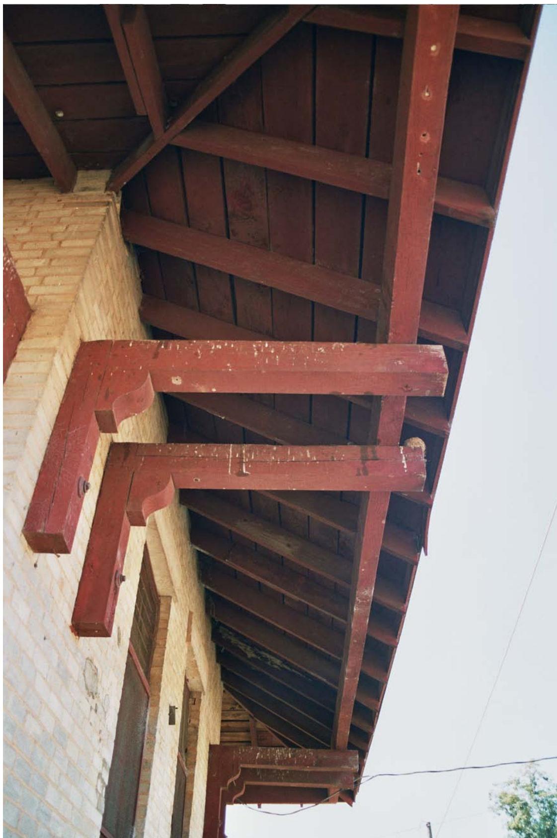
Figure 5.33: October 5, 2005. Detail of eave overhang and cornice brackets, Donalds.
