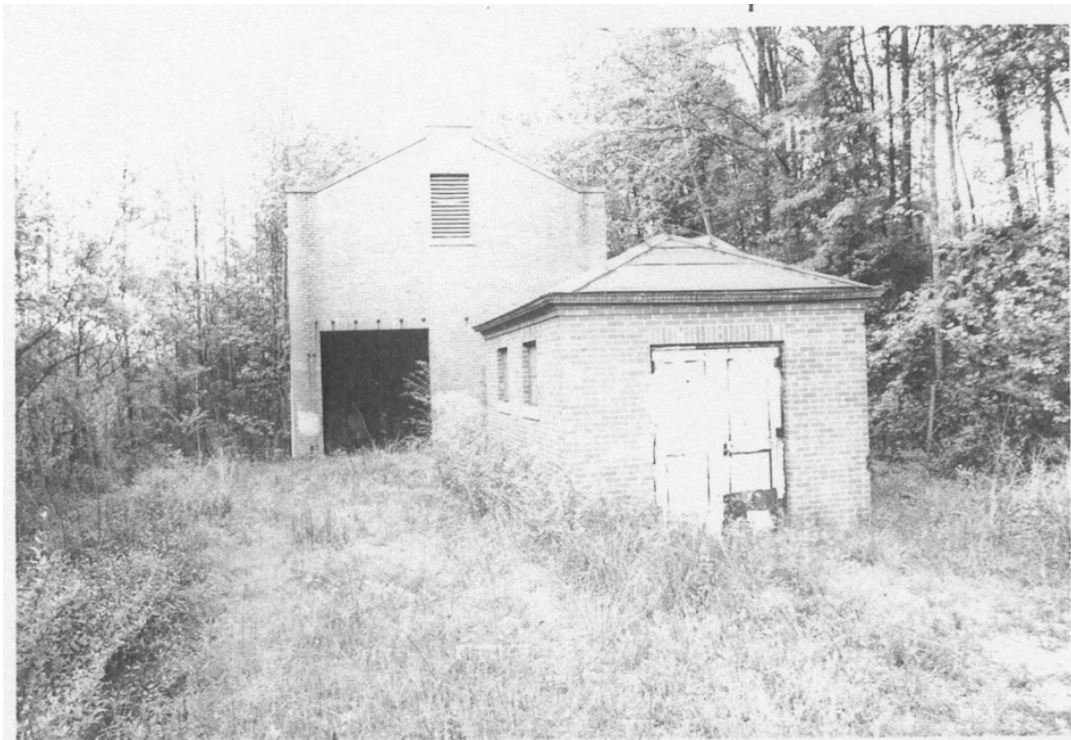
Figure 5.120: The Taylors electrical substation. The P&N used roughly a dozen such substations to feed its overhead catenary wires. Photo courtesy of Thomas Fetters.
