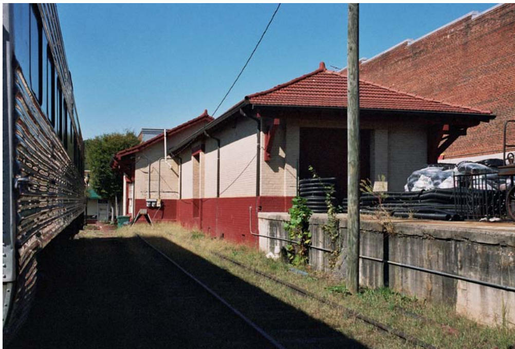
Figure 5.12: October 15, 2005. The freight section. It appears that Belmont was built without a trackside platform; note that the roof overhang of the freight warehouse is much shallower to accommodate the “spotting” of freight cars in front of the freight door. A ramp (not shown) leads up to the deck of the concrete platform nearest the camera, and another unusual feature is the presence of a freight door – which appears original – in the end of the freight house. One reason for these departures from the “standard” layout of P&N stations may be the limited physical space around the station. Originally the P&N tracks continued across Main Street (at left) and joined the main line of the Southern Railway within a matter of yards. For the P&N, Belmont was located at the end of an approximately four-mile long branch, and there may have been no room for additional tracks at the station.
