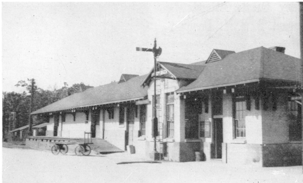
Figure 5.127: As yet, the only photo found of the Tucapau station. Like Piedmont, it has two freight doors (instead of the more common single platform door). The distinguished Westinghouse semaphore is set to “STOP.” Although this photo is the only evidence, it appears that the building was located at the diamond where the Southern Railway crossed the P&N. Both roads used a short branch that ran down into the Startex Mill. Photo appeared in the January, 1948, issue of Semaphore .
