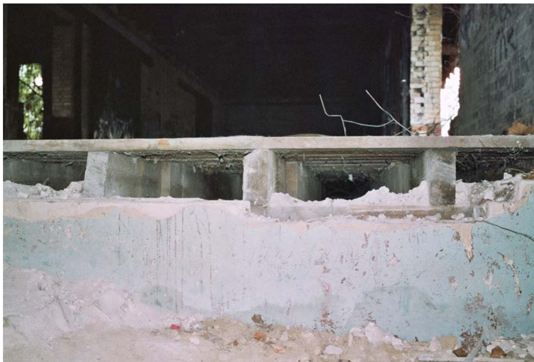
Figure 5.92: October 5, 2005. A collapsed interior wall shows the raised floor and heavy joists of the freight room.
