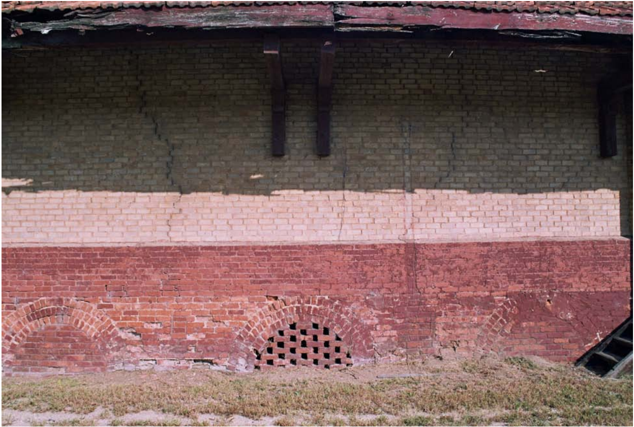
Figure 5.100: October 5, 2005. The west wall shows signs of structural failure, most significantly in the form of cracks such as these which run from ground to top sill.
