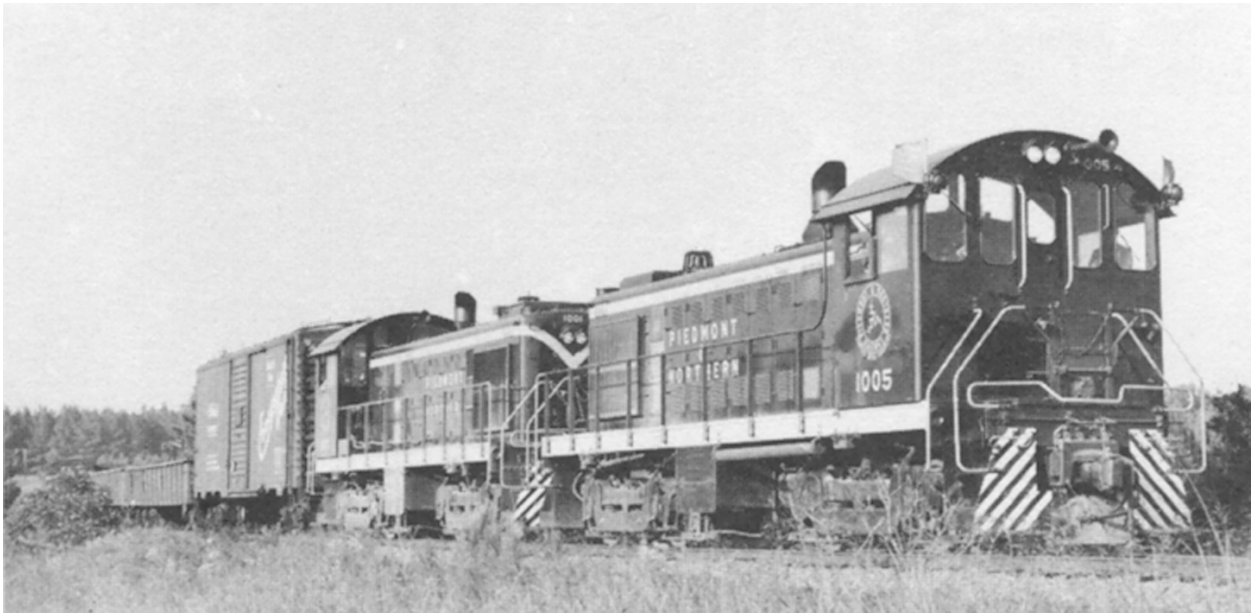
Figure 2.17: It may look as if S4s 1005 and 1001 are running backwards as they trundle through the red clay country of North Carolina, but in fact the P&N often operated these units this way. The improvement in visibility for the crew was tremendous and much more like they were used to seeing after operating electric locomotives for so many years. Fetters and Swanson, p. 133.
