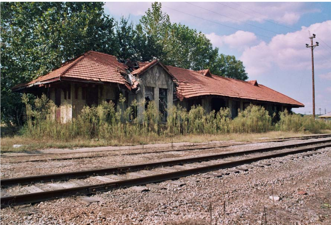
Figure 5.88: October 5, 2005. The Pelzer station today – crumbling, overgrown, and vandalized.
