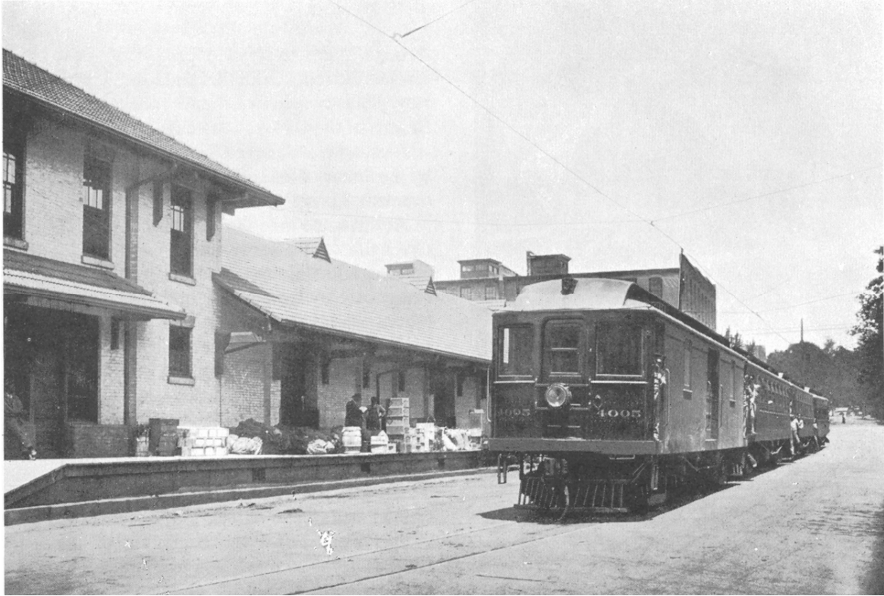
Figure 5.45: The platform on the Academy Street side of the Greenville freight station appears to have been very busy the day this picture was taken. Photo courtesy of Thomas Fetters.
