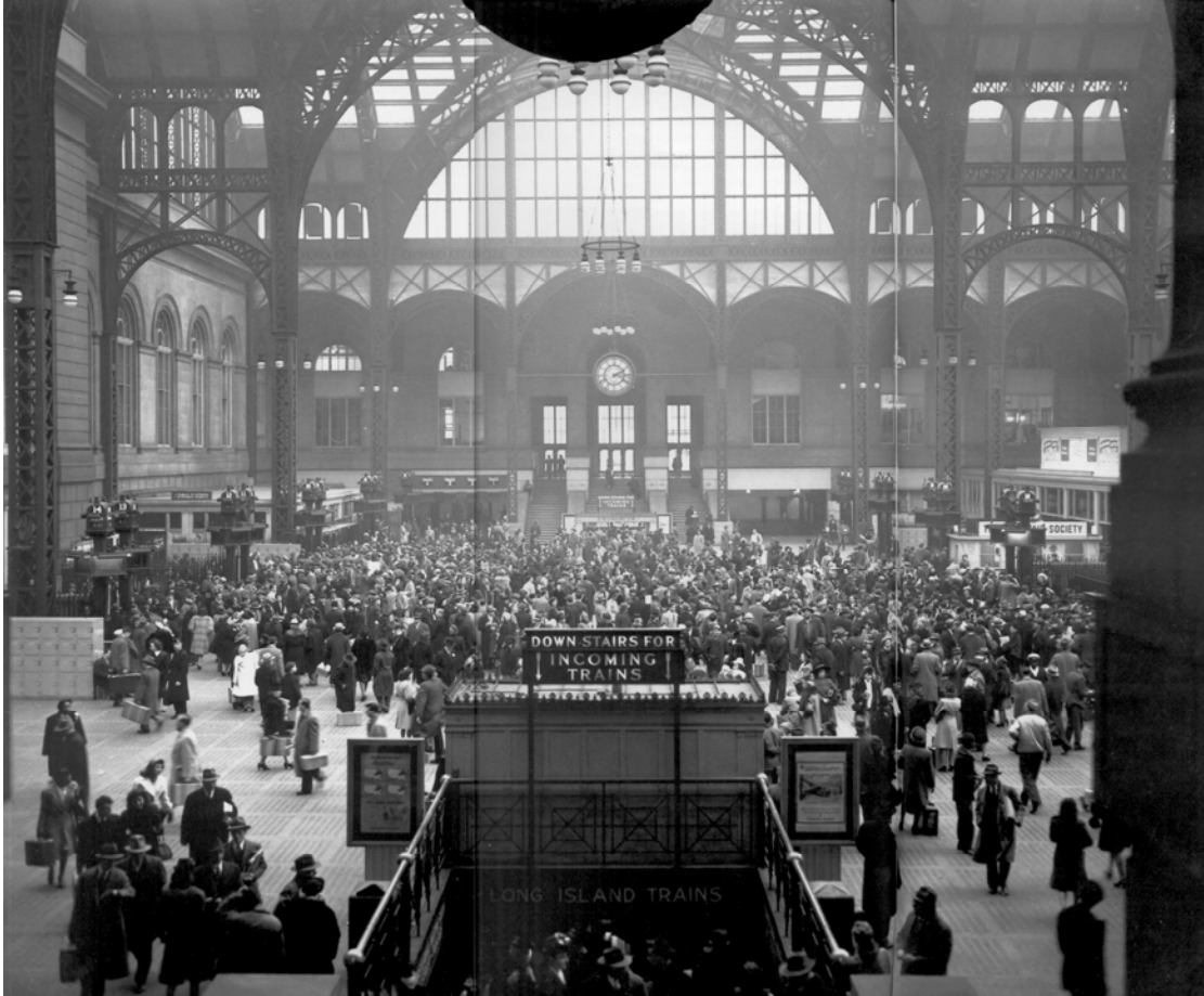
Figure 1.59 (Solomon, pp. 100-101): Penn Station's main concourse, looking along the centerline of the building toward the Eighth Avenue entrance.
