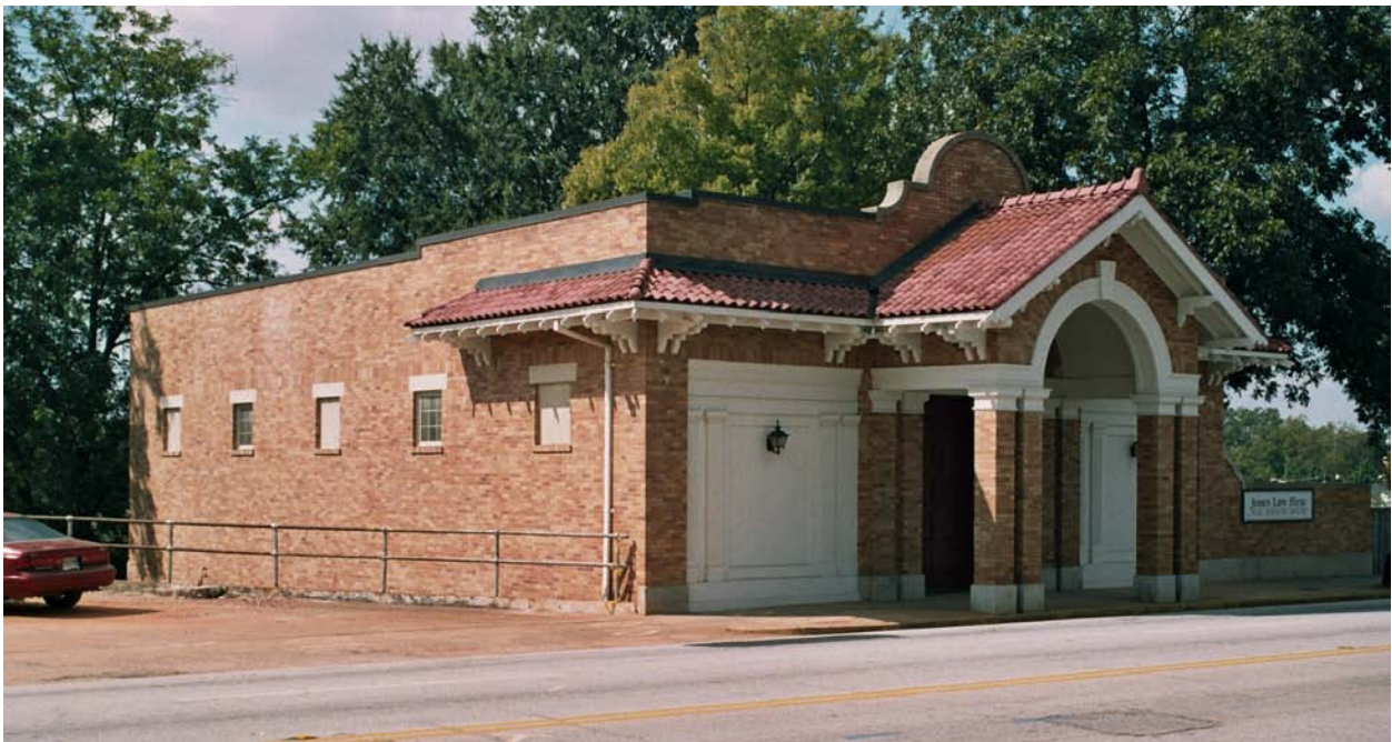
Figure 1.56 (Author's photo): The Piedmont and Northern Railway passenger station at Anderson, S.C., notable for its large arched Main Street entrance.
