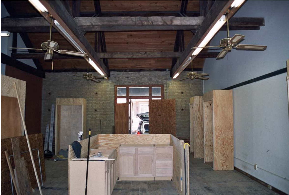
Figure 5.53: October 20, 2005. Interior of what is becoming a boutique; the freight section has been subdivided longitudinally by what appear to be simple wood frame partition walls, but much of the building's original material is intact; for instance, the floors, which have had spot repairs made but are largely original.
