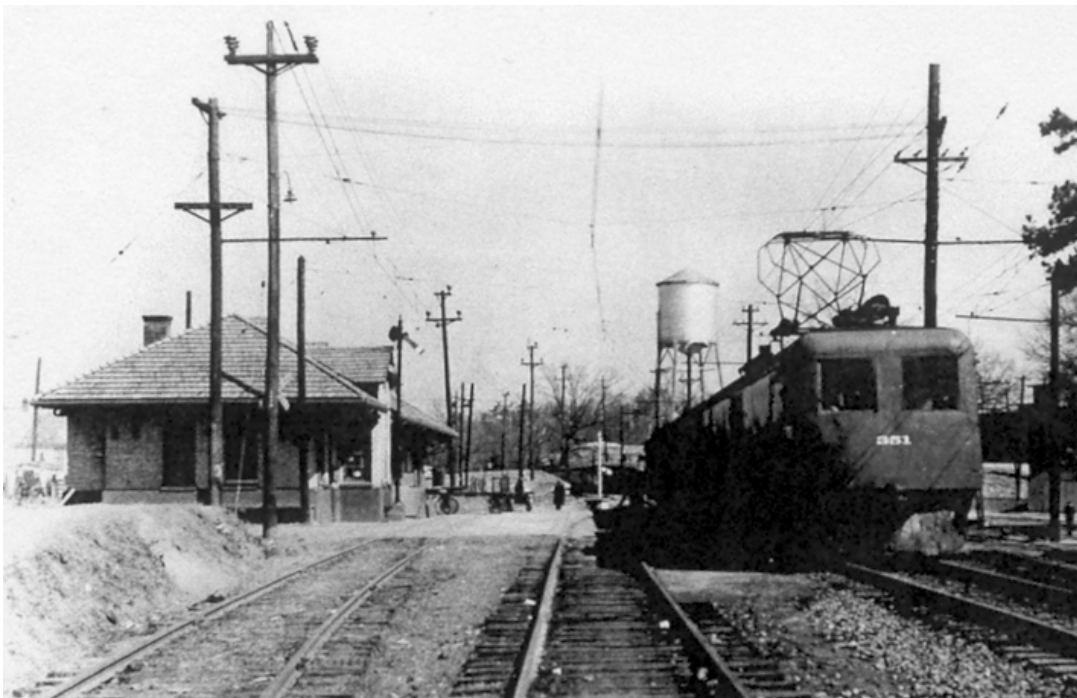
Figure 5.86: The station at Pelzer, South Carolina, during better days. Photo courtesy of Thomas Fetters.
