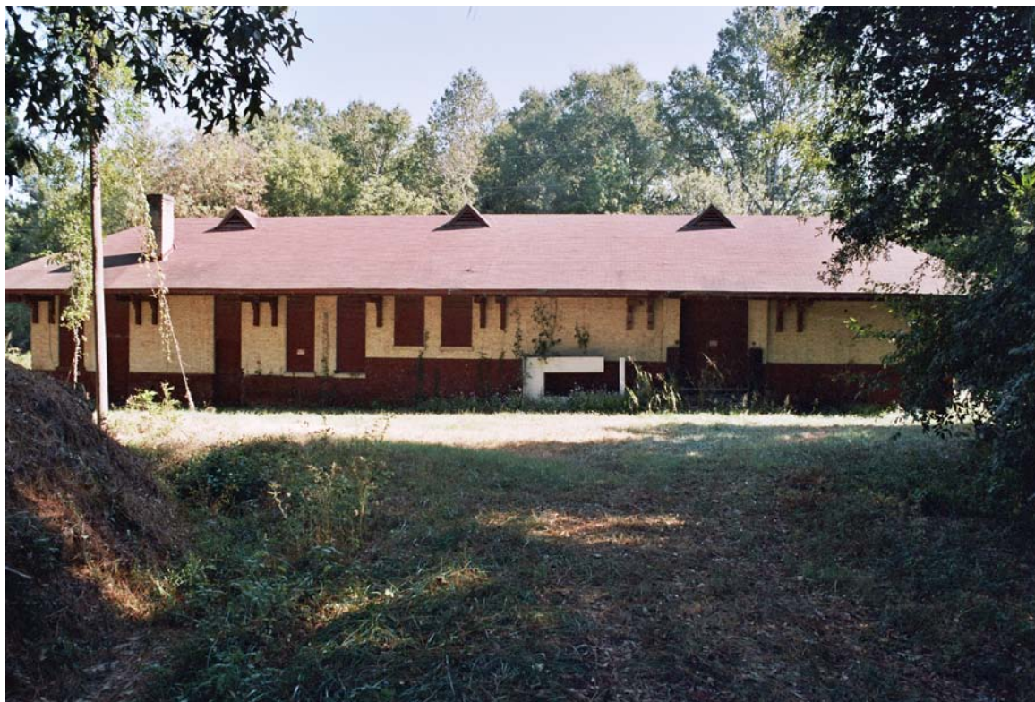
Figure 5.64: October 5, 2005. Profile of the Hodges station from the west.
