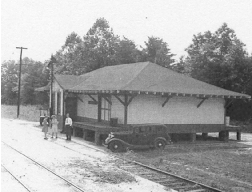
Figure 5.119: October 20, 2005. The small wood-frame station at Taylors, South Carolina. Photo courtesy of Thomas Fetters.
