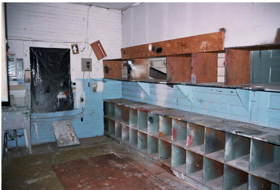
Figure 5.76: October 15, 2005. Interior of the "office." At right, blocked by the added cubbyholes, is the door into the freight room.
