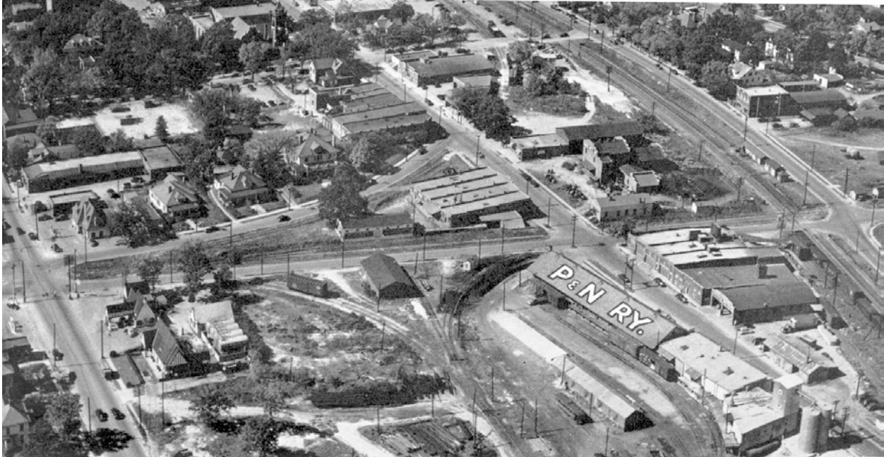
Figure 5.40: This aerial view of the P&N station at Gastonia is undated, but appeared on the cover of the August, 1950, issue of Semaphore Magazine. Note that the small passenger station shown the track chart above (Fig. 5.39) is missing; one of the buildings that has taken its place is – ironically – a gas station.
