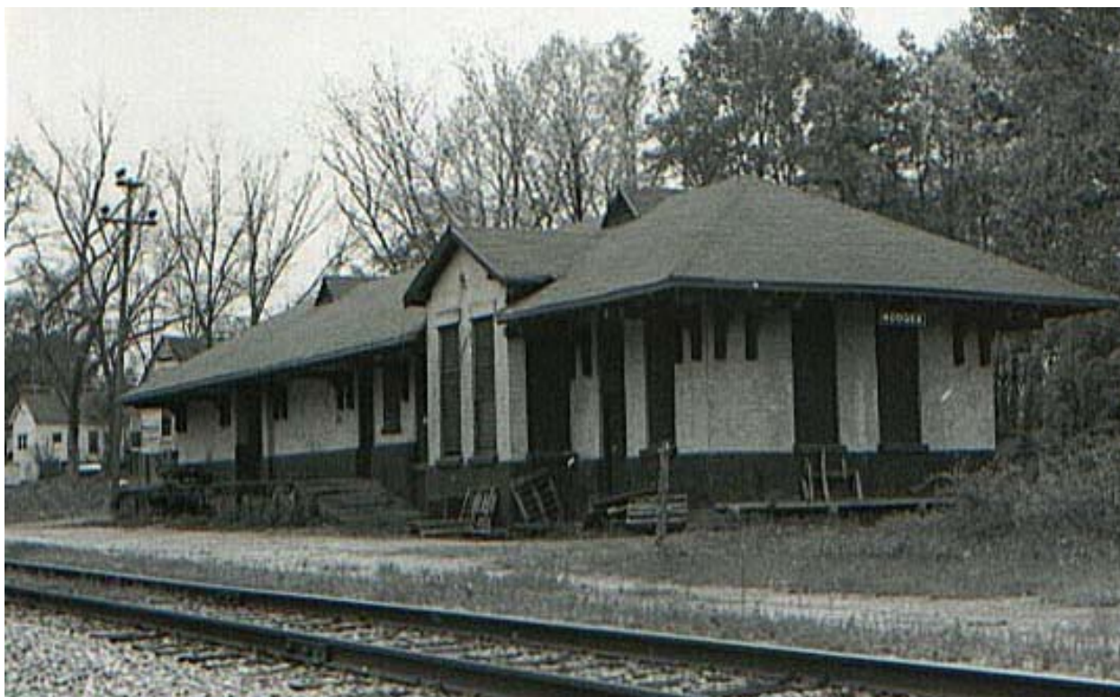
Figure 5.58: The Hodges, South Carolina, station, c. 1986.
