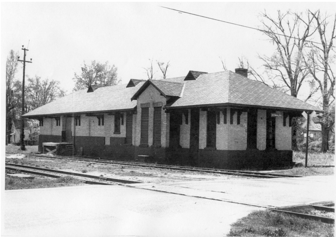
Figure 5.28: A trackside photograph of Donalds probably taken during its period of ownership by Seaboard Coast Line (the tracks have not been removed). Photo courtesy of Thomas Fetters.
