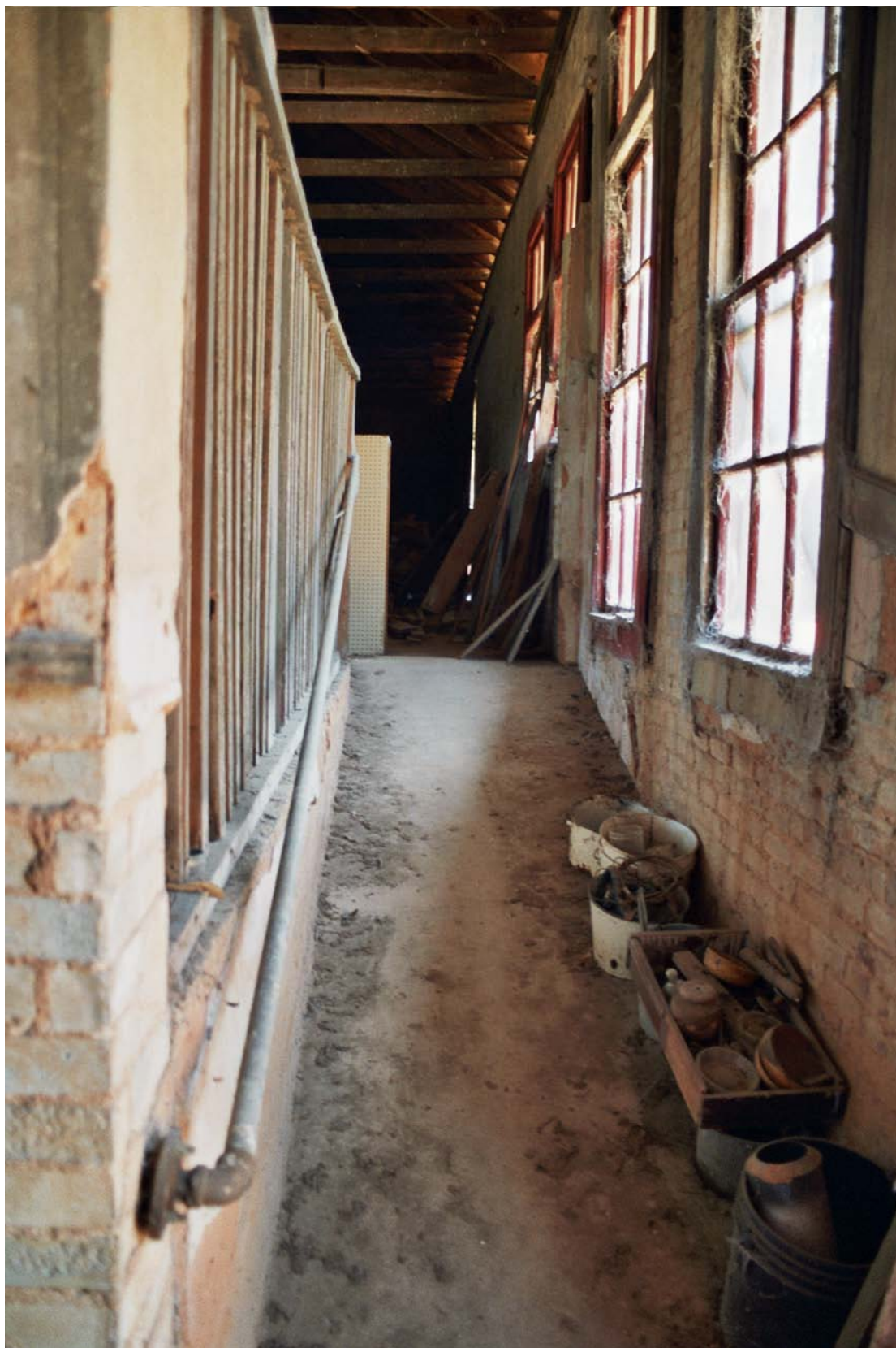
Figure 5.36: October 5, 2005. Ramp from the stationmaster's office up into the freight warehouse; the freight and express office is to the left of the pipe railing.
