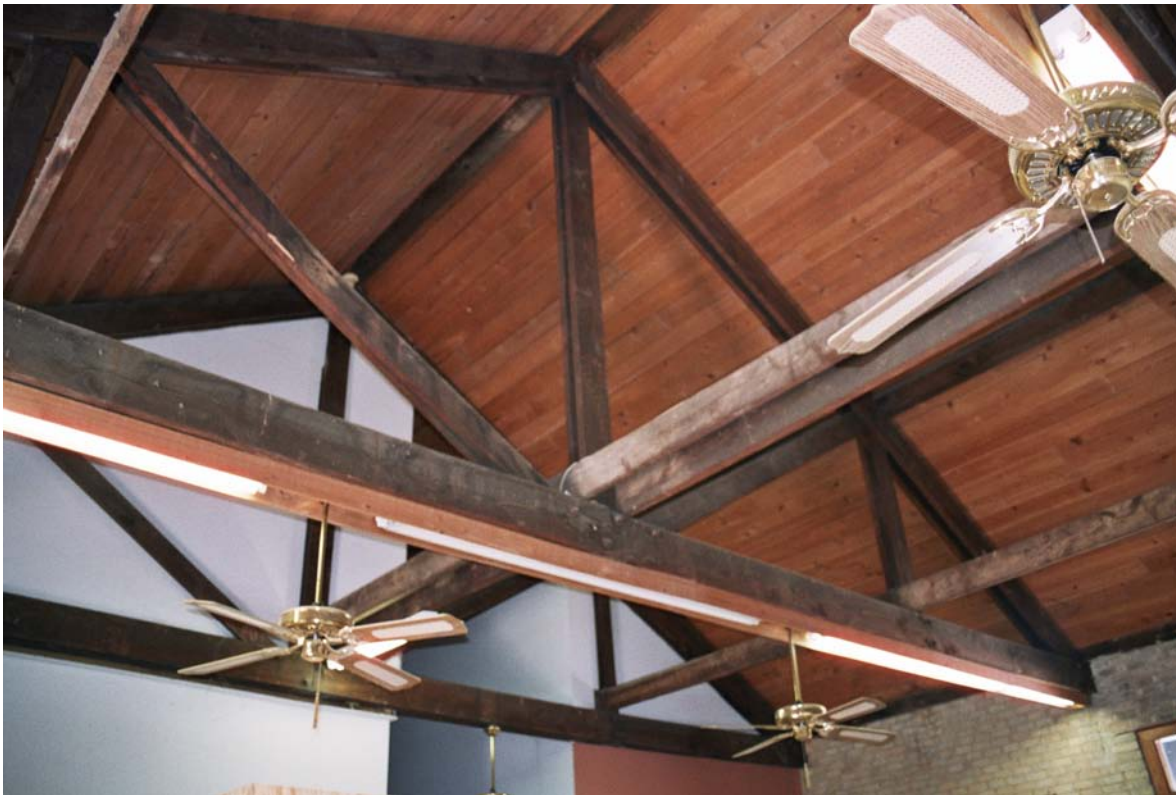
Figure 5.54: October 20, 2005. Detail of roof framing; note placement of fluorescent lighting.
