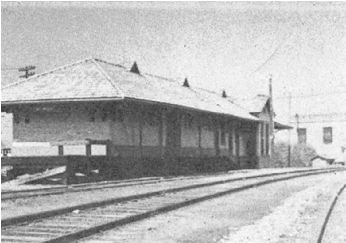
Figure 5.80: The west end of the Mount Holly station. Photo courtesy of Thomas Feters.
