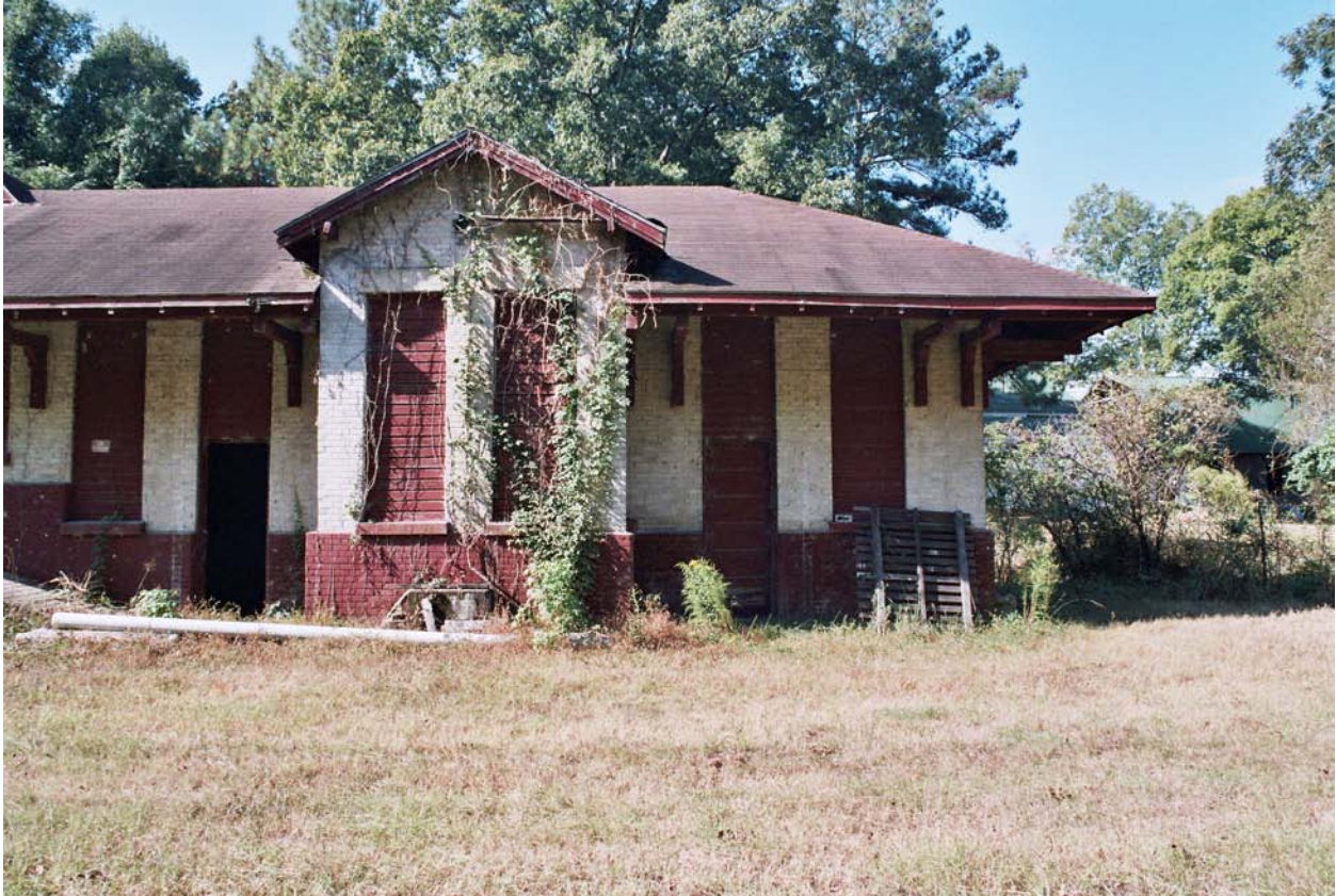
Figure 5.61: October 5, 2005. The “bay” of the stationmaster’s office at the north end. Door at right enters the passenger waiting room; door at left (standing open) enters the freight/express office.
