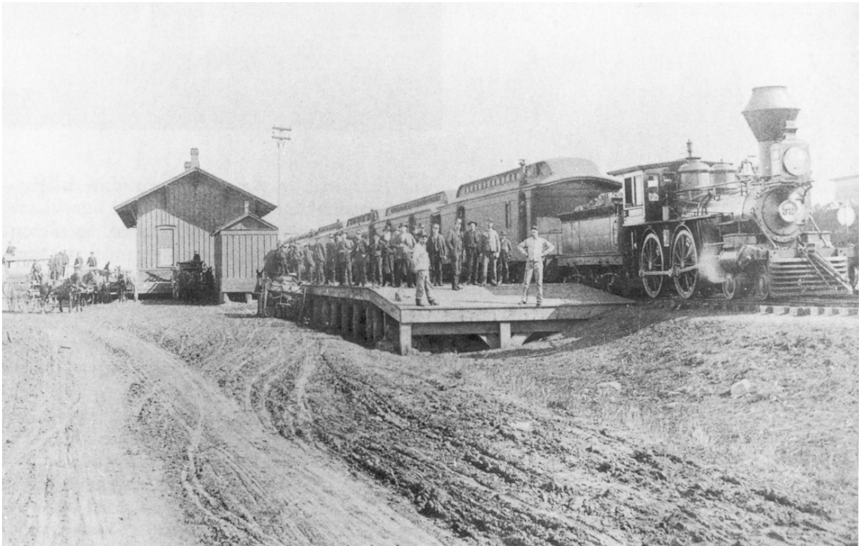
Figure 1.32 (Halberstadt, p.15): Wichita, Kansas, 1880. This photograph is remarkably similar to the painting by E.L. Henry (above) – almost beyond the point of coincidence.
