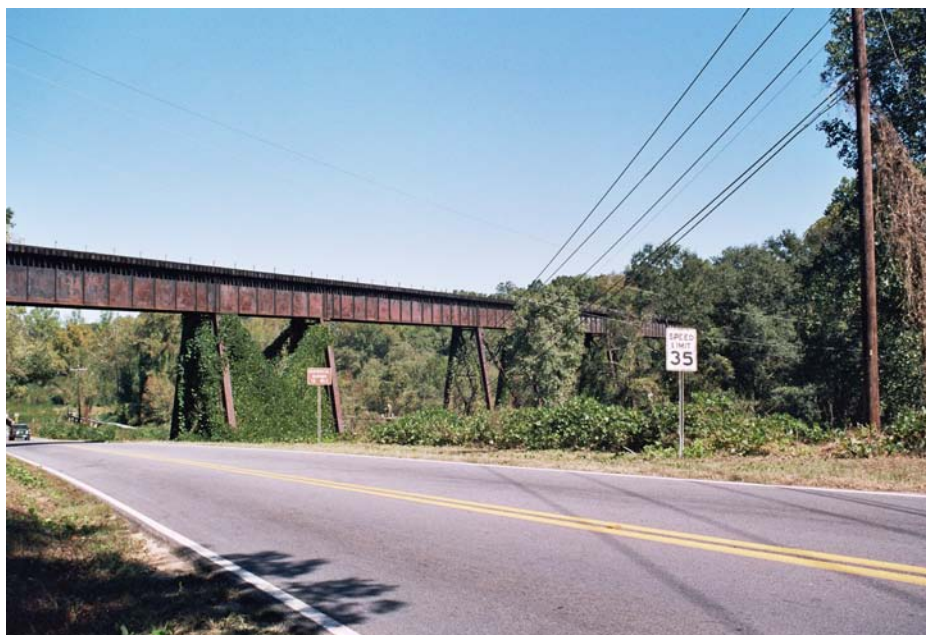
Figure 5.26: October 16, 2005. Although not a station, the steel “Chick Springs Bridge” is a significant landmark of engineering nonetheless; at eighty feet tall and about nine hundred feet long it is the longest and tallest bridge on the former P&N.
