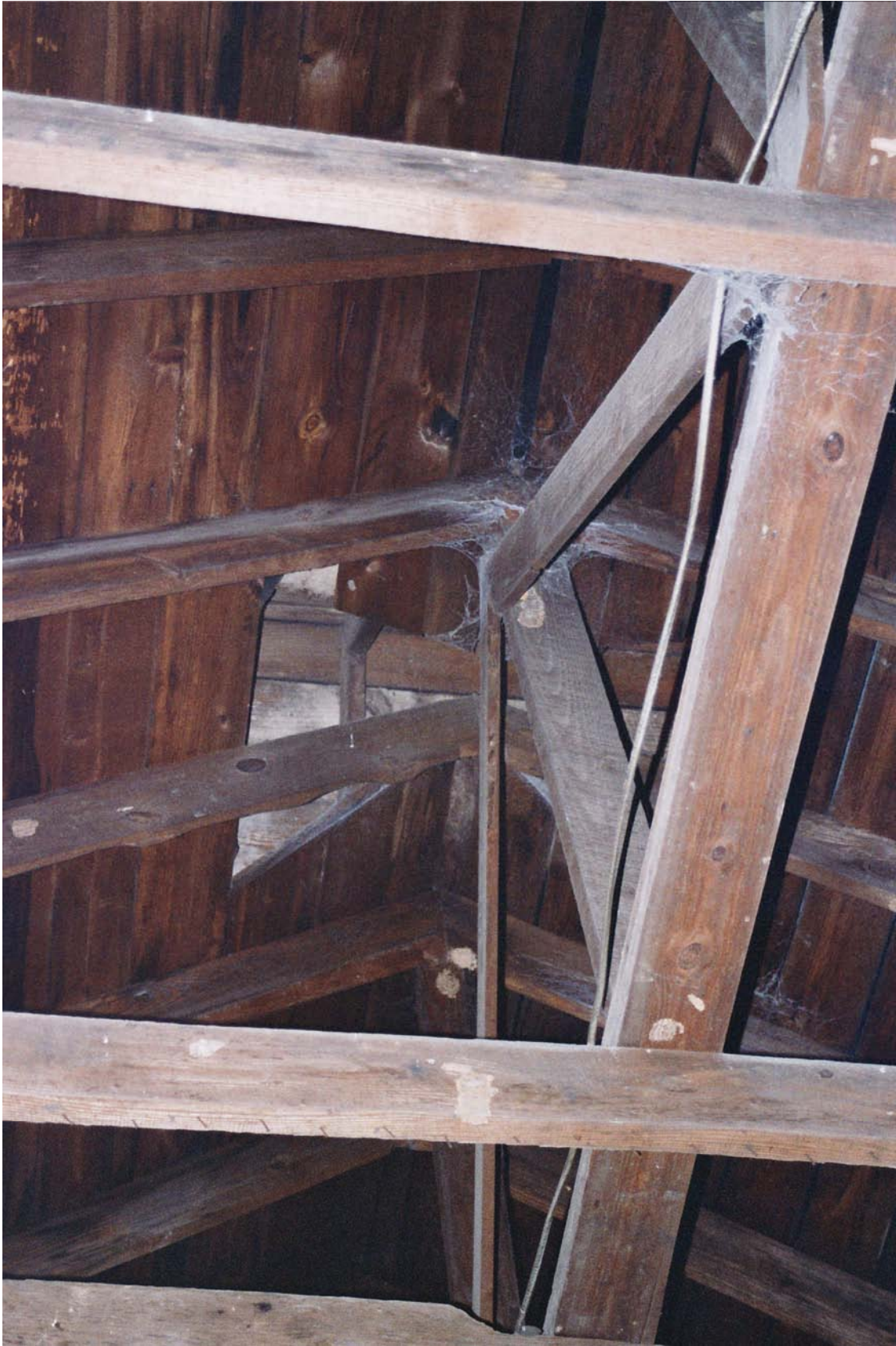
Figure 5.38: October 5, 2005. Framing, roof joists, and attic vent detail, Donalds.
