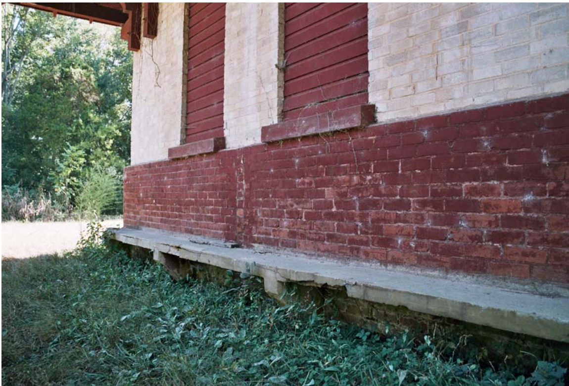
Figure 5.62: October 5, 2005. Concrete bench built into the north wall of the waiting room.
