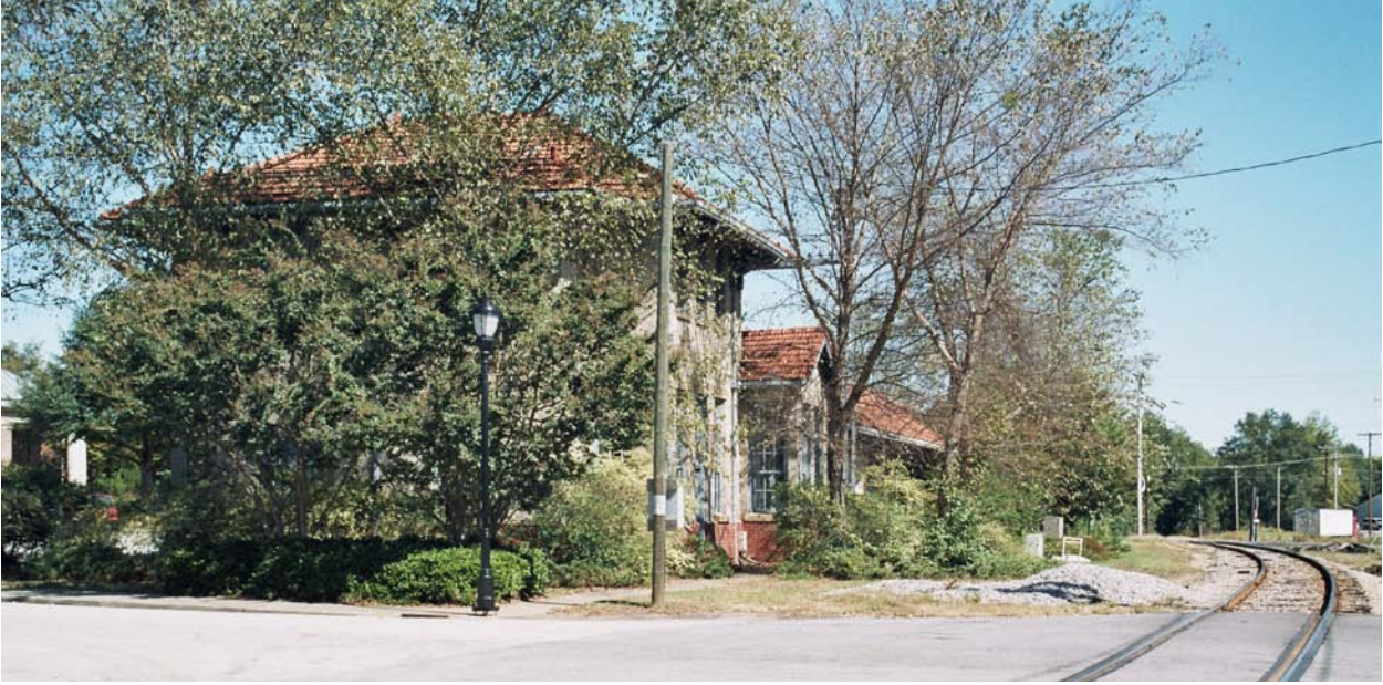
Figure 5.51: October 20, 2005. The site today.
