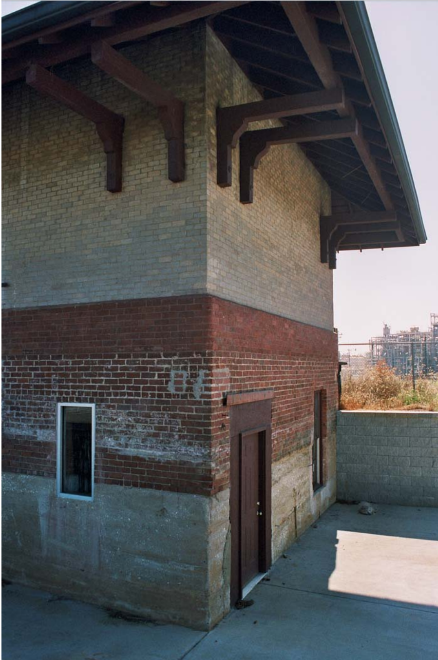
Figure 5.83: October 15, 2005. The earth has been excavated from the west end of the building apparently to create additional space for lease. Note the sealed windows below ground level in the foundation wall. Other ground-level air vents have been similarly filled. There is evidence of moisture problems (it may, however, date from before the rehabilitation and conceivably have led to the excavation at this end). With the care given to the rest of the building, this alteration is somewhat perplexing; it seems to reflect a “numbers-driven” philosophy of rehabilitation. Enclosing this space may prove to have no negative effects on the building, but it goes against the instincts of some preservationists.
