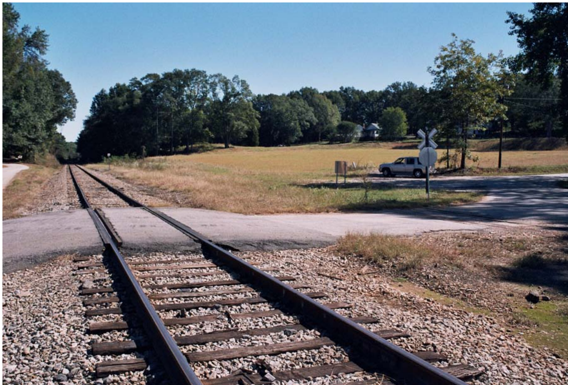
Figure 5.121: October 20, 2005. The site of the Taylors Station. Station probably stood where the vehicle is parked; an “H” shaped electrical pole barely visible indicates that the substation probably stood adjacent to the track and against the treeline in the background.
