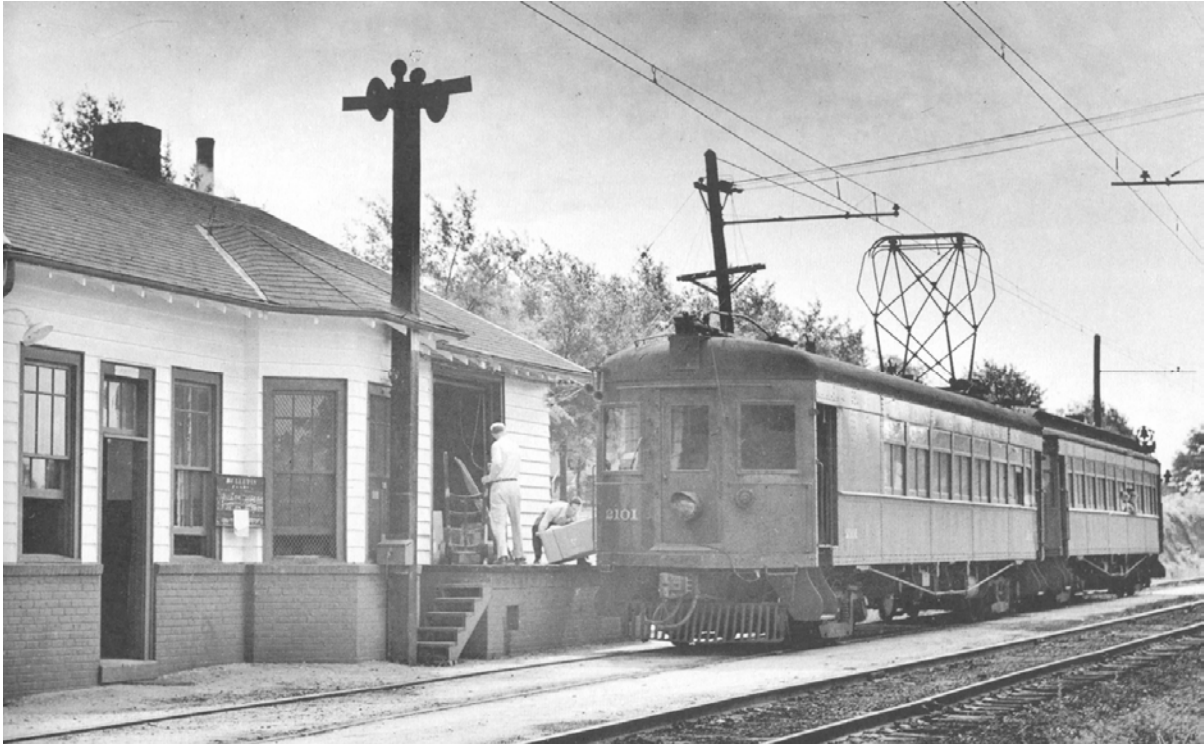
Figure 2.13: Express service was always a vital part of the P&N's income. Here, the expressman loads a heavy package onto express motor No. 2101 at Lyman, South Carolina. Note the other parcels just inside the freight door. Fetters and Swanson, p. 77
