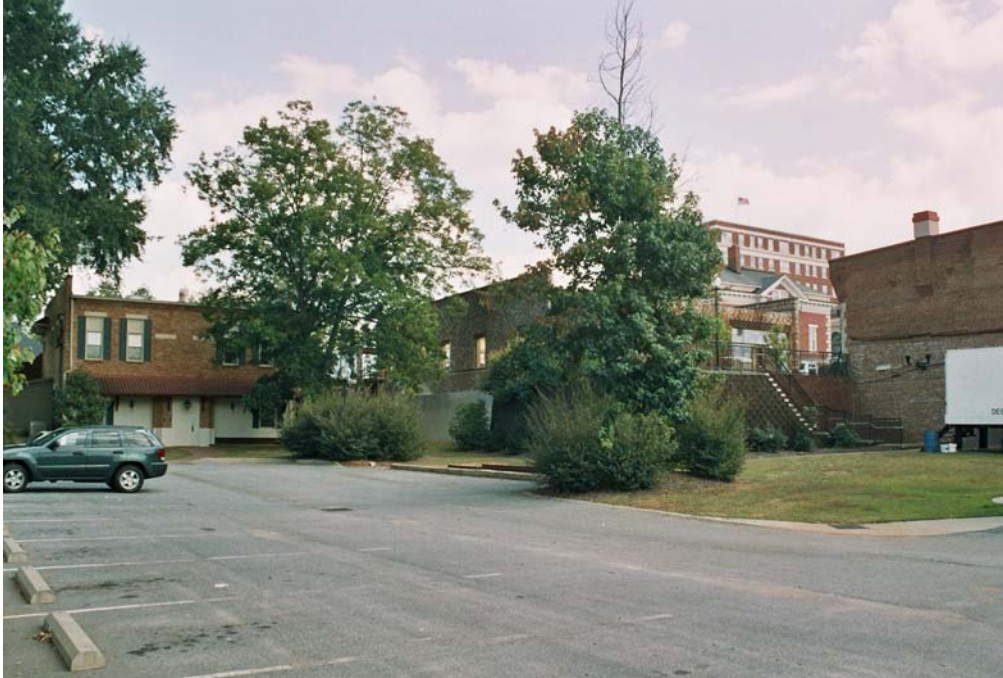
Figure 5.7: October 5, 2005. The rear of the Anderson passenger station (two story brick building with shed roof at left). In the center (between the bushes) is a short length of track to suggest the building's original role; the freight station is out of view to the right.
