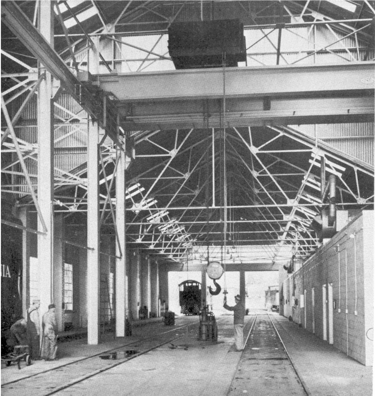
Figure 5.104: Interior view of the main shop looking west, about a year after it was completely remodeled for diesel maintenance. Note the height of the horizontal braces in the superstructure; these would be too low to accommodate the much taller locomotives in use today. Office and storage rooms are on the right; the remodeling was designed and carried out by the architectural and engineering firm of J.N. Pease & Co. (which took the photo), Charlotte. Semaphore , November, 1955.
