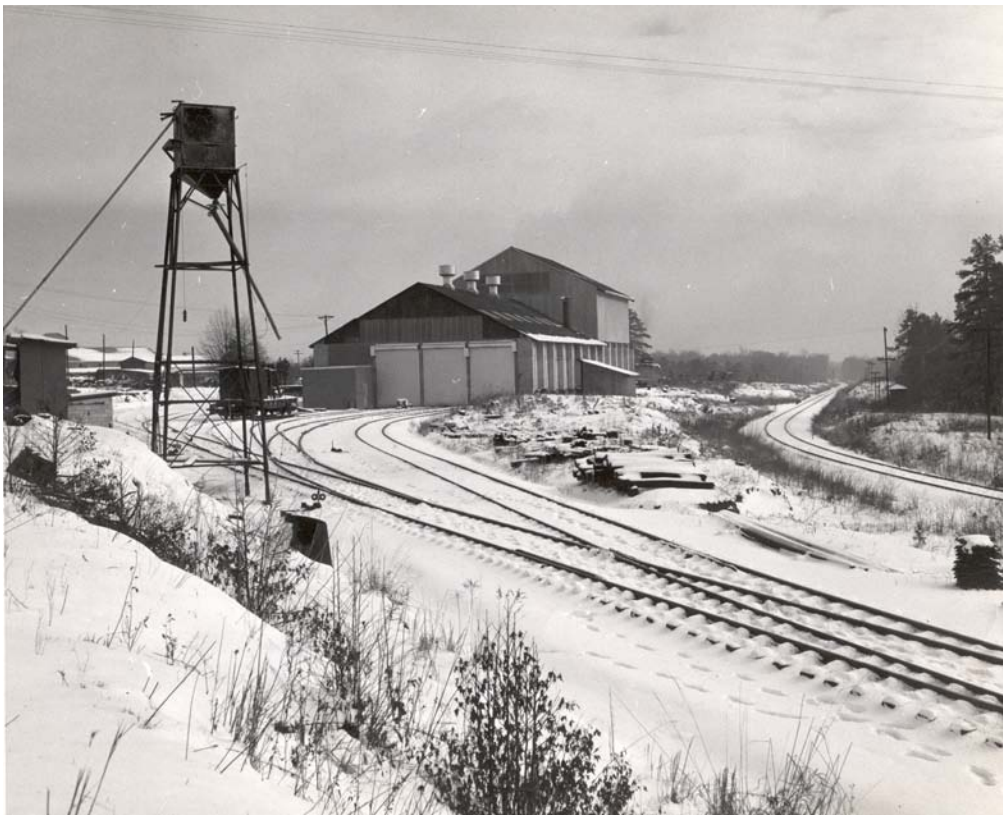
Figure 5.103: Pinoca shops, late 1950s, looking towards Charlotte. In the left foreground is the sand tower, used for getting sand into locomotive sandboxes. Fine grain (to reduce wear on the rails) sand has always been carried on locomotives to limit wheelslip and gain traction under slippery track conditions (such as the snow and ice seen here).
