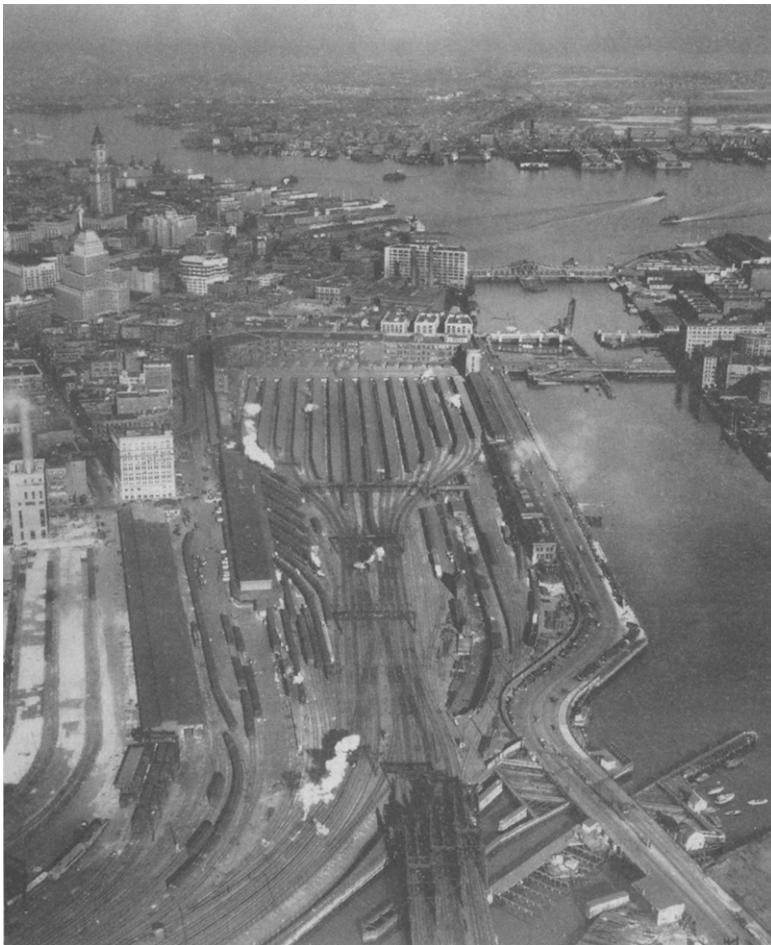
Figure 1.24 (Potter, p. 34): The throat of Boston's South Station, c. 1930. The large "X" shape in its center indicates the presence of a double-slip switch. Mail and express platforms line the left hand side of the facility while platform tracks fan out to reach the head house.
