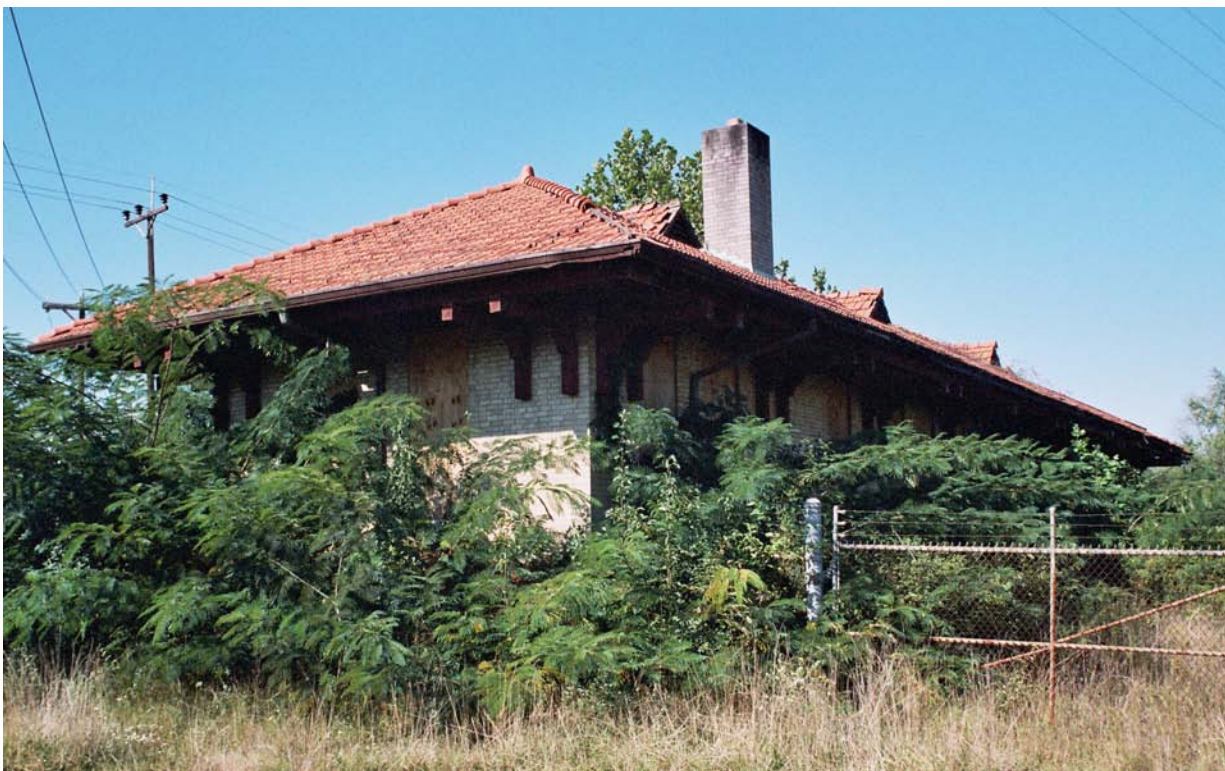
Figure 5.126: October 18, 2005. Unfortunately, this is as much as can be seen of the Thrift station.
