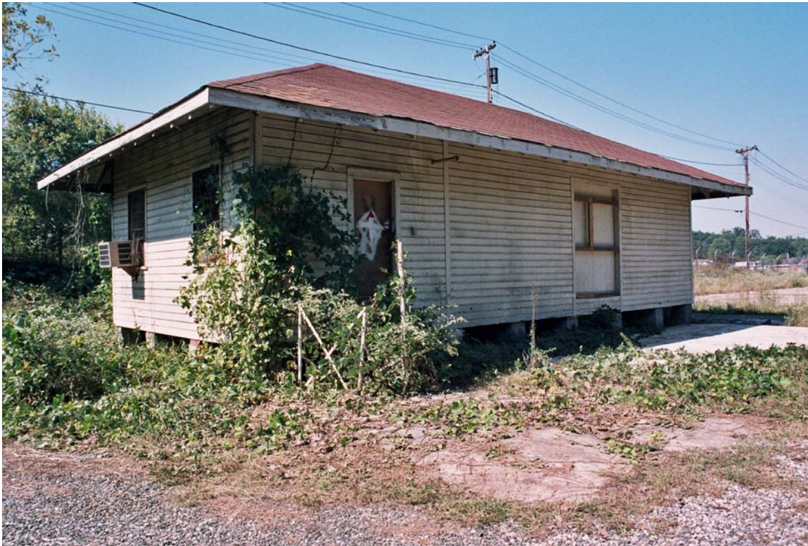
Figure 5.74: October 15, 2005. View of the "office" end of the building.
