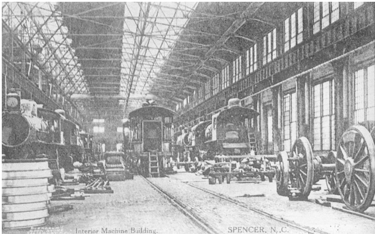
Figure 1.4 (Sides, p. 74): Interior of the back shops at Spencer.
