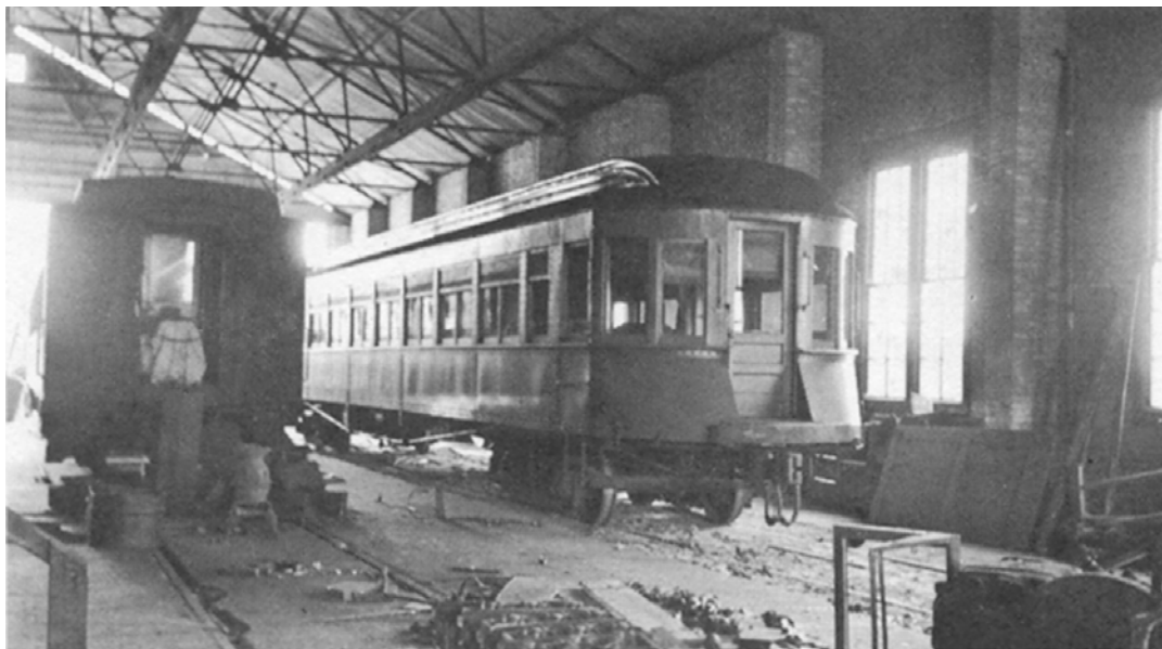
Figure 5.108: The River Junction Shops were always the P&N's main shop facility. In this interior view from about 1935, probably of the original shop building (note the windows), the car on the right is the former business car Catawba , which is nearing completion as a first-class fare parlor car. Its original open observation platform has been enclosed and it has been given a "boat tail," inside of which are parlor chairs.
