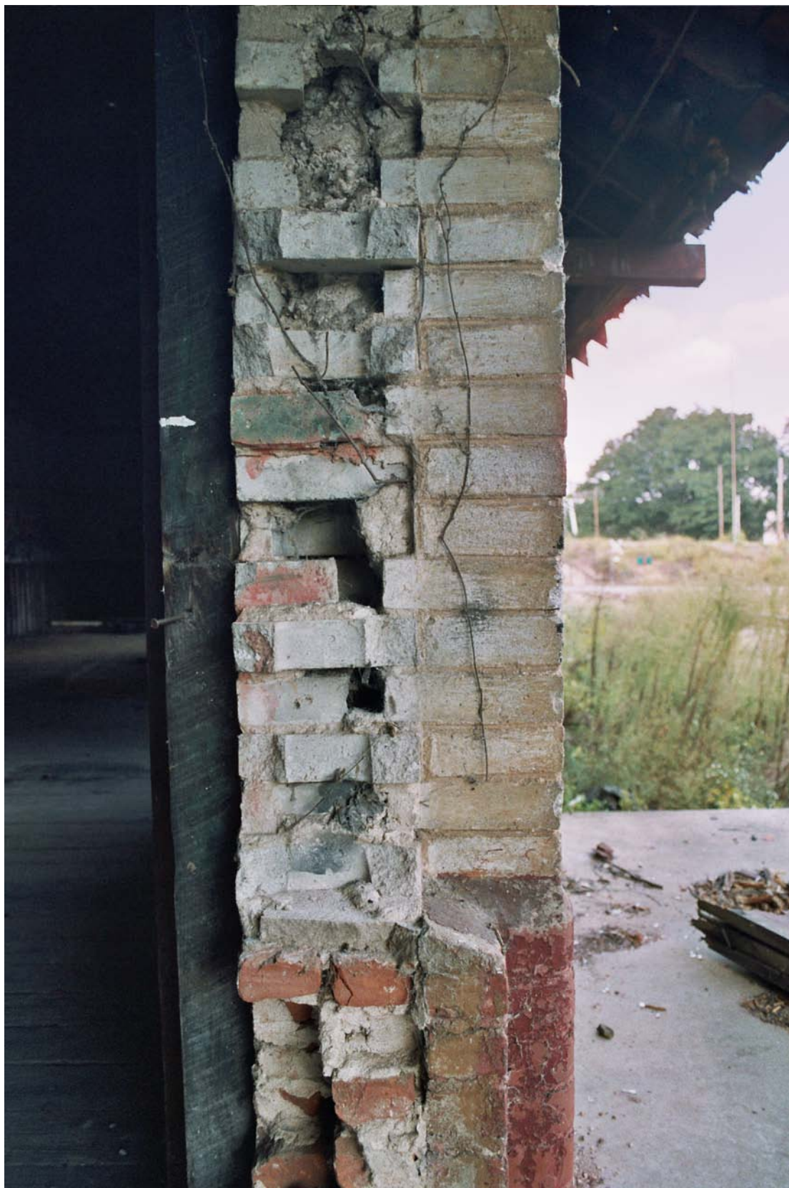
Figure 5.91: October 5, 2005. A very large section of the trackside wall has been knocked out, revealing a cross-section of the brick construction.
