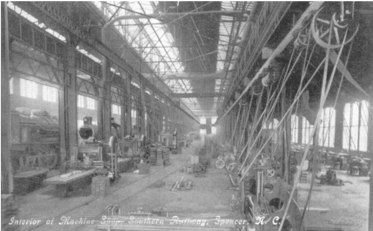
Figure 1.6 (Sides, p. 65): The machine shop.
