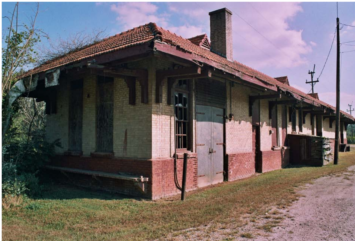
Figure 5.98: October 5, 2005. The passenger end (north) of the building.
