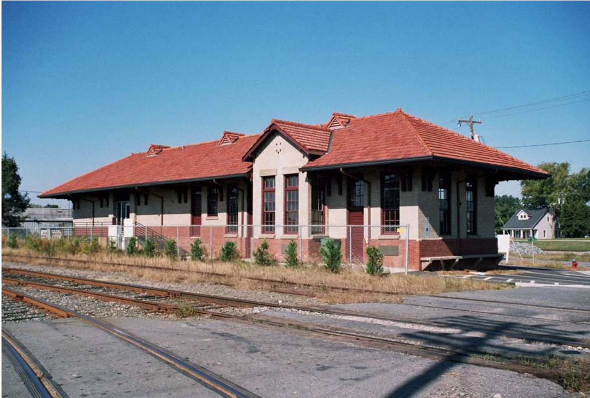
Figure 5.79: October 15, 2005. Today, the Mount Holly station appears to have a secure future. Although it has been necessarily altered, the changes are, for the most part, slight, and at least from the outside it would appear that the rehabilitation work is being carried out with great care.
