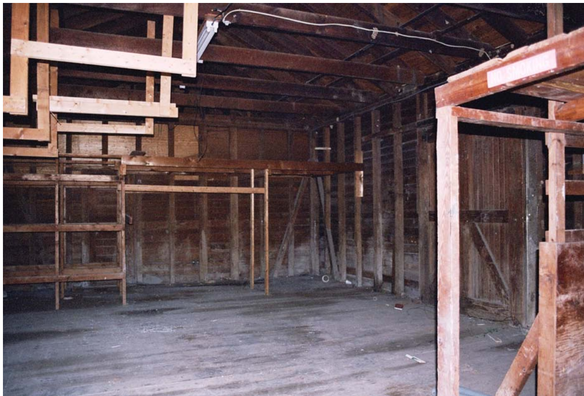
Figure 5.75: October 15, 2005. Interior of the freight room, McAdenville. Note the door at left in the far wall.
