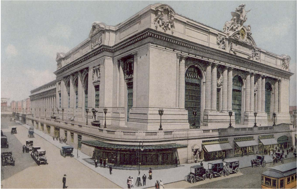
Figure 1.63 (Holland, p. 18): Grand Central Terminal, giving its regards to Forty-second Street.
