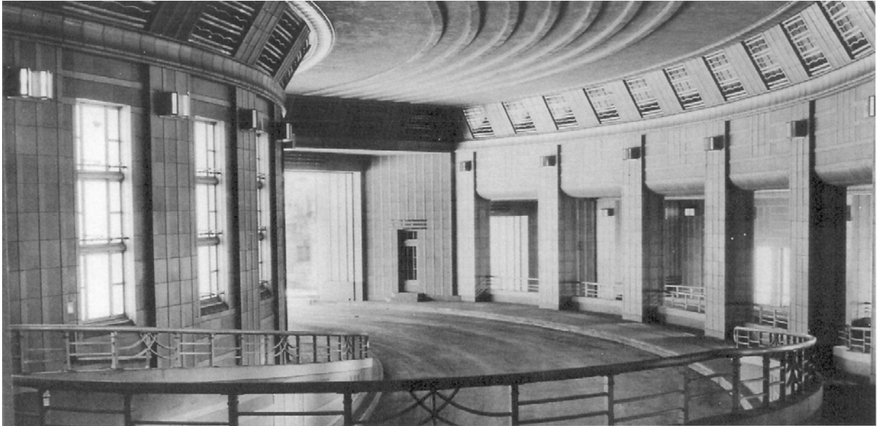
Figure 1.71 (Doughty, p. 115): The taxi lane emerges from beneath the domed concourse to pick up people from the exit platform (Fig. 1.70, lower left).
