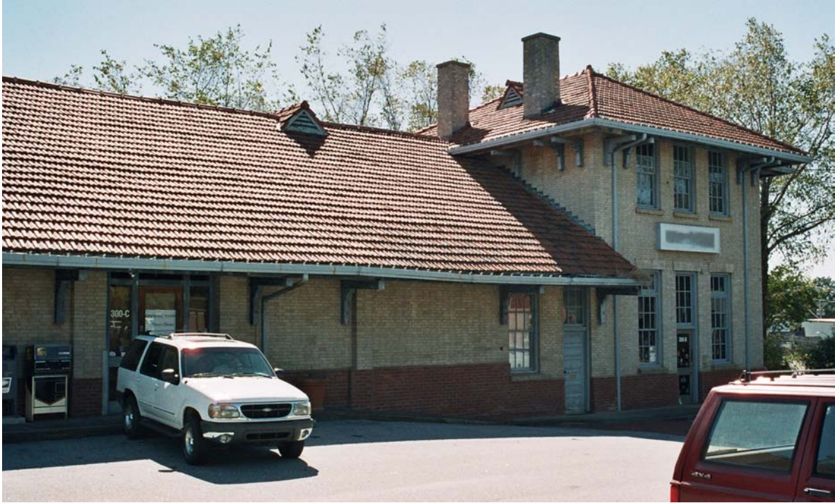
Figure 5.55: October 20, 2005. The two story block at Greer is the only remaining example. Interior photographs were taken in the space directly behind the white Ford. Aside from the red watertable, the choice of color for the building's trim is not in keeping with the original color of doors, windows, cornice brackets, etc. The dull gray mutes what few details Hook relied upon to "show off" the building.
