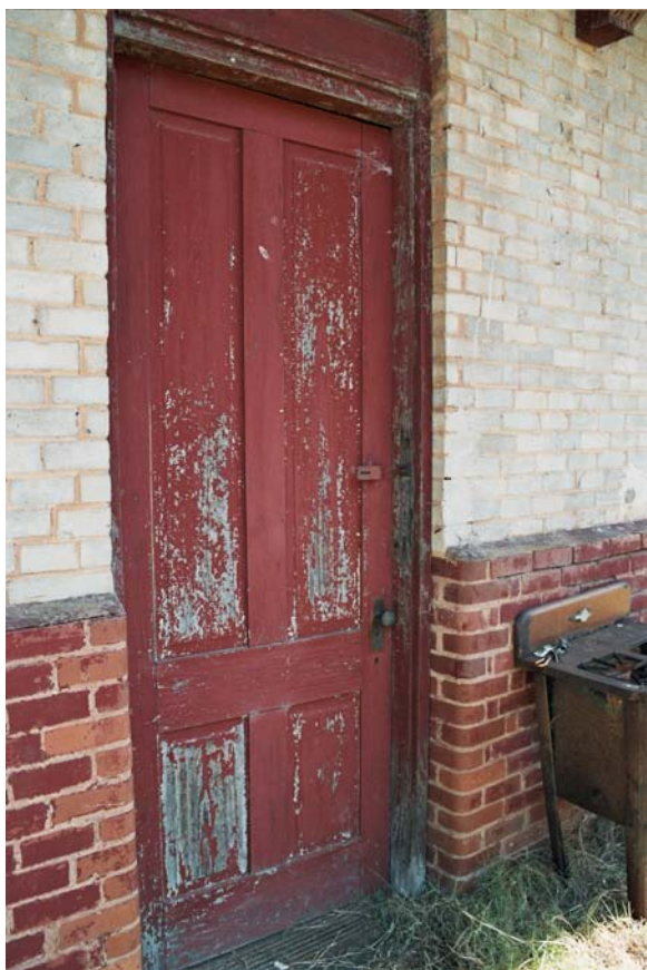
Figure 5.32: October 5, 2005. Detail of door to stationmaster's office, Donalds.
