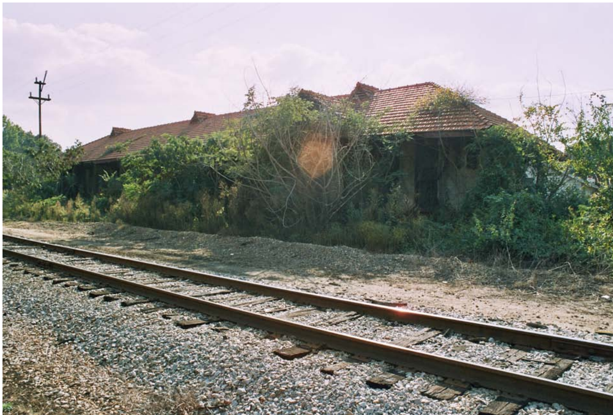
Figure 5.97: October 5, 2005. Trackside elevation of the Piedmont station.
