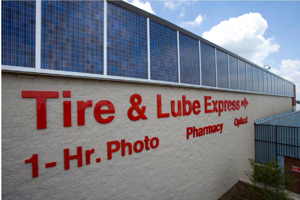
Figure 5.5: Solar panels form the “signature blue stripe” across the façade of the McKinney, TX experimental supercenter. 274
