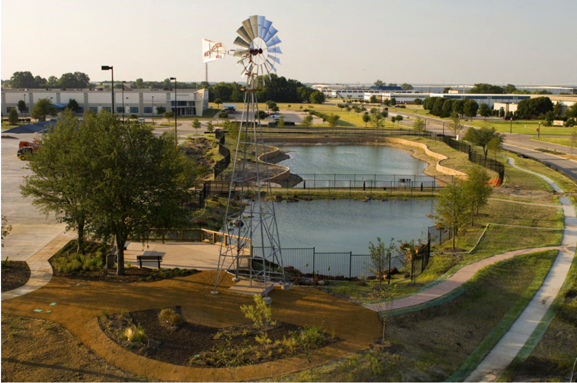
Figure 5.4: Stormwater retention ponds and constructed wetlands at McKinney, TX. 223
