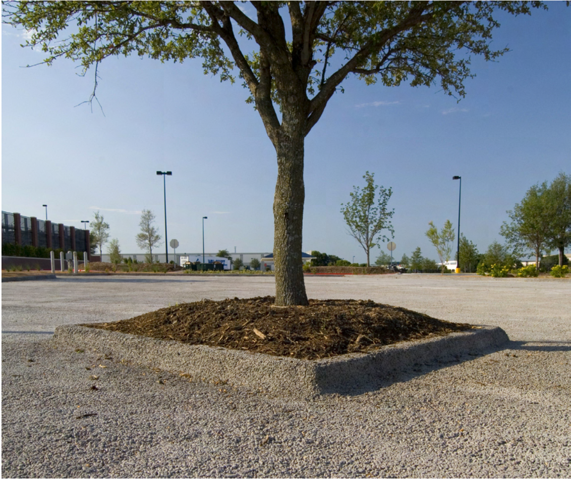
Figure 5.3: Porous pavement at McKinney, TX. 217
