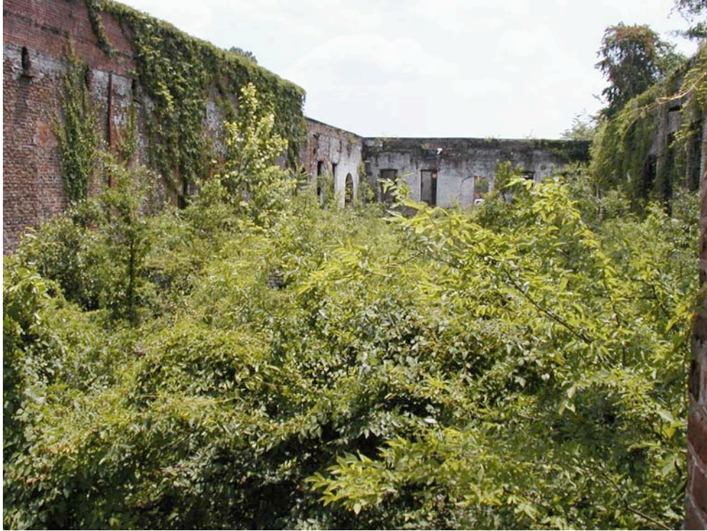
Figure 6-5. Ruins of Carpentry Shop Before Being Cleared For Preservation Work (Source: Coastal Heritage Society).
