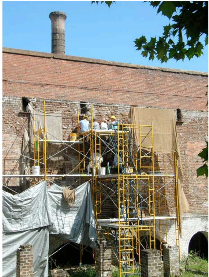
Figure 6-4. CHS Preservation Team Repoints East Wall of the Carpentry Shop (photo by author).
