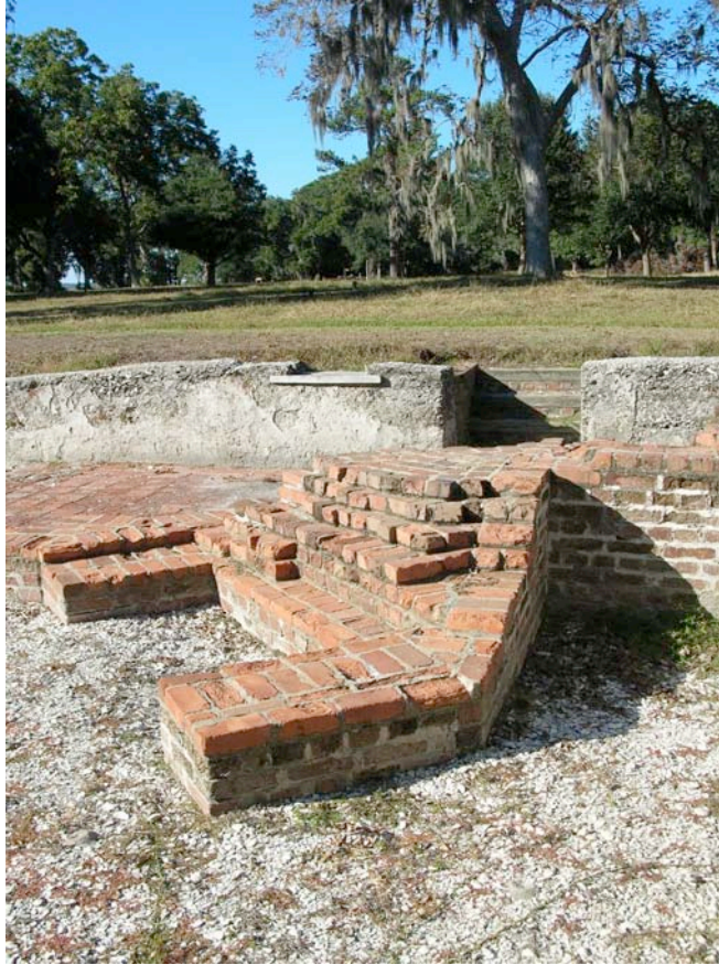
Figure 7-12. New bricks pointed with Portland cement and placed over original materials (photo by author).
