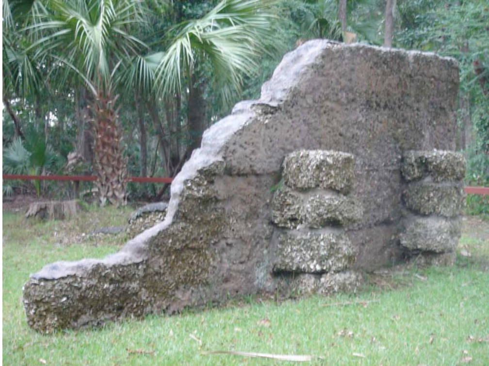
Figure 5-7. View of Tabby Wall (photo by author).
