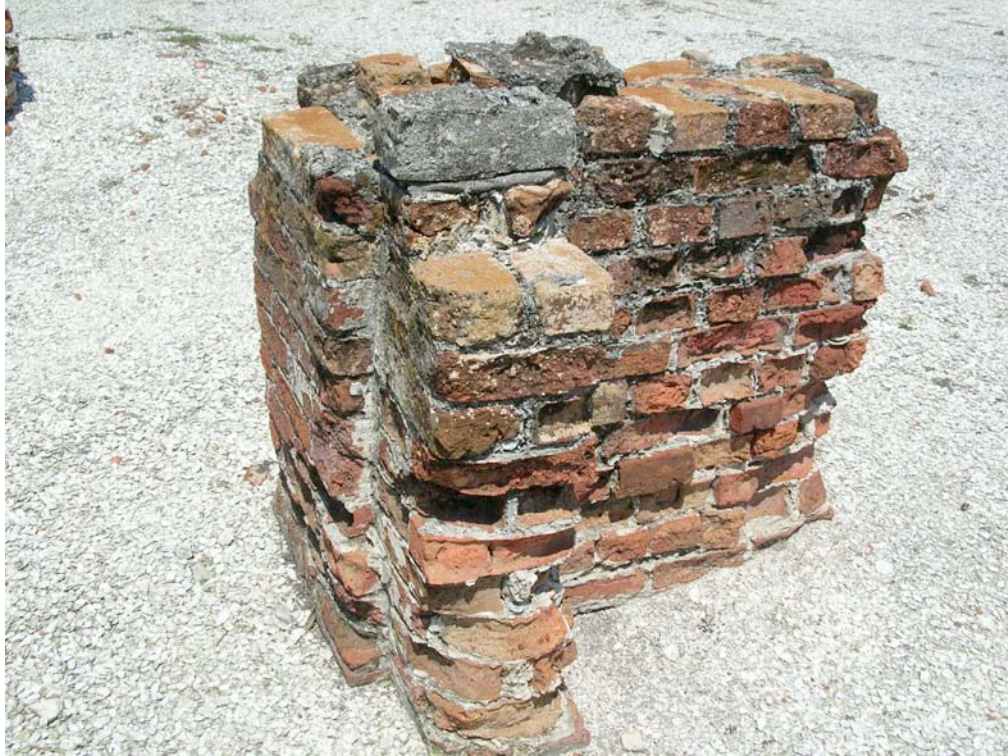
Figure 7-8. Close-up View of Brick Footing at Main House (photo by author).
