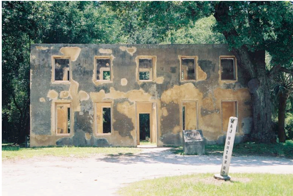
Figure 3-3. Horton House after 2004 Preservation Work (photo by author).
