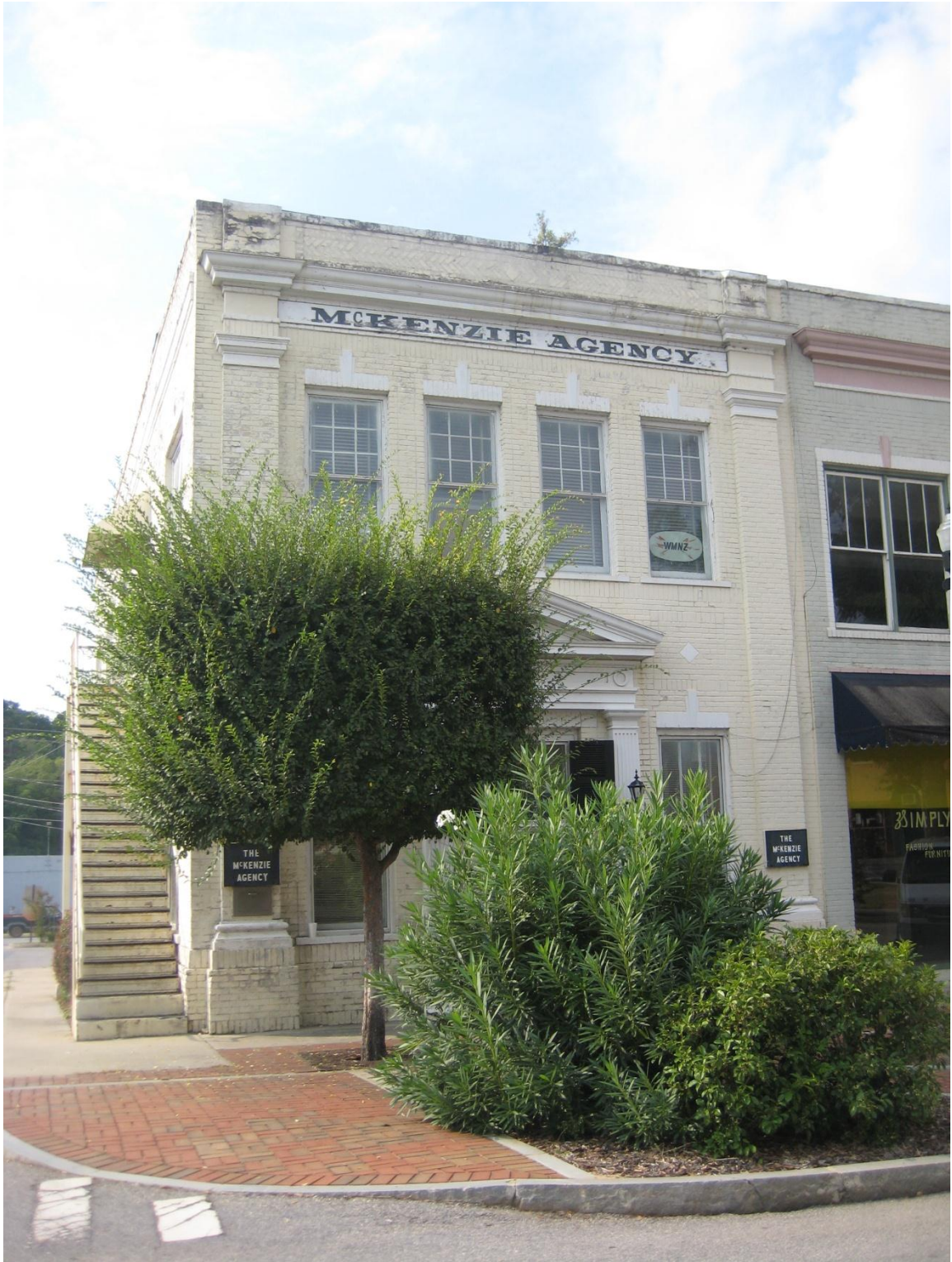
Figure 19. Current state of 115 Cherry Street, the McKenzie Building.
