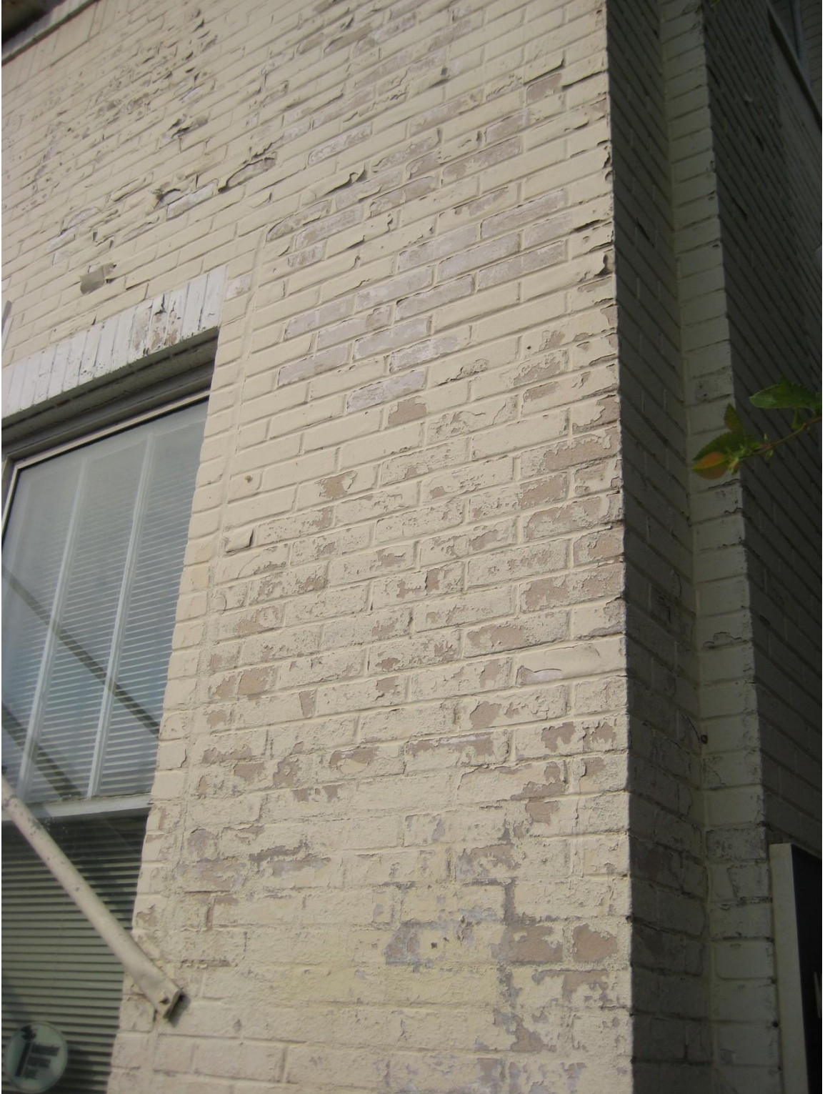
Figure 17. Current state of McKenzie Building. West elevation detail. 108
