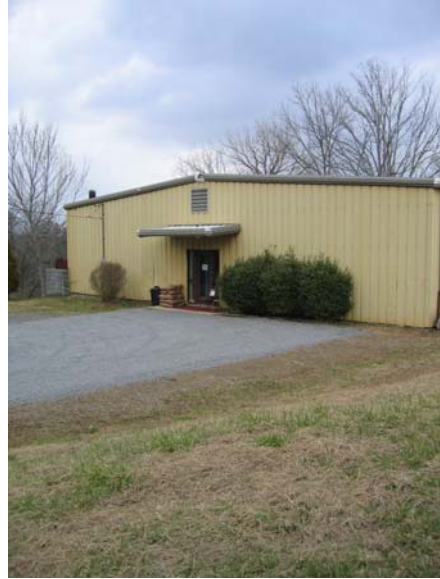
Figure 2.2. Texana Community Building
