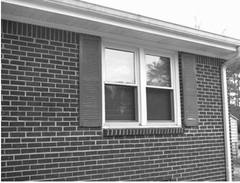
Figure 72. Double-hung sash windows. Powder Springs, Georgia.
