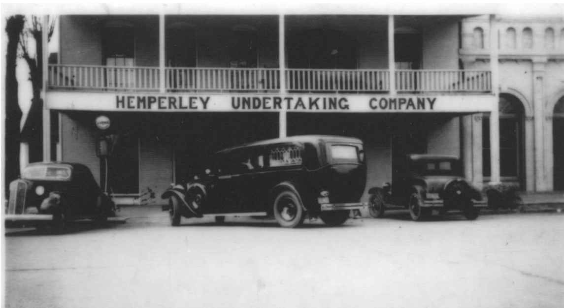
Figure 24 Hemperley Undertaking Company
