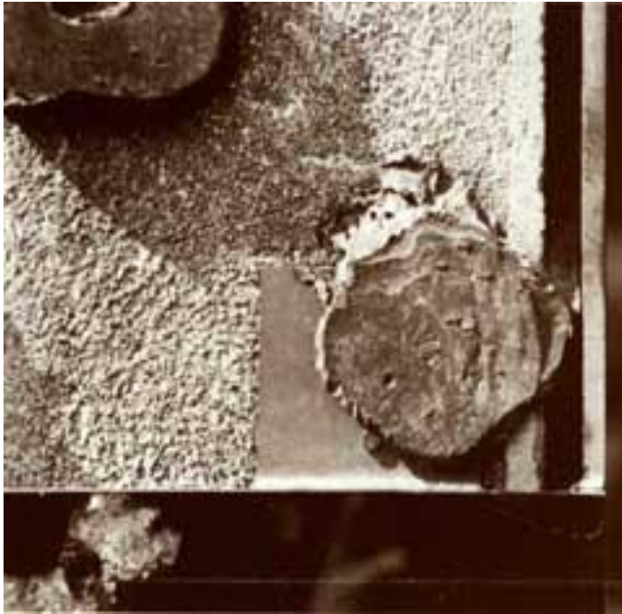
Figure 25 brittle daub of mastic
