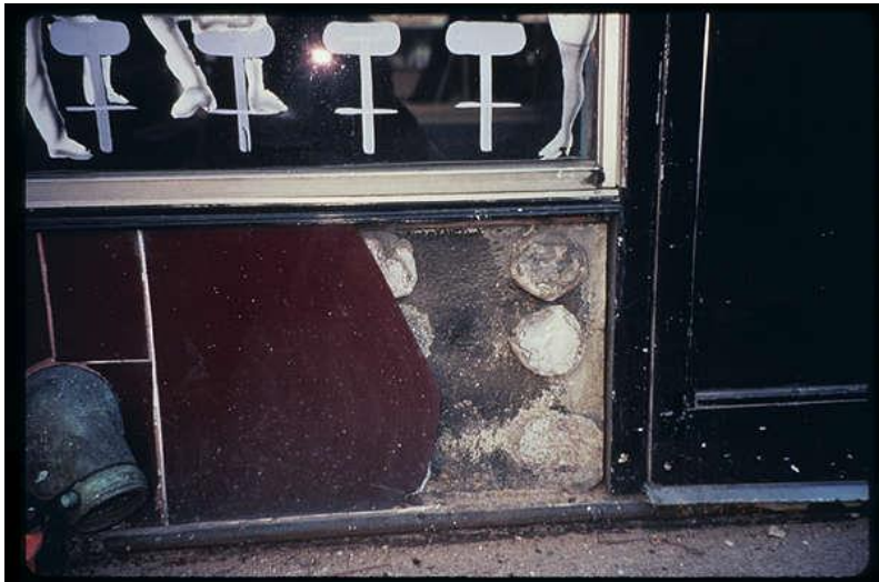
Figure 26 structural glass damage from impact or vandalism
