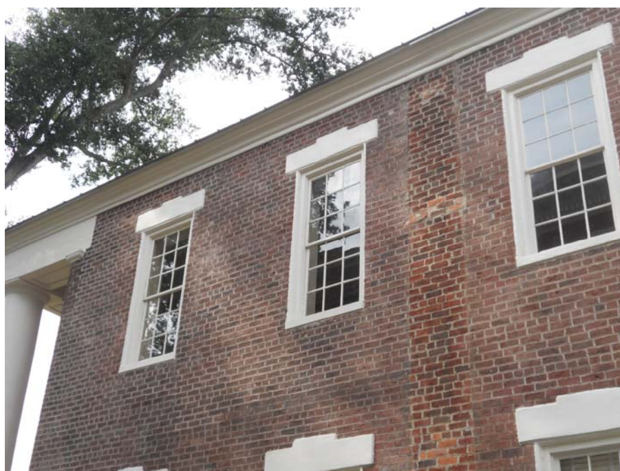
Figure 41: South façade of Phi Kappa Hall showing the color change caused by the repeated application of water proofing material to the exterior prior to a chimney addition being removed
