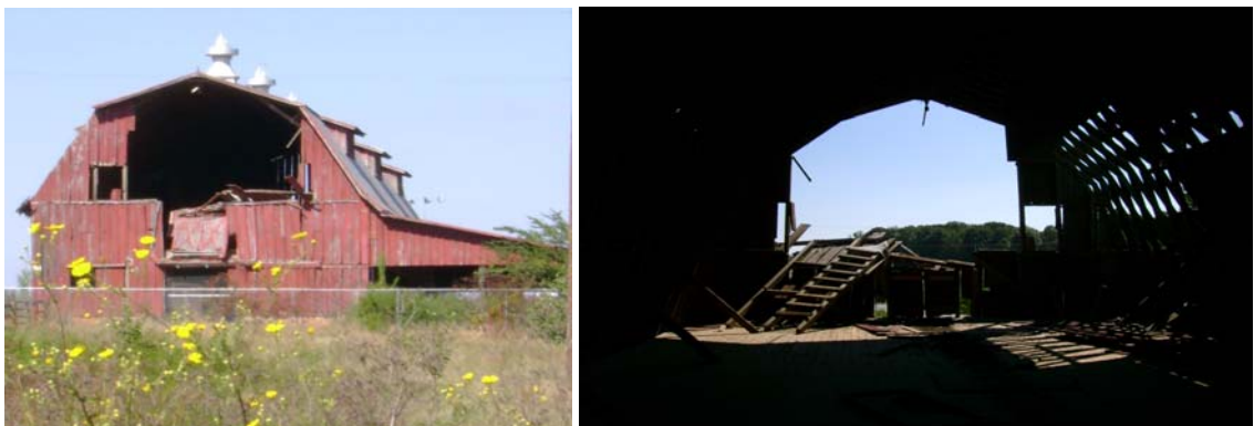
Figure 7: Interior and exterior storm damage to the Red Barn (Photo by Author)
