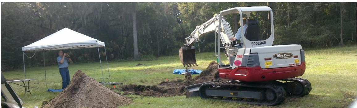
Figure 5.4: Excavation of the soil pit.
