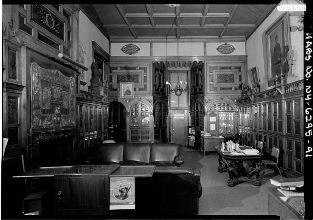
Figure 26. Company K Room, 1984 image
