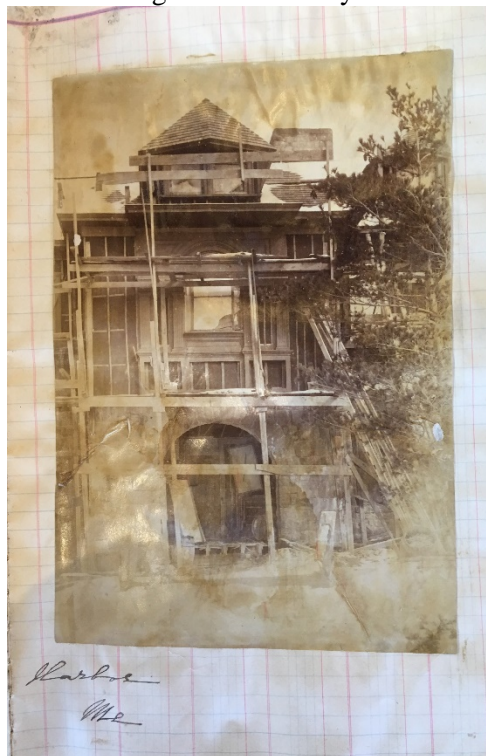
Figure 53. Ban-y-Bryn under construction, entrance, from Stratton's scrapbook
