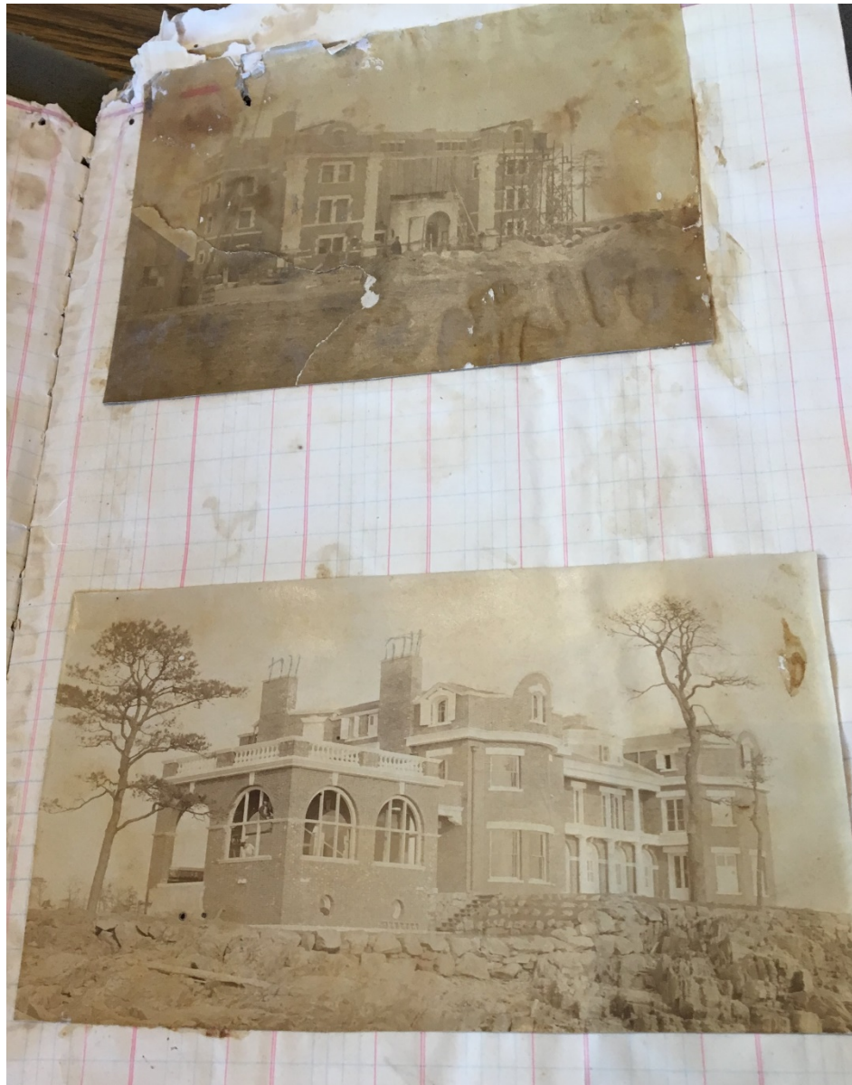
Figure 76. Iselin House under construction, Stratton's Scrapbook
