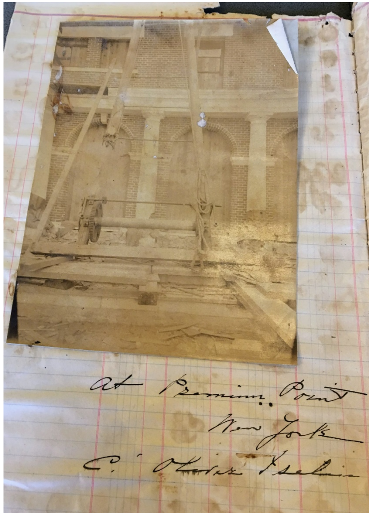
Figure 75. Iselin House under construction, Stratton's Scrapbook
