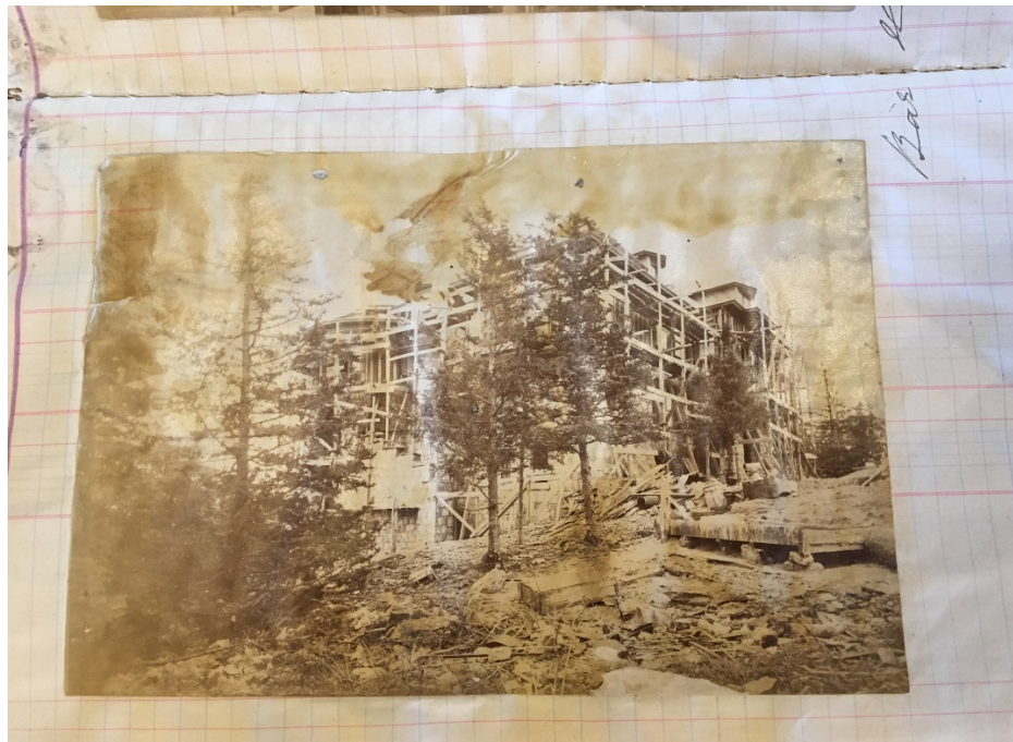
Figure 54. Ban-y-Bryn under construction, from Stratton's scrapbook
