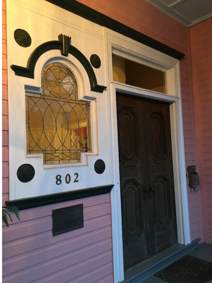
Figure 34. John Dicks House, entrance detail
