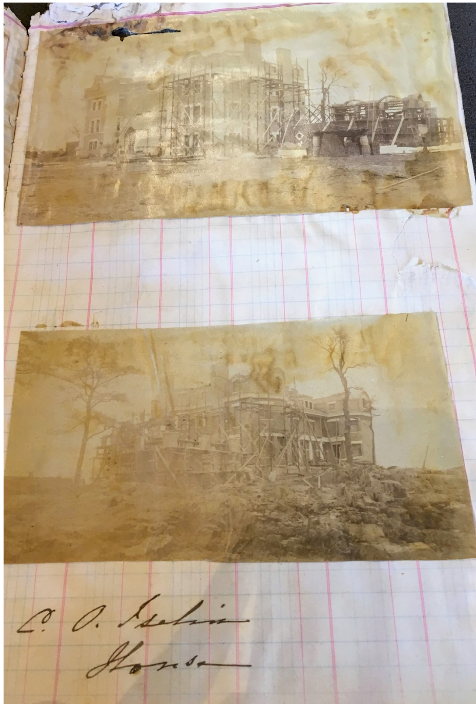
Figure 77. Iselin House under Construction, Stratton's Scrapbook
