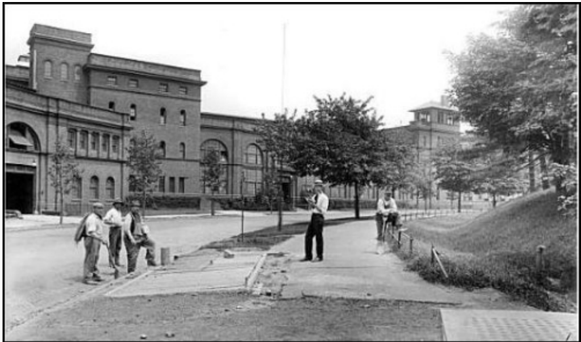
Figure 63. Brooklyn Riding and Driving Club, view along Plaza Street, the entrance to the garage is at the left
