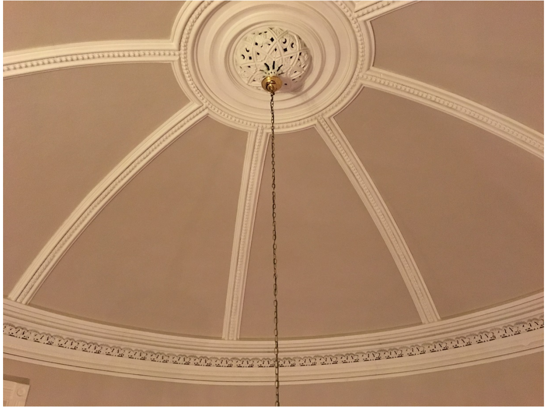
Figure 37. John Dicks House, dome over entry hall
