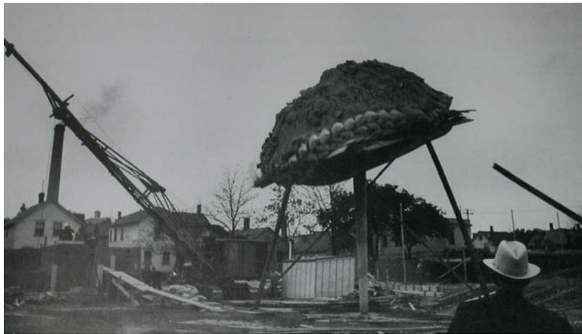
Figure 21: The column collapsing, Mr. Wright in the foreground
