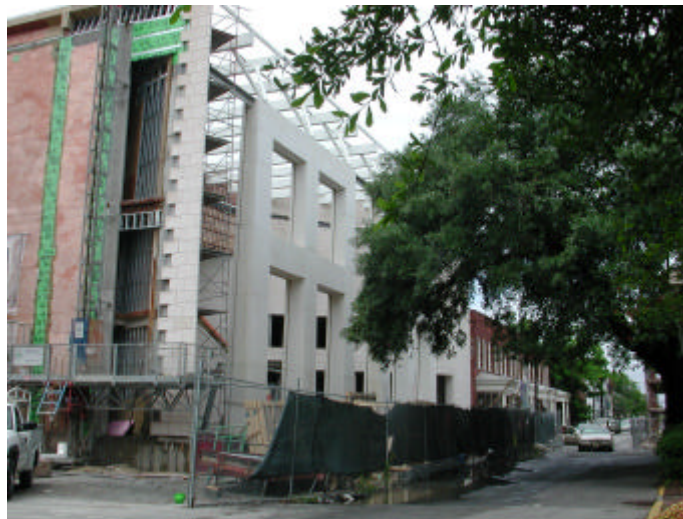
Figure 5-7 Jepson Center north façade under construction
