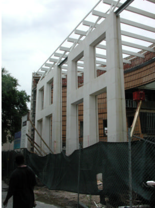
Figure 5-9 Jepson Center entrance under construction
