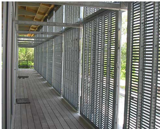
Figure 5.3. When closed, external shading devices create a shady breezeway. (Source: Beth Broome, Architectural Record Magazine)
