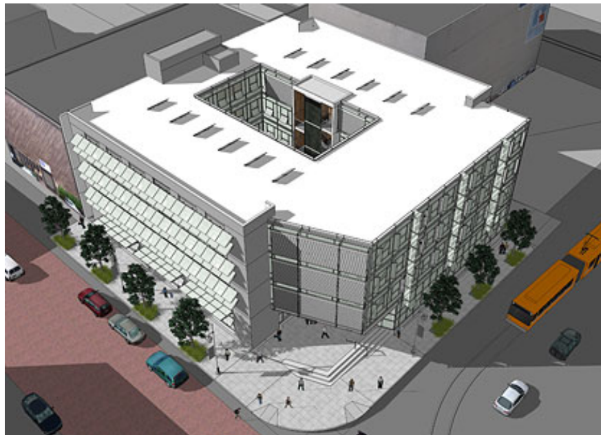
Figure 5.1 Weber + Thompson Building, Seattle, Washington, 2007. A central courtyard stimulates the “stack effect” to increase ventilation. (Source:Weber + Thompson Architects) 22
