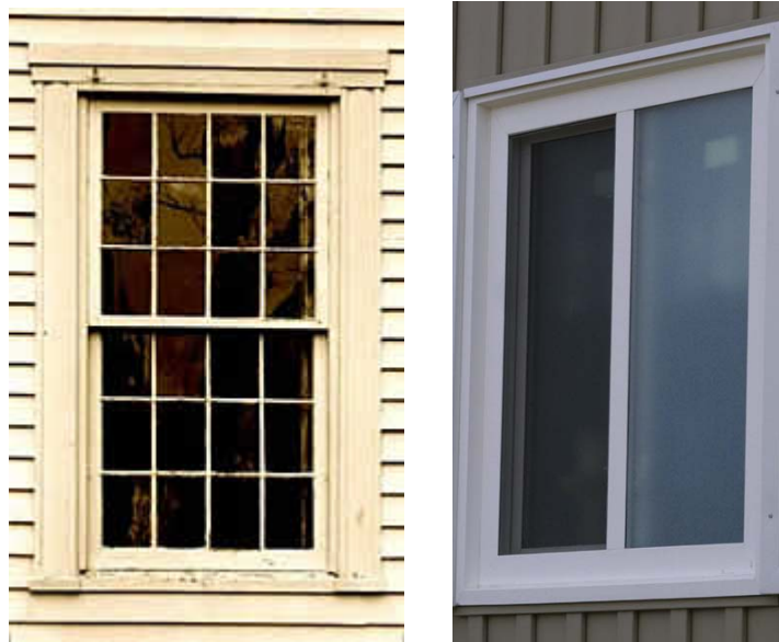
Figure 3.1 The historic window on the left . (Source: John Leeke, National Park Service) has operable sashes that enable building occupants to passively ventilate the building. The modern window on the right (Source: Glengrove Windows) is fixed, meaning it cannot be opened. Building occupants are forced to rely on electricity for ventilation and cooling
