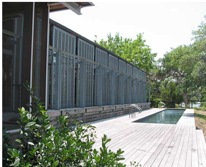
Figure 5.2. External Shading Devices reminiscent of Charleston’s historic shutters (Source: Beth Broome, Architectural Record Magazine)
