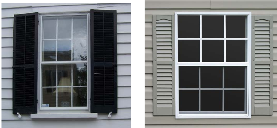
Figure 3.3 The historic window on the left . (Source: Newport Preservation) has operable louvered shutters. The modern shutters on the right (Source: Shawnee Shutters) are bolted to the house.
